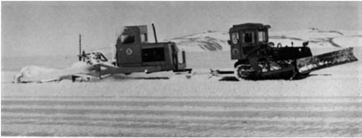
Figure 56. U.S. Navy (NCEL) pulverizing mixer towed by small bulldozer. This was experimental construction on the Ross Ice Shelf between McMurdo Station and White Island. (Photo by M. Mellor, 1961.)
