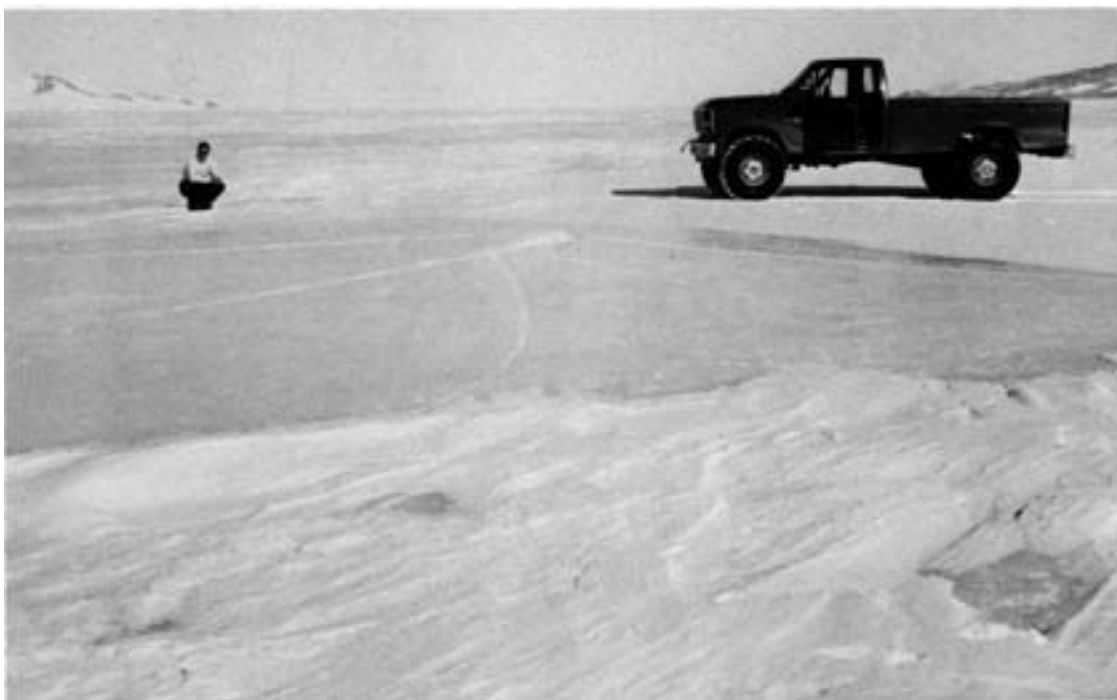
b. Ice blister. When subsurface melt cavities re-freeze in the autumn, the water expands and pushes up the surface to form an ice blister, which has radial cracks. An area that has significant numbers of ice blisters is unsuitable for runway construction. Even if there is enough snow cover to form a protective reflection layer, it is difficult to plane the blistered surface perfectly flat. (Photo by M. Mellor, 3 December 1989.)
