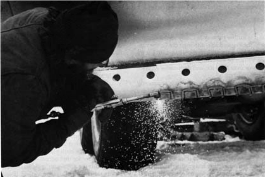
a. Teeth are cut into the replaceable edge with a torch.
