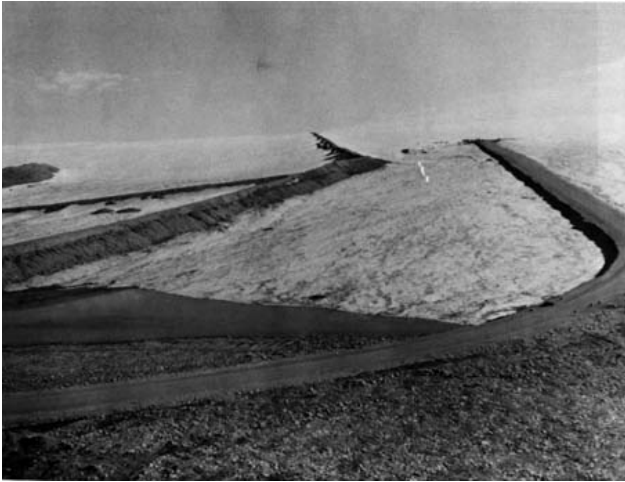
Figure 80. Gravel roads built on glacier ice in Greenland. The road to the right is newly built. The one to the left has deteriorated due to ablation of the adjacent bare ice. The mean annual temperature here is -11^{\circ}\text{C} , and the thaw index is 270–360 ^{\circ}\text{C} degree-days, causing the ice to suffer net ablation of about 8 ft/yr (2.4 m/yr). The optimum depth of gravel fill was 3 ft (0.9 m), with 2.5 ft (0.76 m) of coarse material and 0.5 ft (0.15 m) of fine gravel capping. (U.S. Army photo by SP5 W.J. Davis, 1961.)
