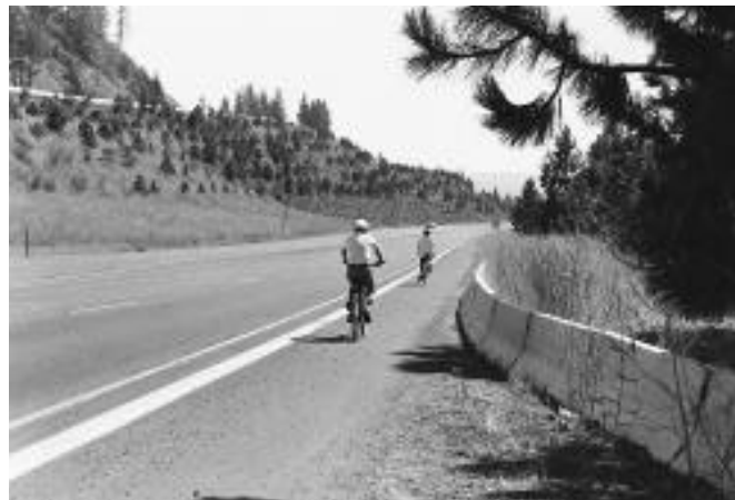
A shoulder bikeway is one of three types of standard bicycle facilities.
