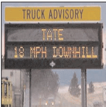
Downhill speed information system displays safe speeds at Emigrant Pass 76
