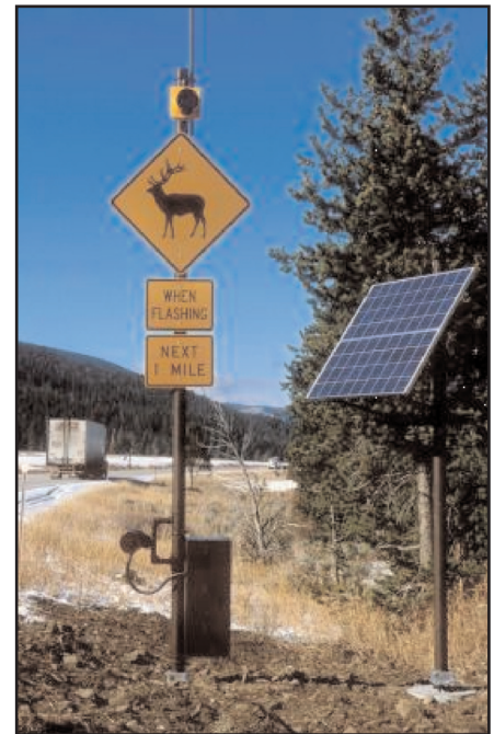
Animal detection system on U.S. Highway 191 in Yellowstone National Park 102
