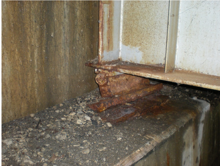
Figure 3. Debris accumulated in the beam seat area as a result of a failed joint/seal in the deck above the bearing
