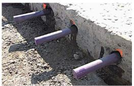
Dowel bars, studied in this project, are set in one slab of pavement waiting for the next one to be poured.
