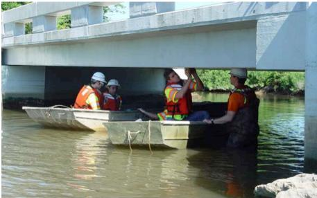
Figure 13. Instrumenting Bridge Underside
