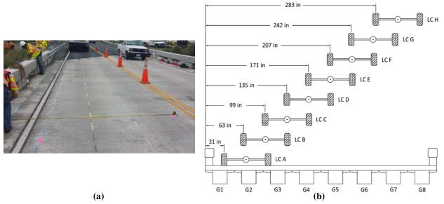
Figure 15. Wheel Path (a) Markings and (b) Configuration
