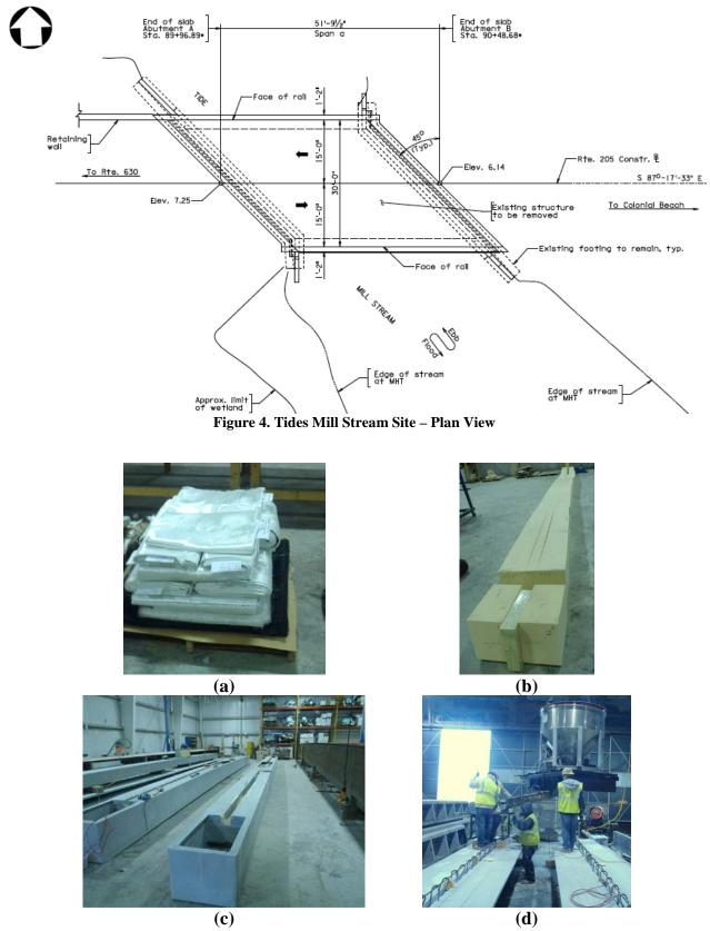
Figure 5. HCB Fabrication Process: (a) Glass Fiber Fabric, (b) Foam Inserts, (c) Completed HCB Box, and (d) Placement of SCC Within HCB Arch
