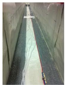
Figure 9. Internal VWG Placement at Tension Level
