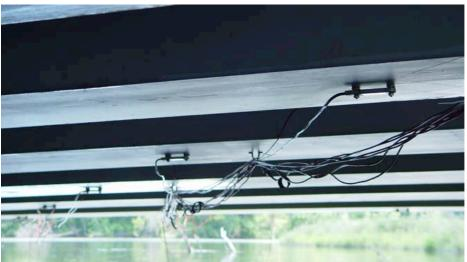
Figure 14. Bottom Flange External Strain Gauge Placement
