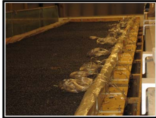
d) Manometer Tubes Feeding to Manometer Board
