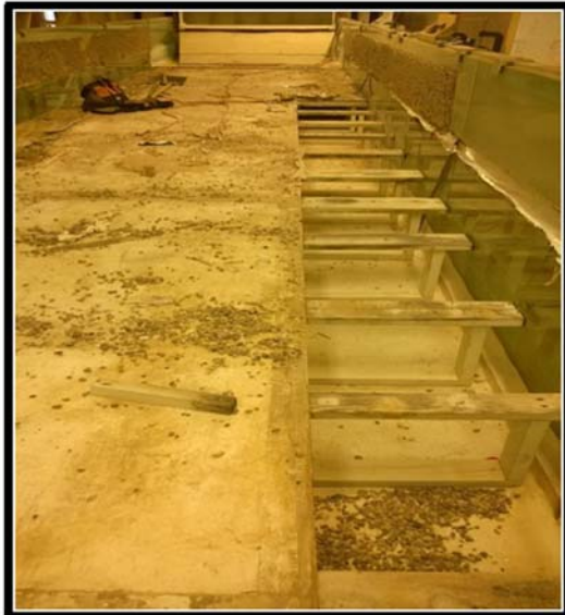
c) Partial Demolition of Prior Installation
