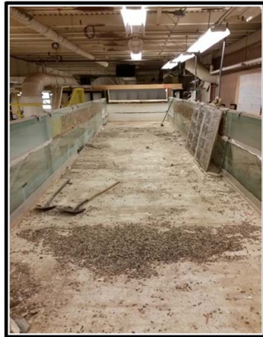
d) Complete Demolition-Before Clean-Up
