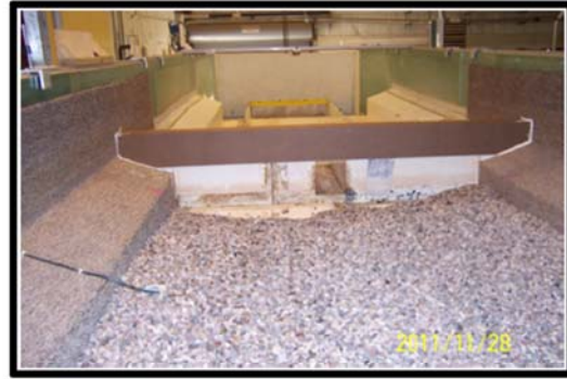
b) Prior Installation-Looking Downstream (Barnes, 2013)
