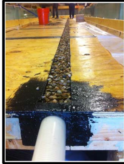
b) Underdrain Slot Backfilled with Aggregate
