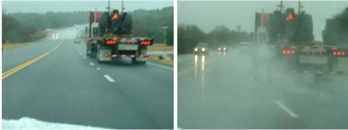
Figure 4. PFC pavement reduces splash and improve visibility in the evening (Barrett and Stanard (2008))
