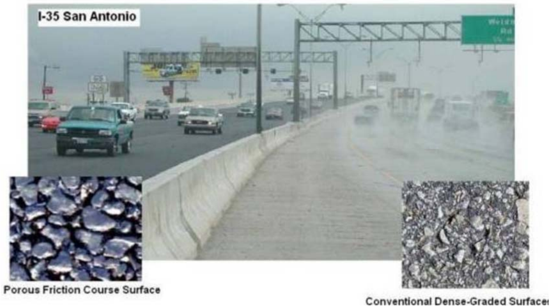
Figure 5. PFCs in urban areas to reduce splash and spray (San Antonio IH 35) (Arambula (2013))
