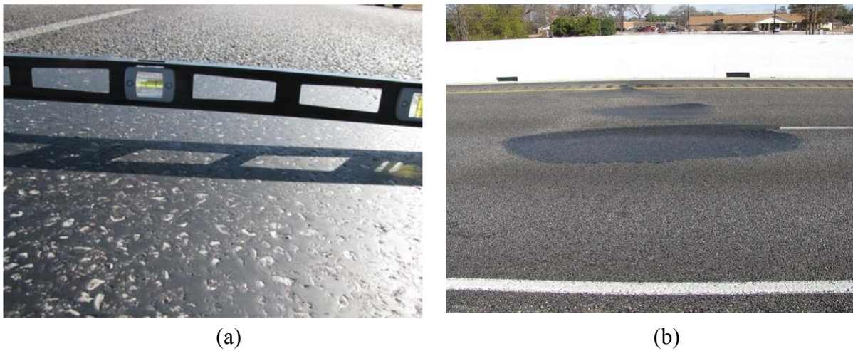
Figure 9. Most frequent failure mode of PFC pavement in Texas (modified from Arambula et al. 2013): (a) raveling and rutting; and (b) rutting and bleeding.
