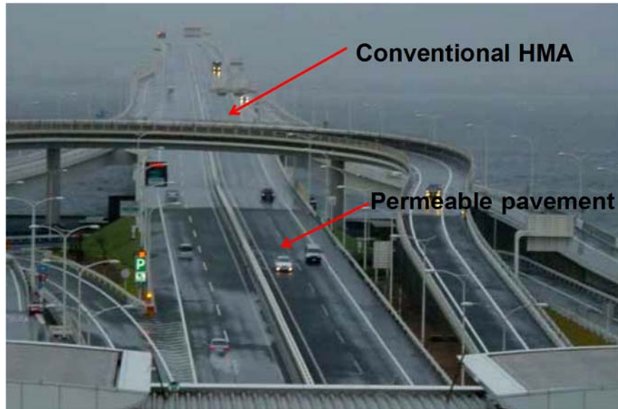
Figure 3. PFC pavement reduce water standing on pavement during a rainstorm (modified from Poulikakos et al. (2003)).
