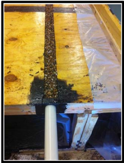
c) Underdrain Slot Backfilled with Aggregate
