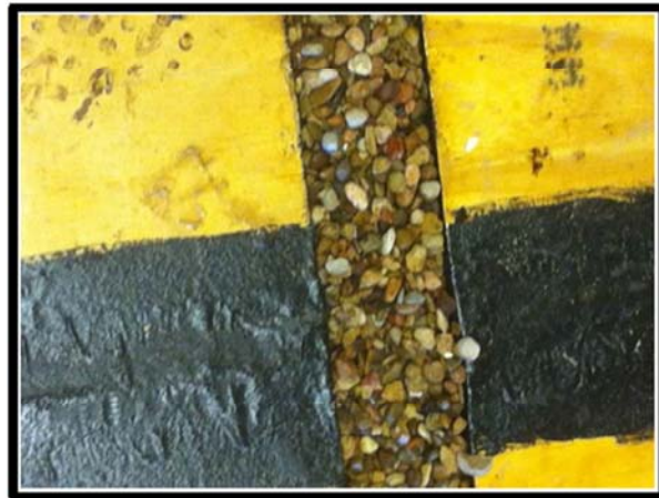
d) Underdrain Slot Backfilled with Aggregate
