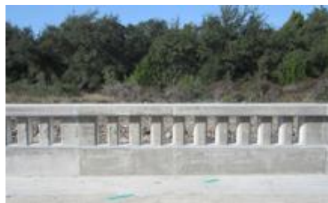
Figure 1. Aesthetic barrier tested at TTI
