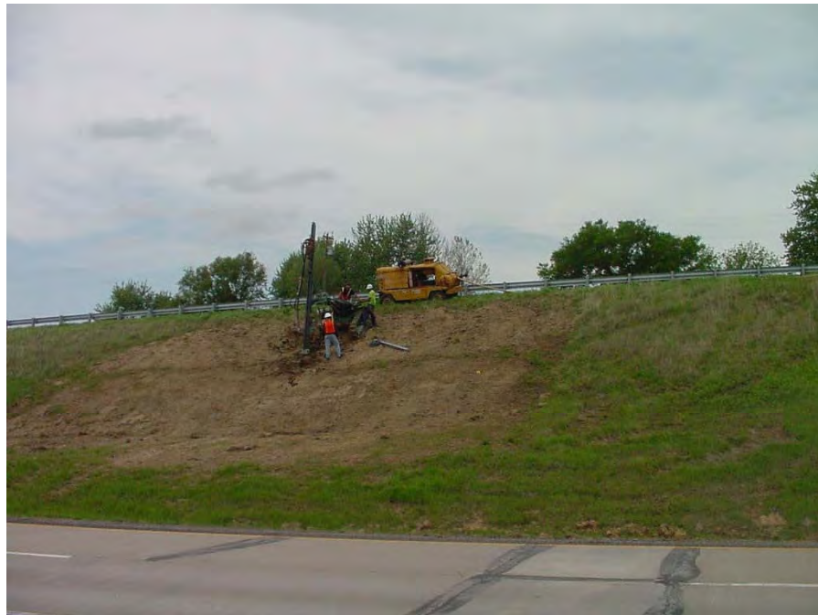
Figure 8.7 Photograph of US36-Stewartsville control slide during installation of instrumented reinforcing members.
