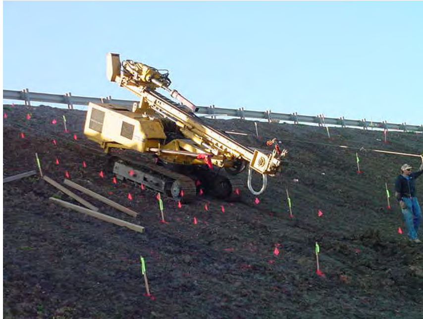
(a) Davey-Kent DK100B track-mounted hydraulic rig
