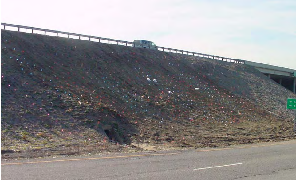
Figure 10.8 Photograph of I435-Wornall Road site following installation.
