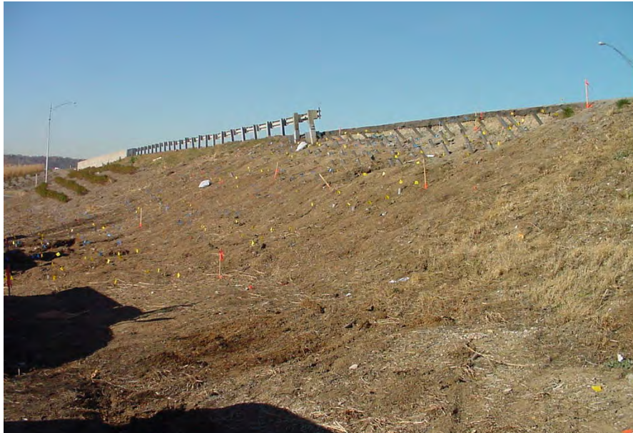
Figure 10.11 Photograph of I435-Holmes Road site just after installation.
