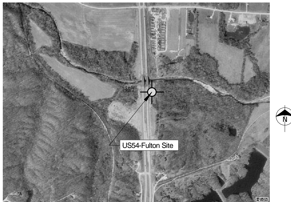
Figure 9.1 Air photo of area surrounding US54-Fulton site taken April 3, 1995 showing location of slope selected for stabilization (from USGS).
