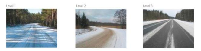
Figure A.5.3 LOS 1-3 in Estonia (LOS 4 is bare pavement; adopted from PIARC 2015)
