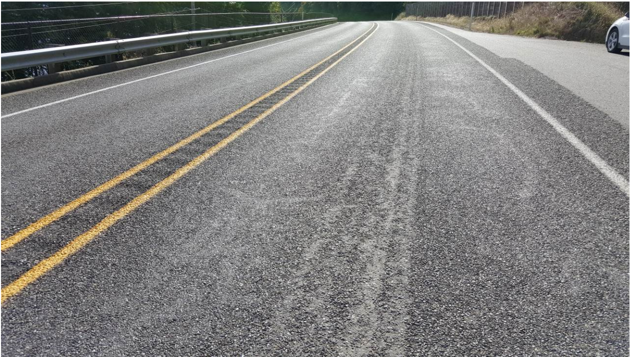
Figure 51. OR1a, SR101, three years after installation. Very slight flushing and shadowing of the sealed cracks.
