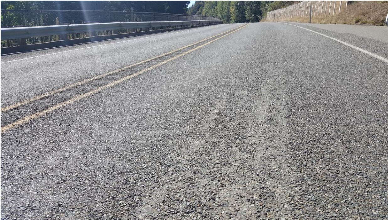
Figure 52. OR1a, SR101, four years after installation. Slight amount of rutting beginning to appear. Flushing does not seem to be a big issue.
