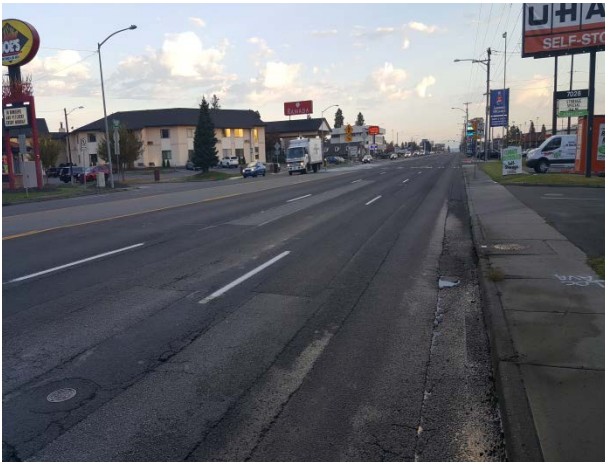
Figure 119. ER2a, SR2, Reactive, at 2016 inspection. Dig outs, crack sealing and patching were necessary to preserve the roadway.
