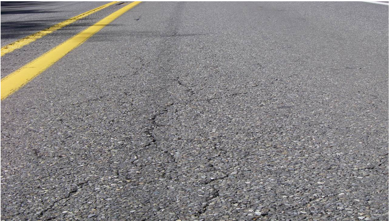
Figure 24. OR1b, SR101, prior to treatment. Alligator cracking was noted over the entire lane, but especially severe in the wheel paths.
