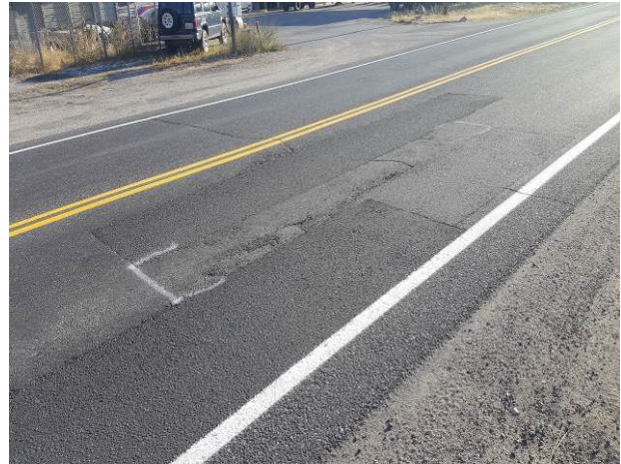
Figure 54. ER3, SR291, Emerging, age 50 months. Additional dig outs added in 2015. Transverse reflection crack noted at 10 months after treatment. More dig outs are scheduled for installation in 2017.
