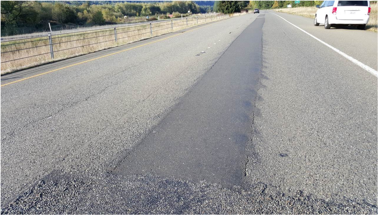
Figure 77. OR2, SR8 three years after installation. Slight rutting in the patch.
