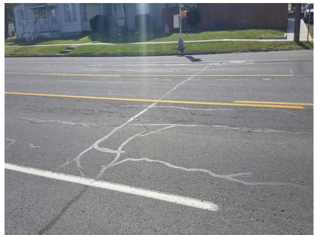
Figure 56. ER5, SR2, Reactive, age 38 months. Transverse reflection crack noted at the age of 10 months after treatment.
