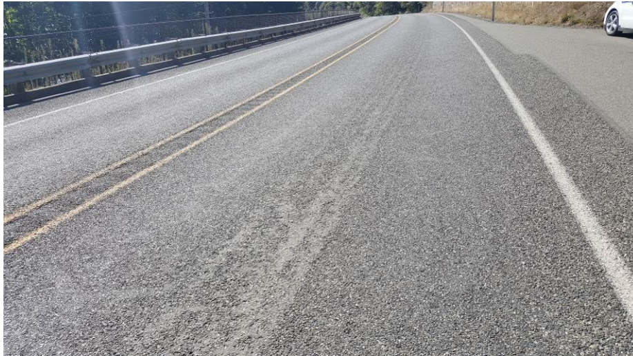
Figure 135. OR1a crack sealing plus chip sealing on SR 101. (September 2016)
