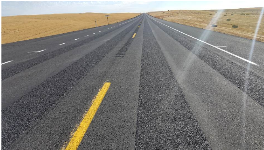
Figure 133. ER10, wheel path chip seal rut filling on US 2. (September 2016)
