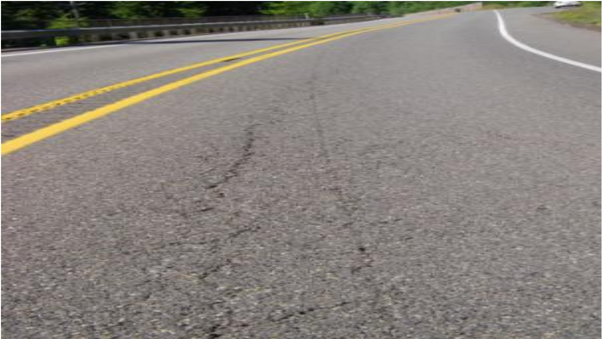
Figure 48. OR1a, SR101, prior to treatment. Alligator and longitudinal cracking noted.
