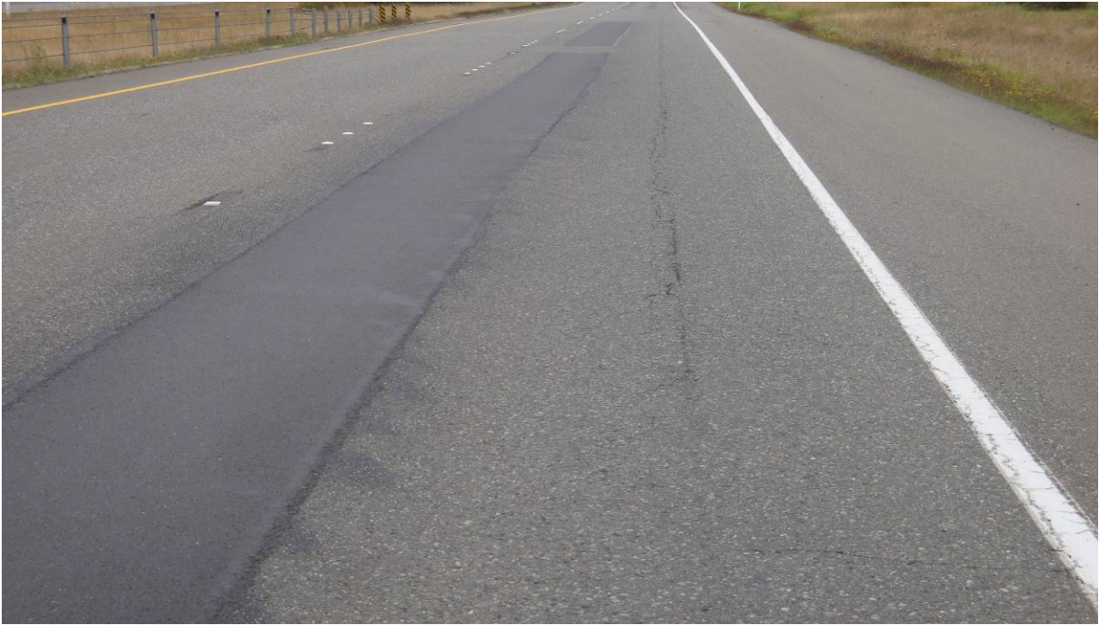
Figure 75. OR2, SR8, one year after installation. Dig out patch looks excellent.
