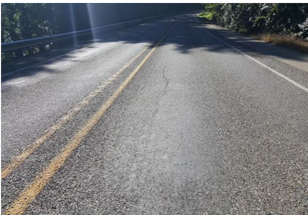
Figure 20. OR1b, SR101, Reactive, age 50 months. Longitudinal cracking noted at 21 months. Slight flushing in the wheel paths.
