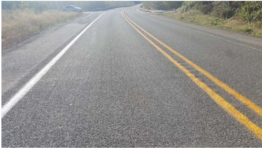
Figure 134. OR3b full lane chip seal on SR 101. (September 2016)
