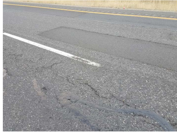
Figure 118. ER1a, SR2, Reactive, at 2016 inspection. Dig outs, crack sealing and patching were necessary to preserve the roadway.
