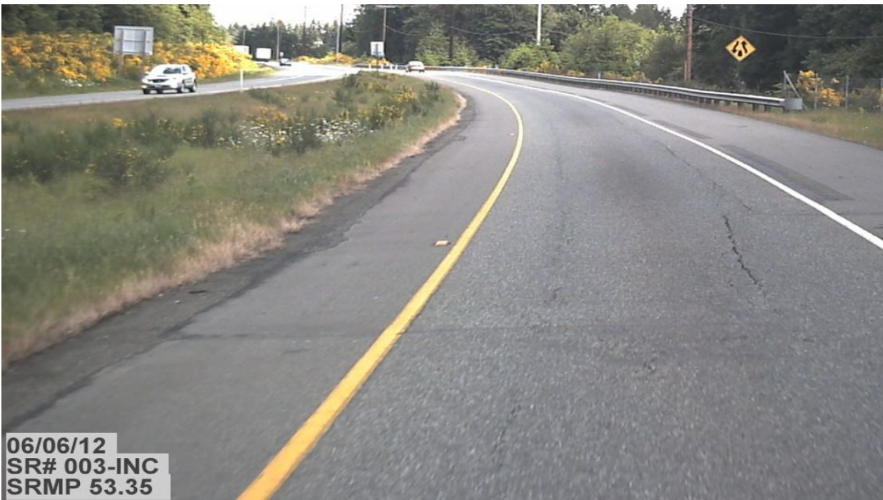
Figure 88. OR4, SR3, prior to treatment. Longitudinal, transverse and alligator cracking.
