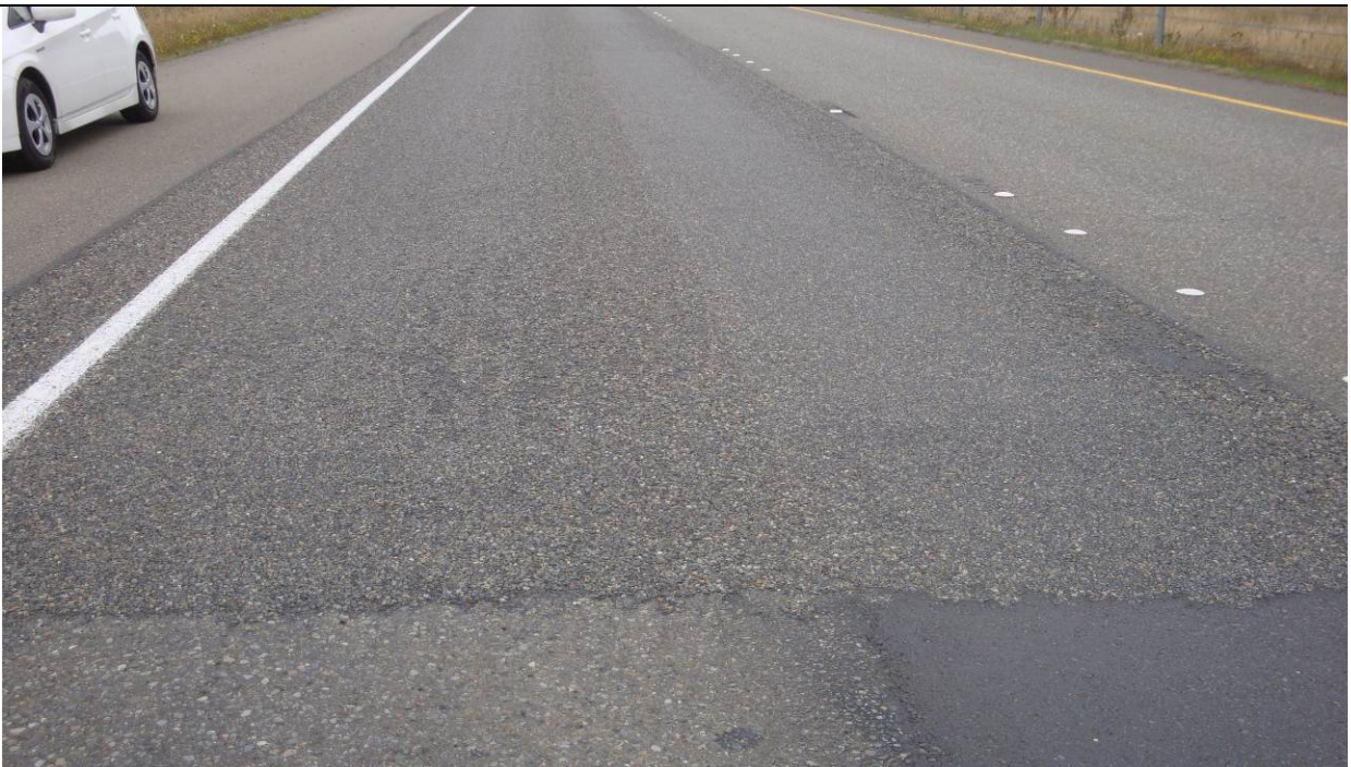
Figure 100. OR2a, SR8, one year after installation. Slight flushing in the wheel paths over the dig out patches.
