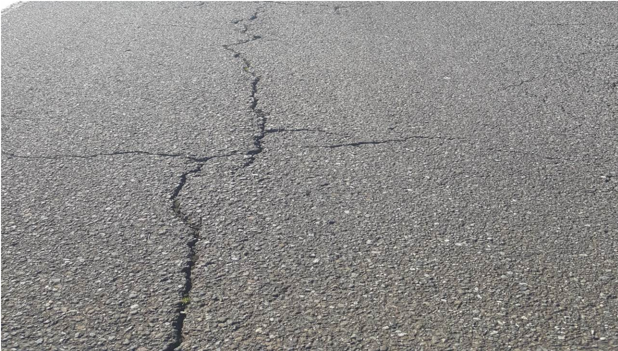
Figure 125. OR3a, SR101, four years after the other sections were treated. Cracks are wide and beginning to spall.
