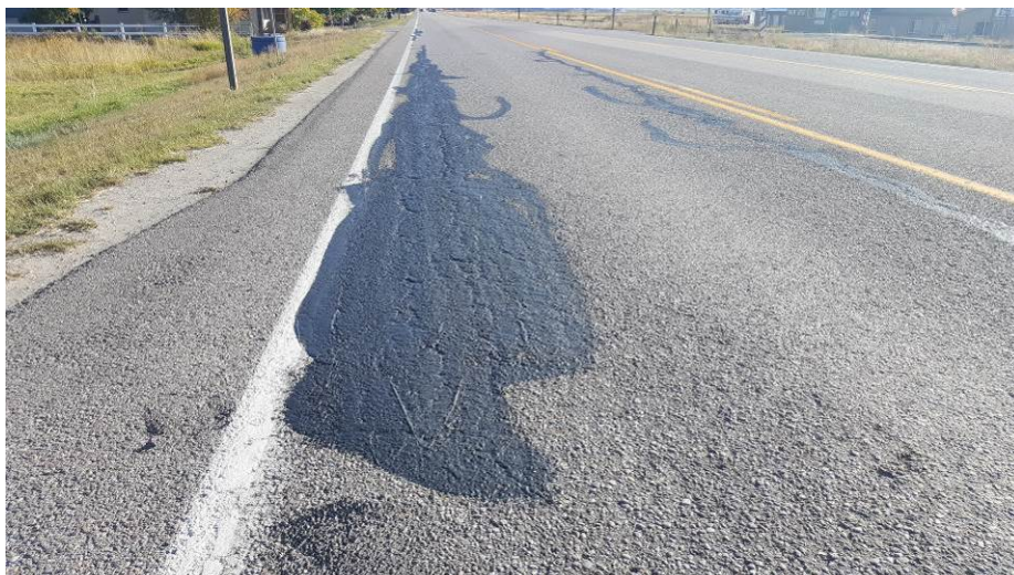
Figure 132. ER41, excessive crack sealant used on alligator cracking on SR 20, ER41. (November 2016)
