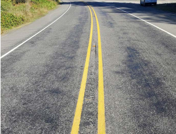
Figure 97. OR14, SR7, Strategic, age 39 months. Dig out patches flushing through the chip seal at 27 months.
