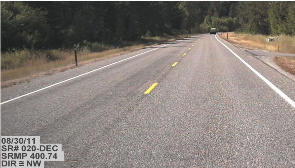
Figure 41. ER7, SR20, prior to installation. Rutting is visible in the wheel paths.
