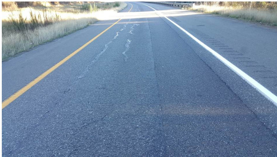
Figure 138. OR4 dig outs plus crack sealing on SR 3. (September 2016)
