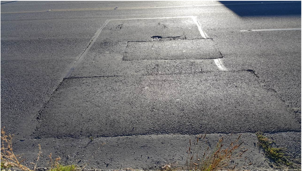
Figure 83. OR5, SR7, three years after installation. No change in the dig out patches.
