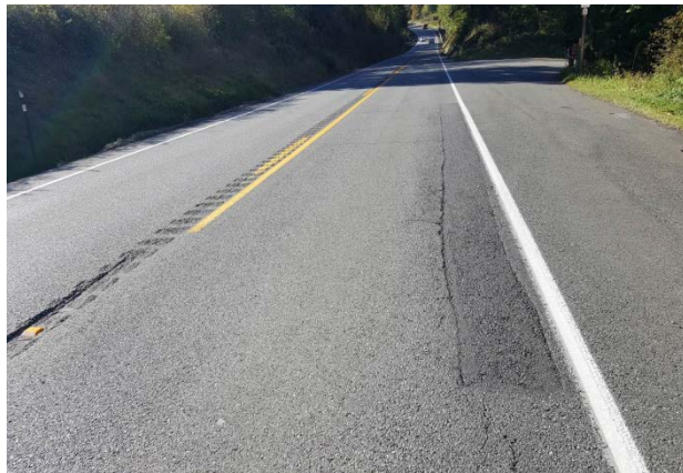
Figure 60. OR11, SR20, Strategic, age 38 months. Raveling of patch edges noted at 25 months.
