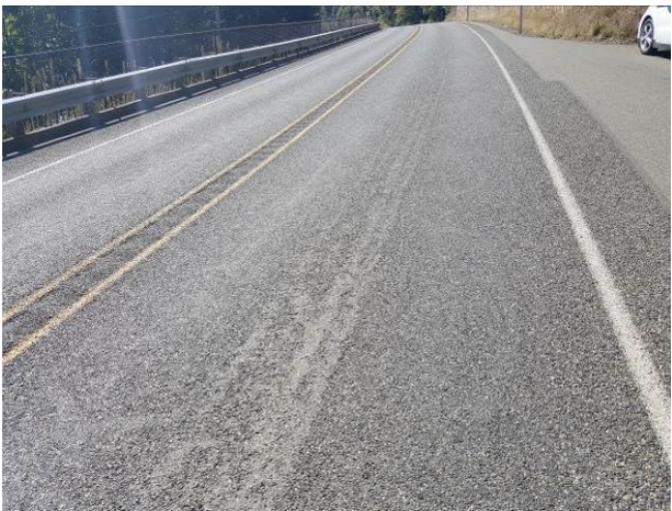
Figure 46. OR1a, SR101, Reactive, age 50 months. Underlying crack sealant can be seen as shadowing.
