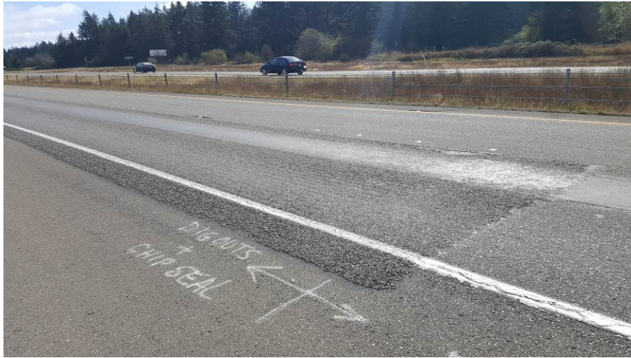
Figure 139. OR2a dig outs plus chip seal SR 8. (September 2016)
