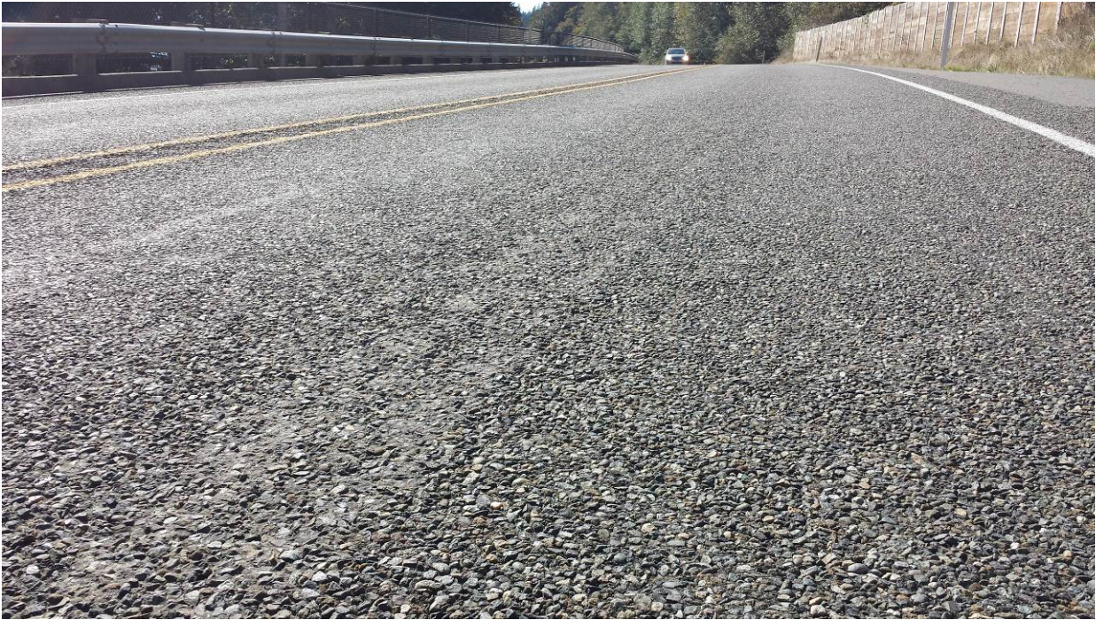
Figure 50. OR1a, SR101, two years after installation. Shadowing of the sealed cracks visible.
