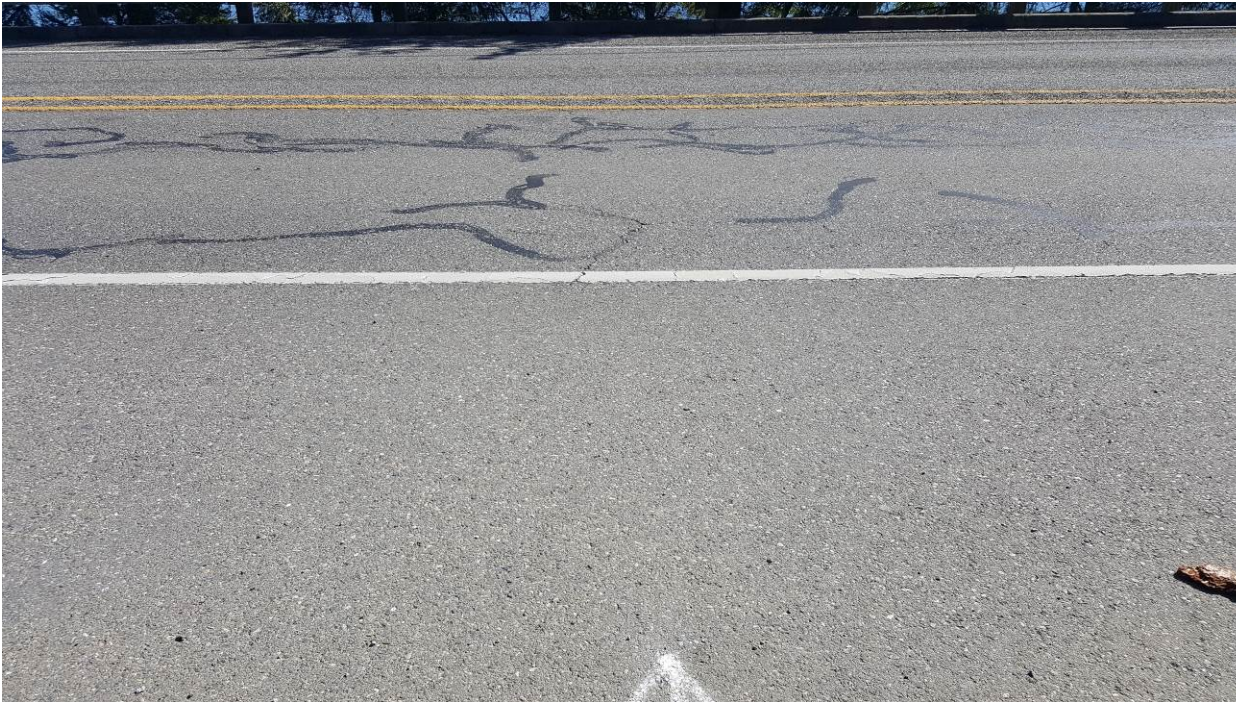
Figure 19. OR1, SR101, four years after installation. There has not been much change in the condition of the crack sealant since year one.
