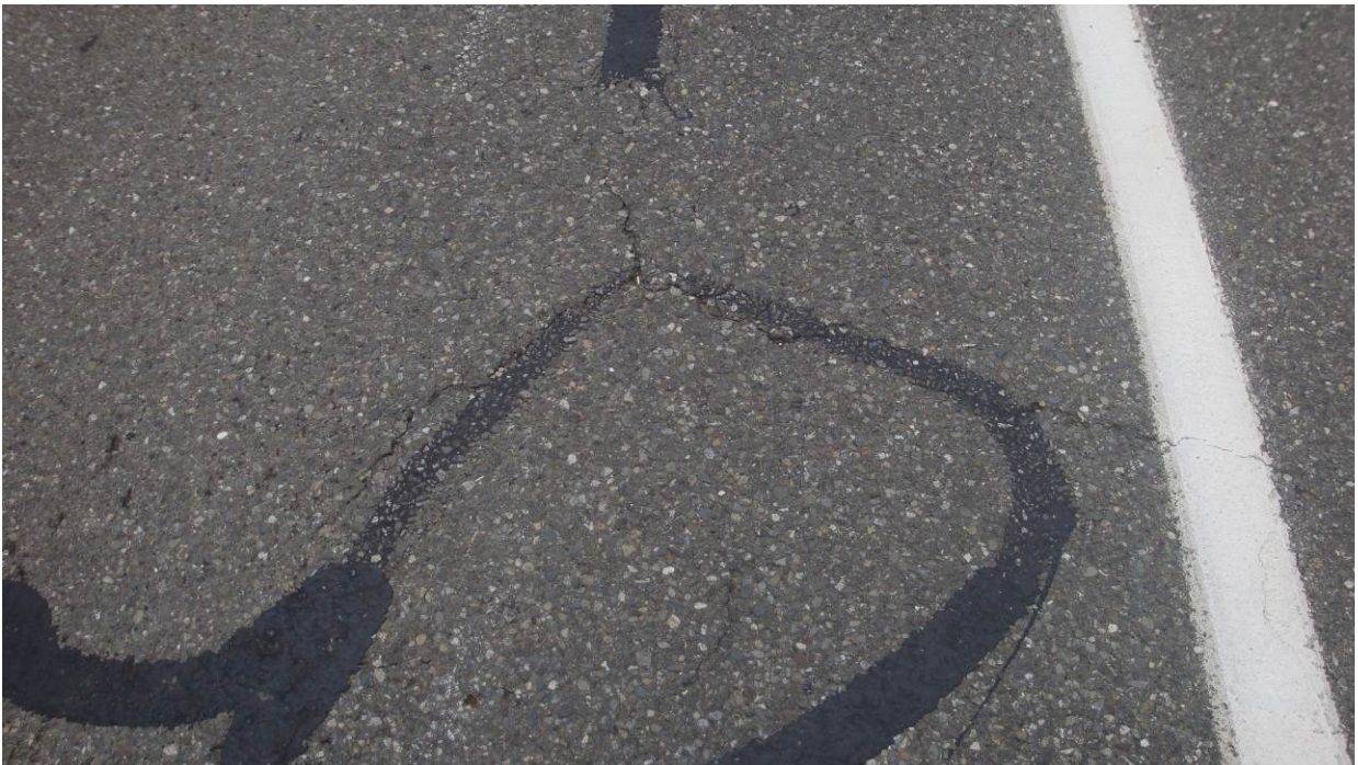
Figure 16. OR1, SR101, one year after installation. Slight wear of sealant over banding.
