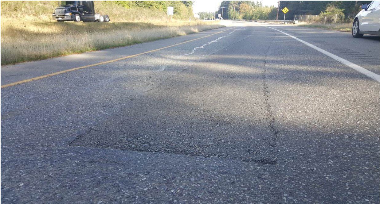
Figure 91. OR4, SR3, two years after installation. No change in dig out patch or crack sealing.
