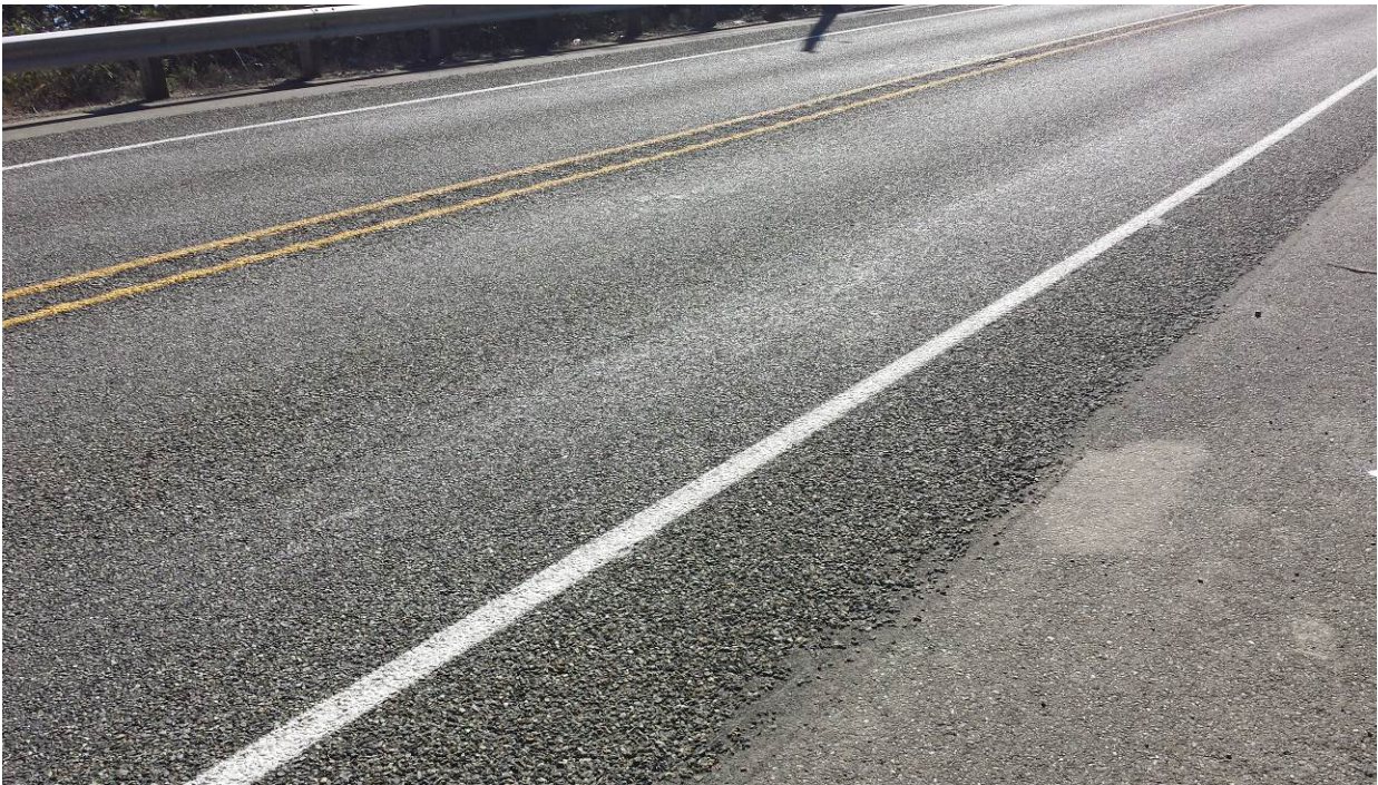
Figure 26. OR1b, SR101, two years after installation. Longitudinal crack appears to have “healed”. There is slight flushing in the wheel paths.
