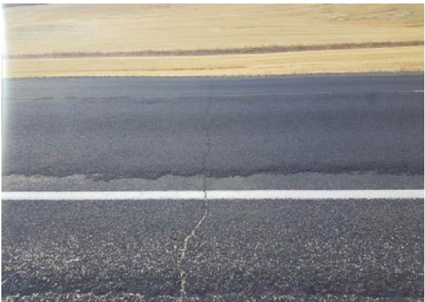
Figure 106. ER20, SR272, Strategic, age 12 months. Transverse crack reflecting through the patch.
