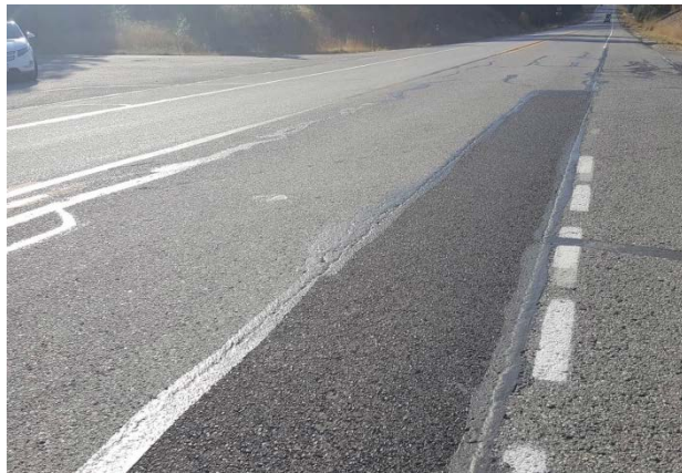
Figure 60. OR11, SR20, Strategic, age 38 months. Raveling of patch edges noted at 25 months.
