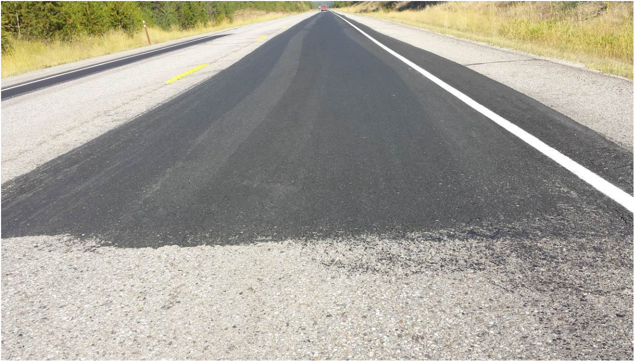
Figure 114. ER9a, SR395, a few months after installation. Blade patch looks excellent.
