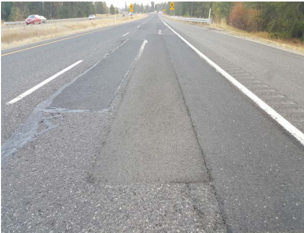
Figure 84. ER1, SR2, Reactive, age 50 months. Additional dig outs and crack sealing done in 2015.
