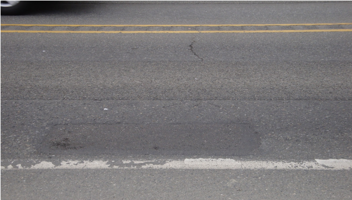
Figure 35. OR12, SR20, three years after installation. Some loss of aggregate but no reflection cracking.
