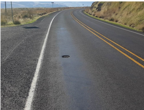
Figure 93. OR2a, SR8, Strategic, age 50 months. Flushing over the dig out patches.
