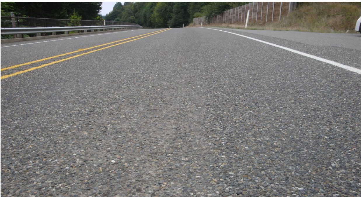
Figure 49. OR1a, SR101, one year after installation. Chip seal looks excellent.
