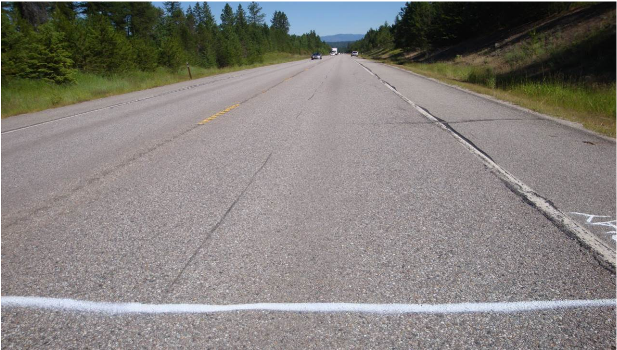
Figure 113. ER9a, SR395, prior to treatment. Longitudinal, transverse and alligator cracking.
