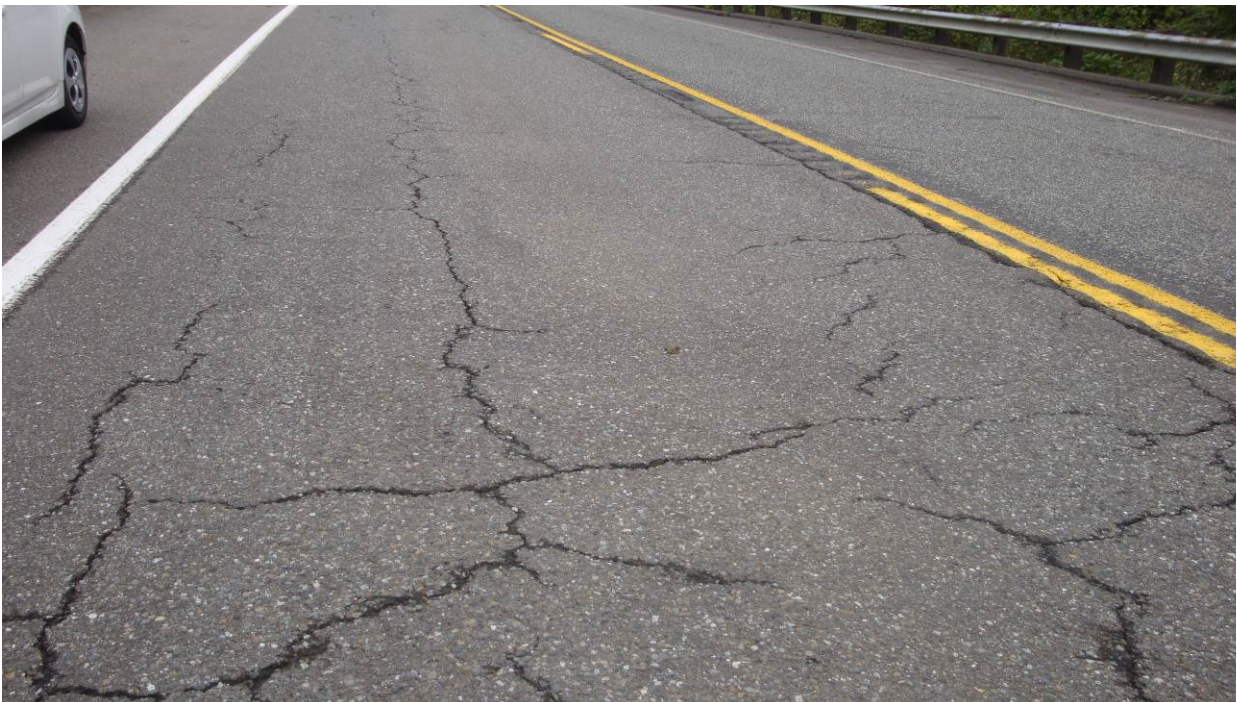
Figure 122. OR3a, SR101, one year after the other sections were treated. Cracking looks severe due to moisture in the cracks.
