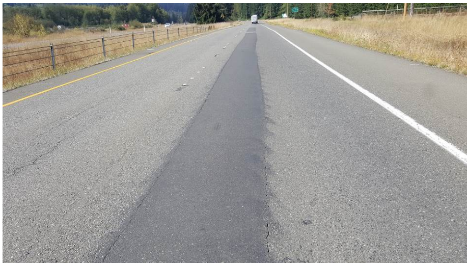
Figure 137. OR2 dig outs on SR 8. (September 2016)
