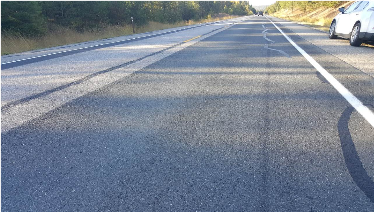
Figure 116. ER9a, SR395, two years after installation. Longitudinal reflection cracking has been sealed. Note slight flushing in the left wheel path.
