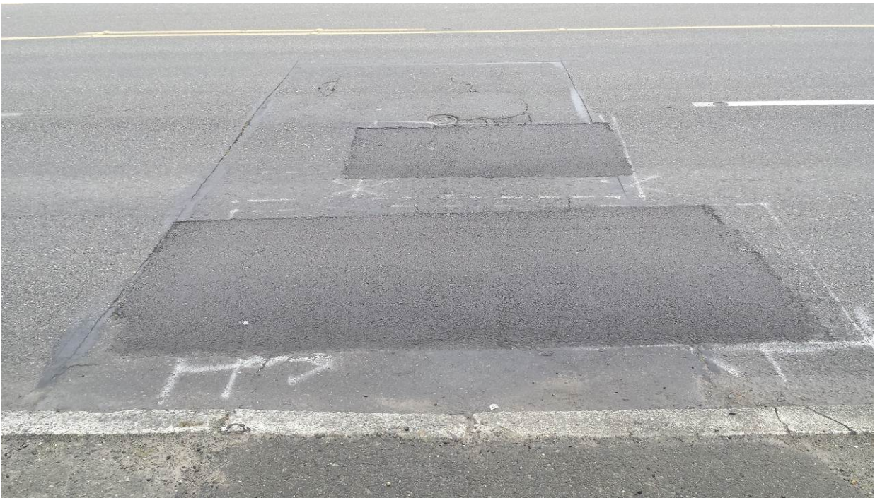
Figure 81. OR5, SR7, one year after installation. No change in the dig out patches.
