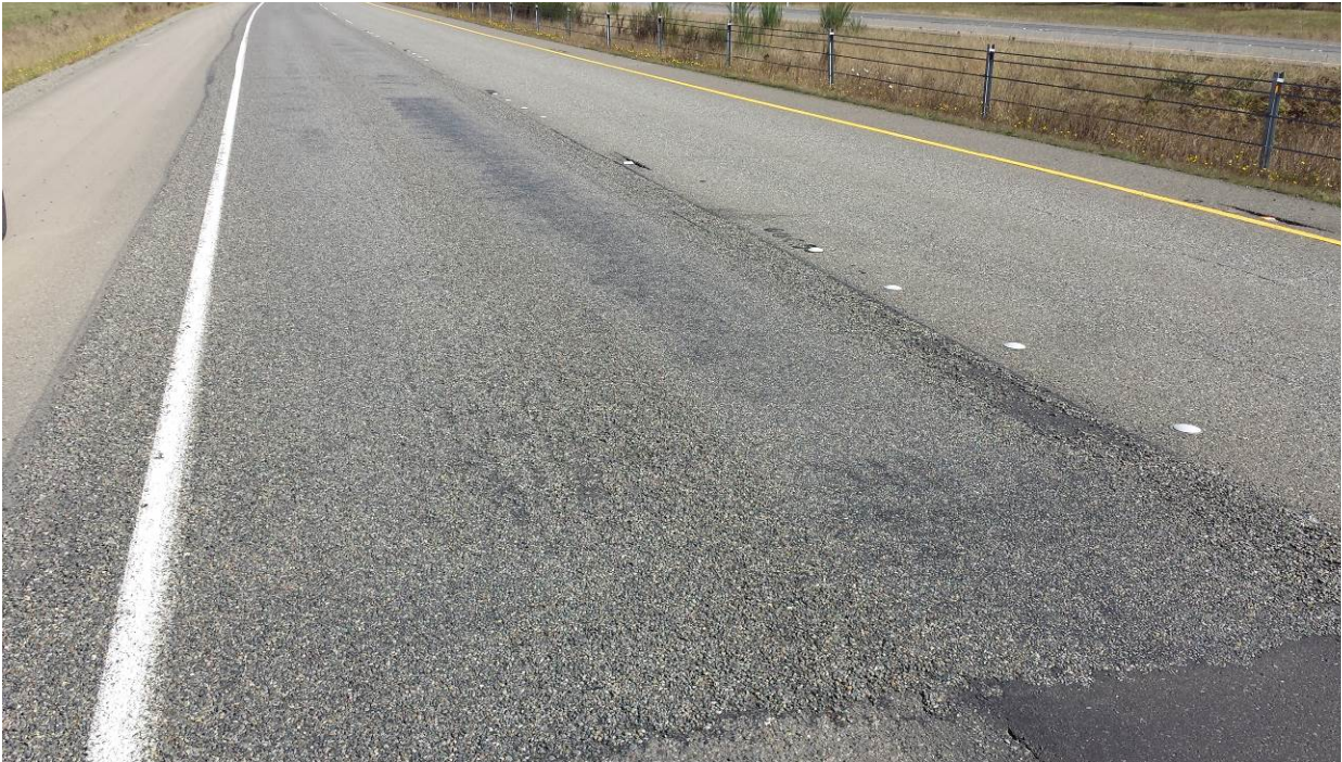
Figure 101. OR2a, SR8, two years after installation. Increased flushing in the wheel paths over the dig out patches.
