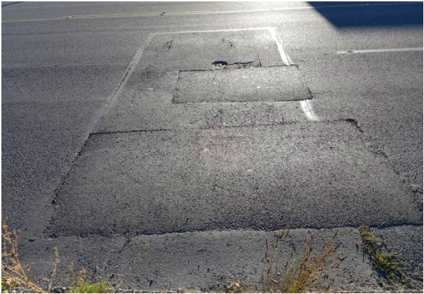
Figure 57. OR5, SR7, Strategic, age 39 months. No problems with patches, pavement continues to deteriorate adjacent to the patches.
