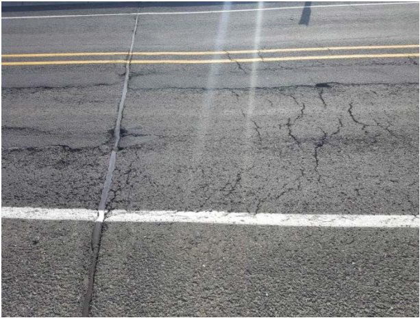
Figure 104. ER8, SR195, Strategic, are 27 months. Blade patch used to fill wheel path ruts.
