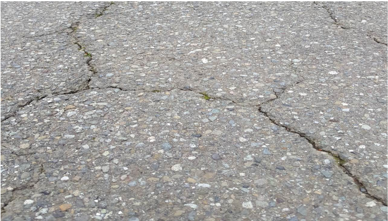
Figure 124. OR3a, SR101, three years after the other section were treated. Cracks are wide but not spalling.
