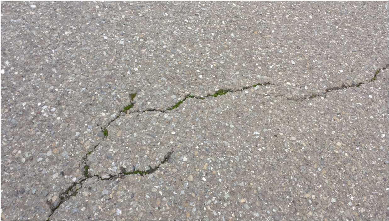
Figure 123. OR3a, SR101, two years after the other sections were treated. Vegetation growing in the wider cracks.
