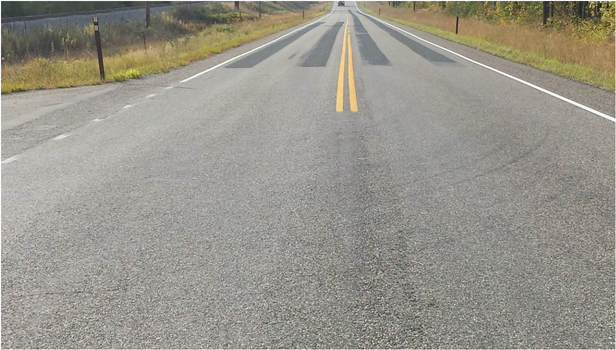
Figure 44. ER7, SR20, two years after installation. No change in chip seals.
