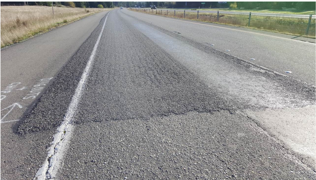
Figure 102. OR2a, SR8, three years after installation. Increased flushing in the left wheel path throughout the length of the chip seal.
