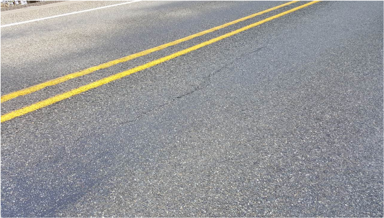
Figure 27. OR1b, SR101, three years after installation. Longitudinal crack is getting longer and wider. The flushing in the wheel paths is about the same.
