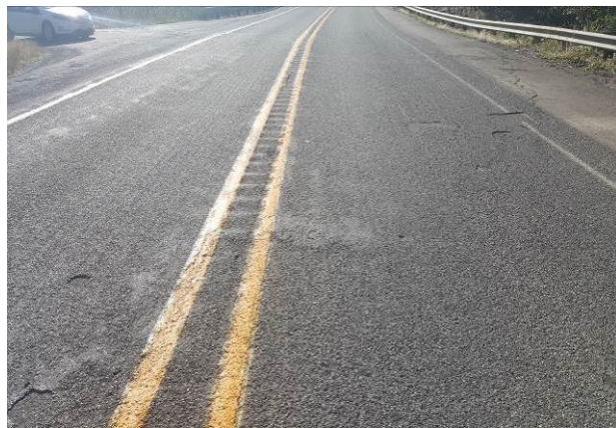
Figure 21. OR3b, SR101, Reactive, age 50 months. Delamination and spalling noted.
