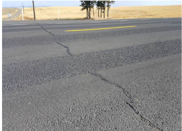
Figure 37. ER10, SR2, Strategic, age 24 months. Cracking noted at 12 months.
