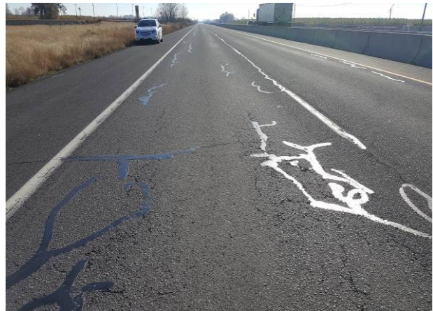
Figure 8. SC1, SR97, Strategic, age 14 months. No spalling or potholes.
