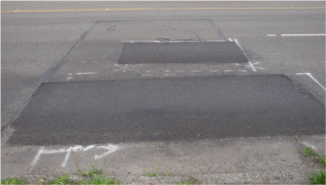
Figure 80. OR5, SR7, immediately after installation. Dig out patches look good. They appear to be related to utility cuts in original pavement.
