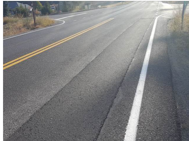
Figure 120. ER3a, SR291, Emerging, at 2016 inspection. Dig outs, crack sealing and patching were necessary to preserve the roadway.
