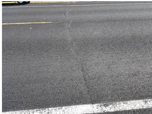
Figure 47. NC1, SR155, Strategic, age 26 months. Transverse crack locations are visible.
