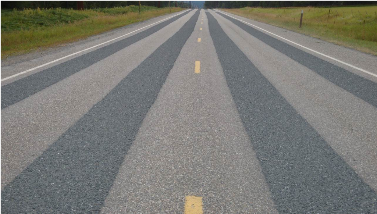
Figure 42. ER7, SR20, a few months after installation. Excellent looking wheel path chip seal rut filling.
