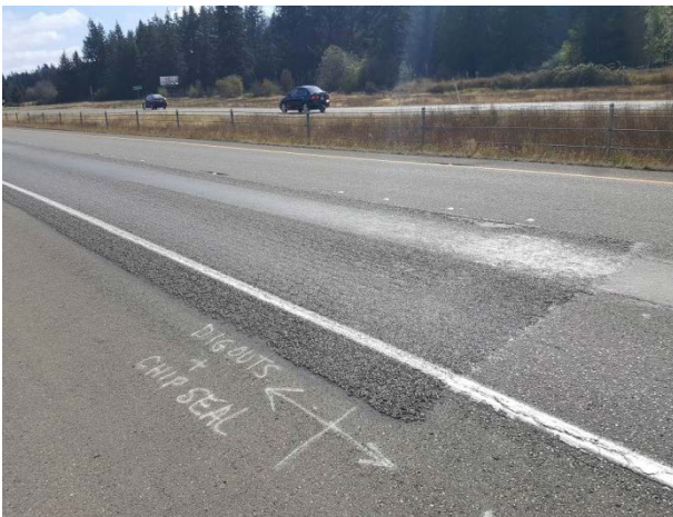
Figure 93. OR2a, SR8, Strategic, age 50 months. Flushing over the dig out patches.
