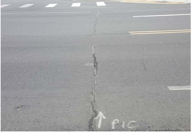
Figure 63. ER11, SR270, Emerging, age 25 months. Transverse crack at 12 months after installation.
