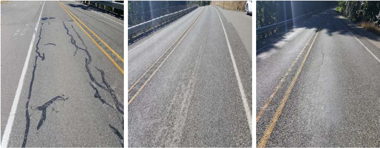
Figure 129. OR1, OR1a and OR1b on SR 101. OR1 has crack sealing, OR1a has crack sealing and chip sealing, and OR1b has a chip seal with no crack sealing.
