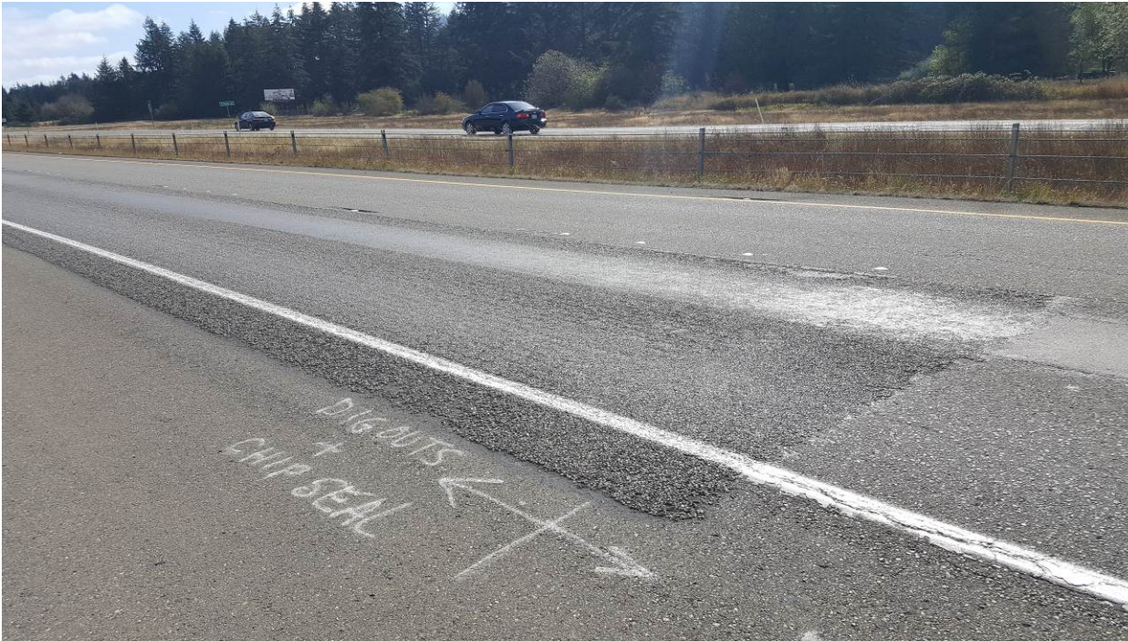
Figure 103. OR2a, SR8, four years after installation. Flushing has remained about the same as in 2015.
