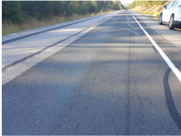
Figure 105. ER9a, SR395, Strategic, age 25 months. Transverse and longitudinal cracking reflecting through the patch at 13 months. It is possible that this could have been a paver and not a blade patch.
