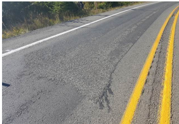
Figure 23. OR22, SR101, Strategic, age 14 months. Loss of aggregate at bottom of superelevation.
