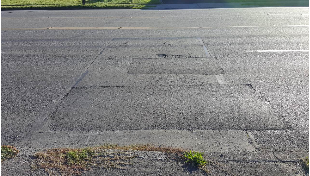
Figure 82. OR5, SR7, two years after installation. No change in the dig out patches.
