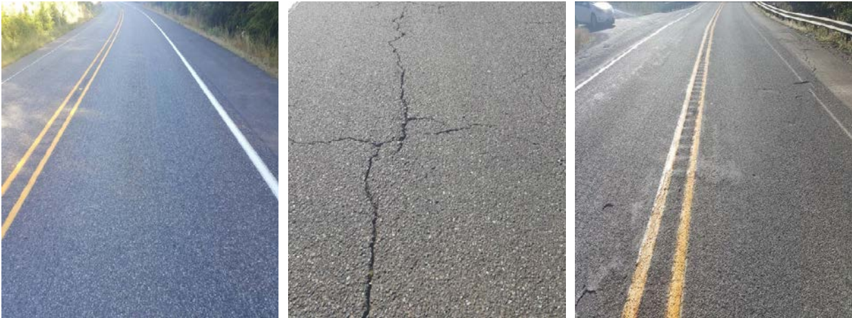
Figure 131. OR3, OR3a and OR3b on SR101. OR3 received dig outs and a chip seal, OR3a is a control section with no treatment and OR3b received a chip seal with no dig outs.
