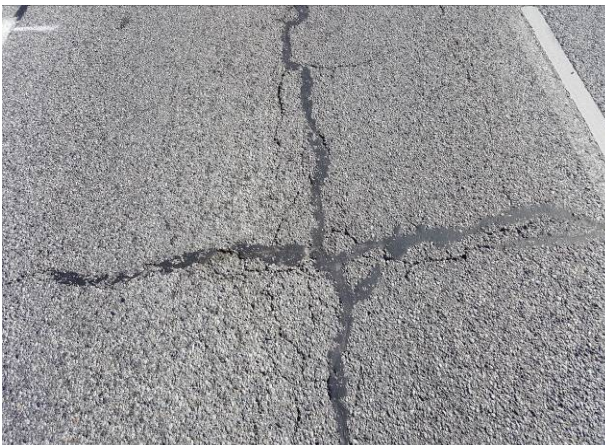
Figure 7. NC2, SR2, Strategic, age 26 months. No spalling or potholes.
