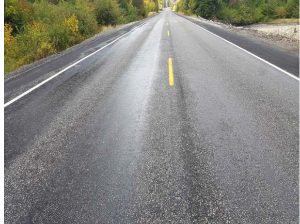
Figure 98. NC3, SR207, Strategic, age 26 months. Dig out patches flushing through the chip seal after 12 months.
