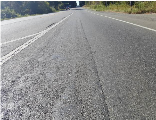
Figure 29. OR12, SR20, Strategic, age 38 months. Longitudinal reflection crack and flushing noted at 10 months.
