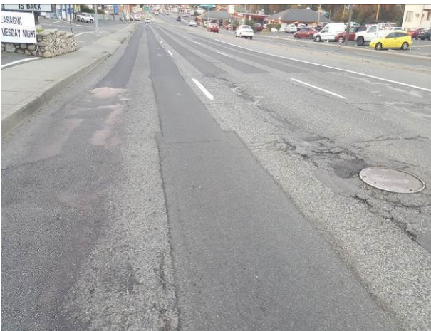
Figure 55. ER2/4, US2, Emerging, age 50 months. Additional dig outs installed in 2013 and 2015.
