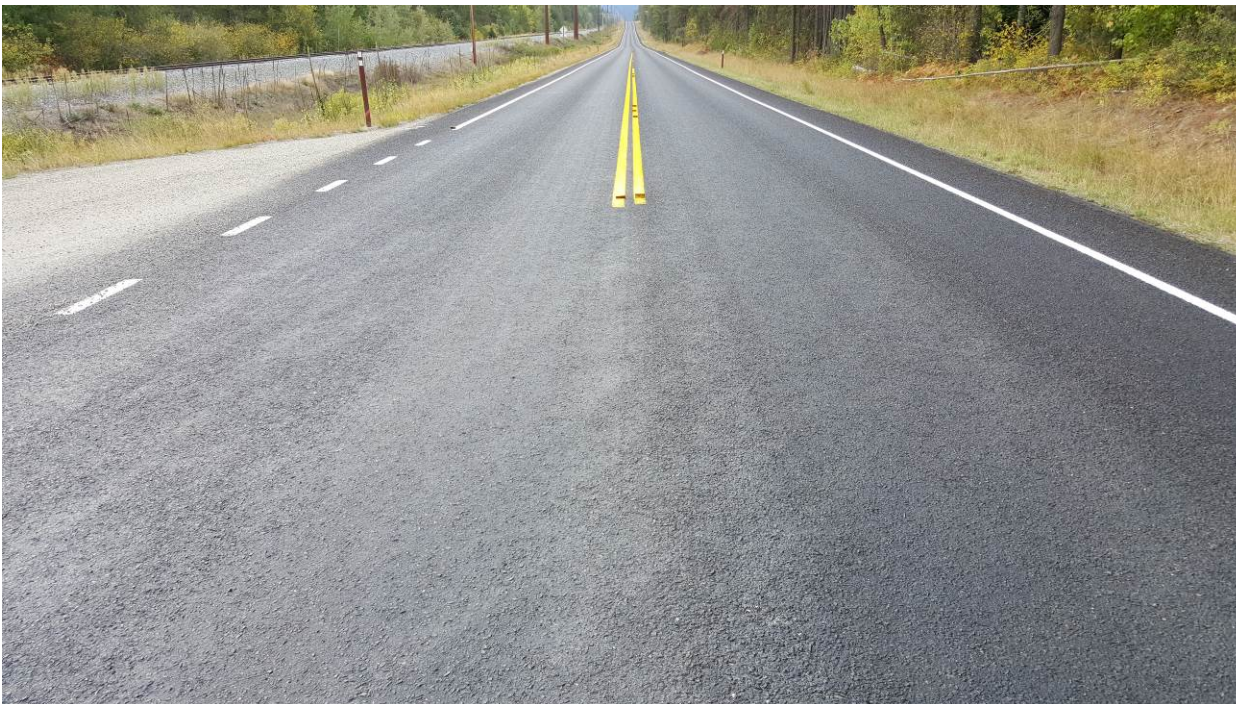
Figure 45. ER7, SR20, three years after installation. Full lane chip seal installed under Contract 8728, US 2 ET AL 2015 Eastern Region Chip Seal.
