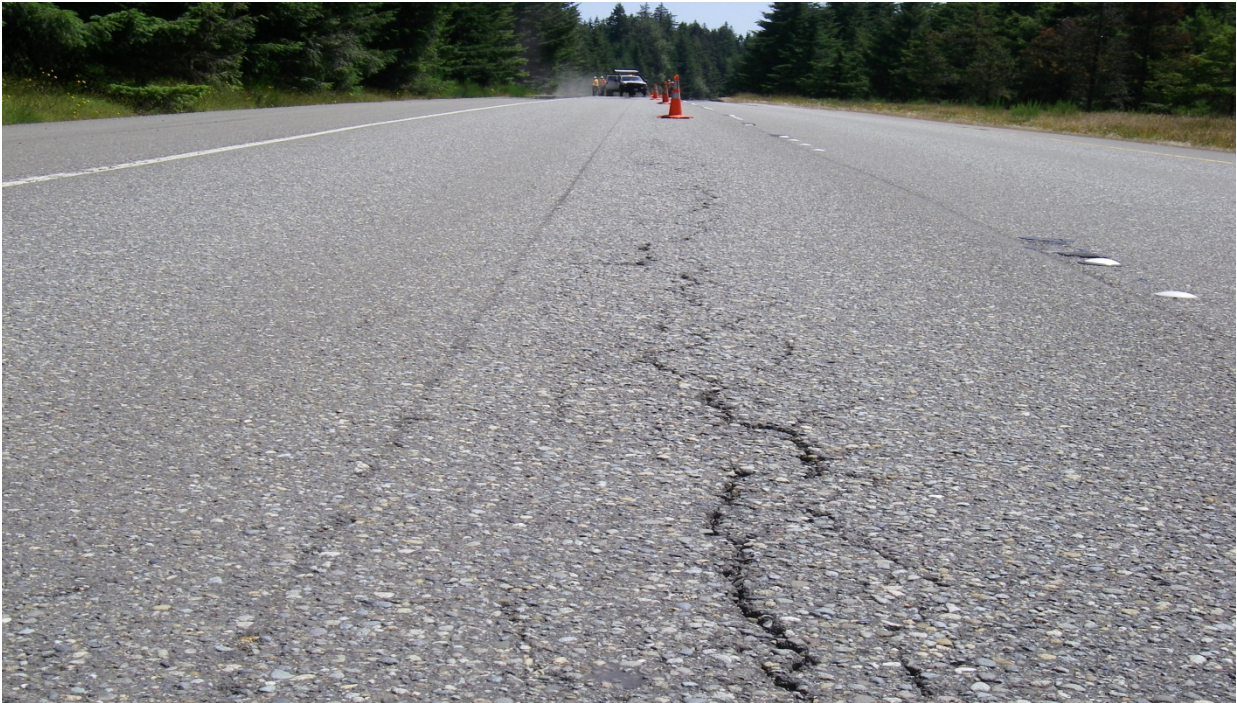
Figure 74. OR2, SR8, prior to treatment. Alligator cracking in the left wheel path. This is not the same location as the following photos which had alligator cracking in both wheel paths.
