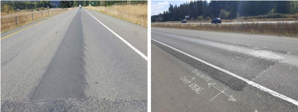
Figure 130. OR2 and OR2a on SR8. OR2 received dig outs and OR2a received dig outs and a chip seal.
