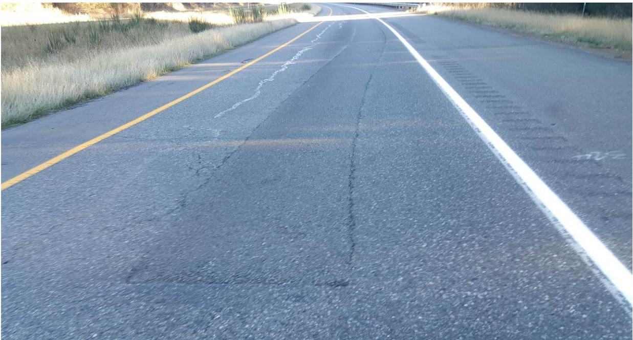
Figure 92. OR4, SR3, three years after installation. No change in dig out patch or crack sealing.
