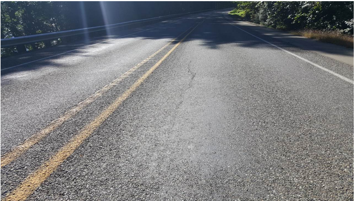
Figure 28. OR1b, SR101, four years after installation. Longitudinal crack condition is about the same, slight rutting and flushing in the wheel paths.
