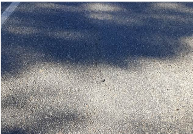
Figure 22. OR16, SR16, Strategic, age 38 months. Longitudinal crack and pumping of fines noted at 14 months.
