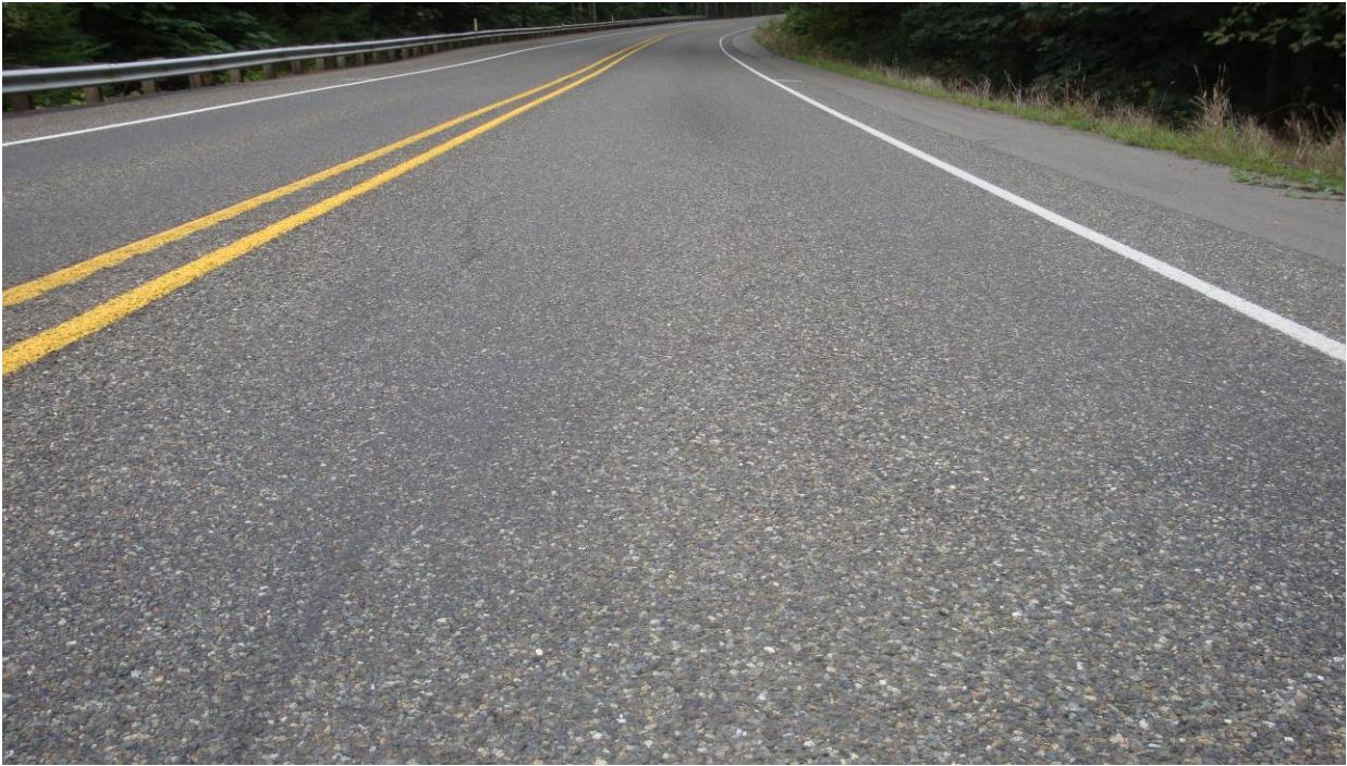
Figure 25. OR1b, SR101, one year after installation. Slight flushing in the wheel paths, one longitudinal crack in the left wheel path.
