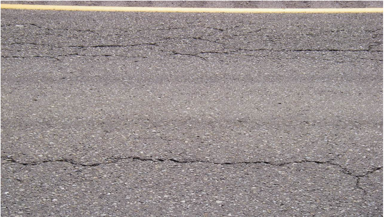
Figure 15. OR1, SR101, prior to treatment. Cracks exceed 1/4 inch in width in places.
