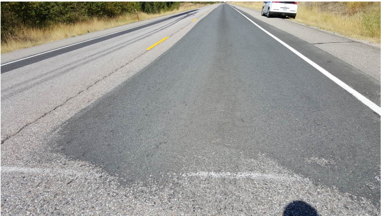
Figure 115. ER9a, SR395, one year after installation. Some wear of the blade patch at each end. Transverse cracks reflected through the blade patch after only one year.
