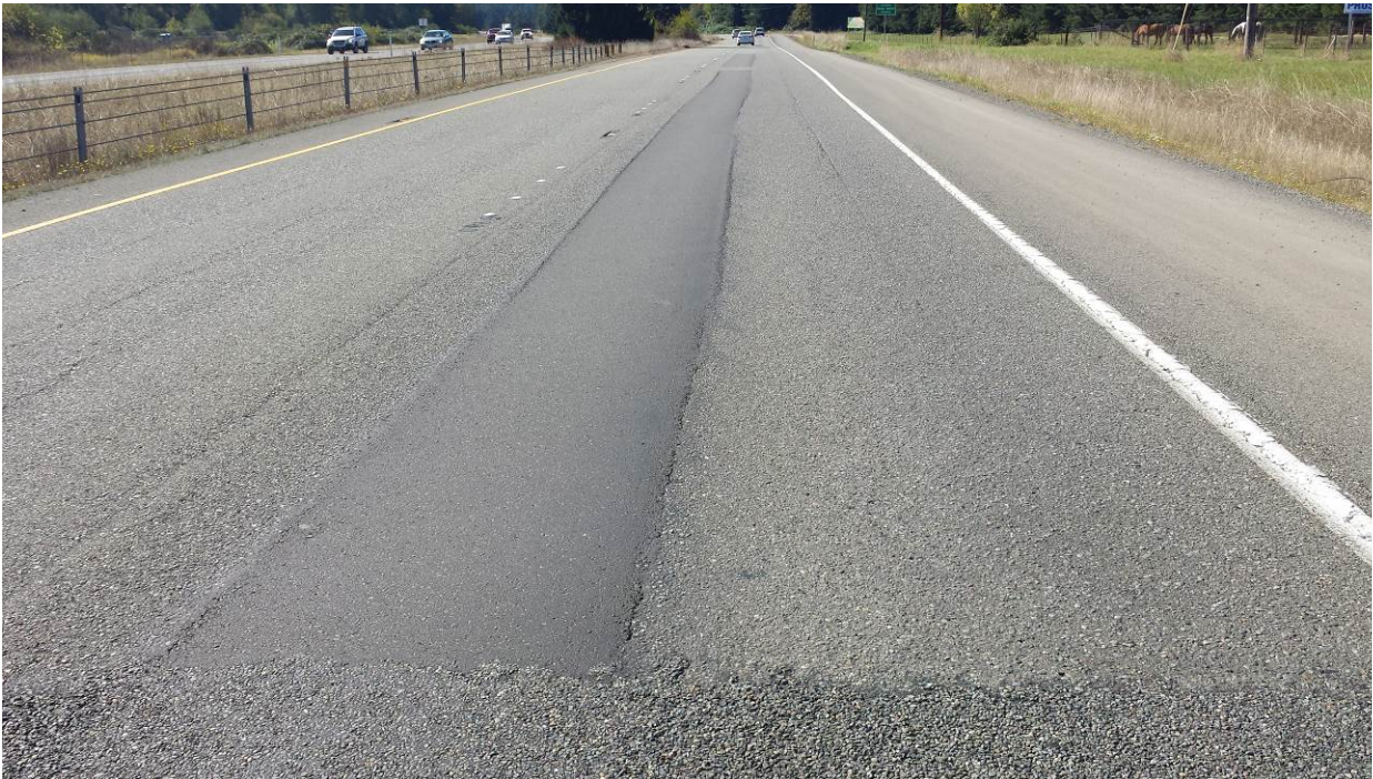
Figure 76. OR2, SR8, two years after installation. No change in condition of patch.
