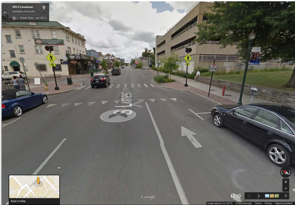
Figure 15: Midblock Crossing with Curb Extensions
