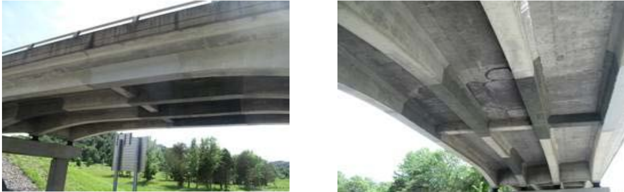
Figure 14 Retrofit Inspection - May 2017
