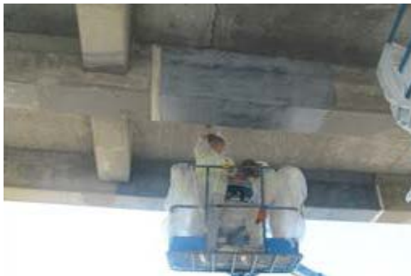
Figure 12 Applying Outer Layer of Epoxy
