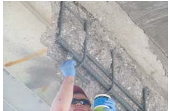
Figure 8 Blast Cleaning and Coating Exposed Steel
