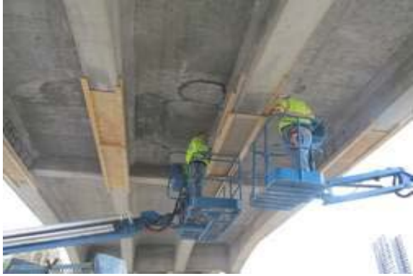
Figure 9 Attaching Forms and Placing Repair Mortar
