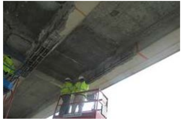
Figure 7 Removing Loose Concrete
