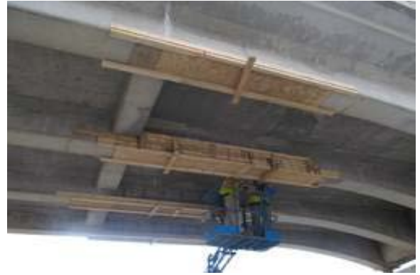
Figure 9 Attaching Forms and Placing Repair Mortar
