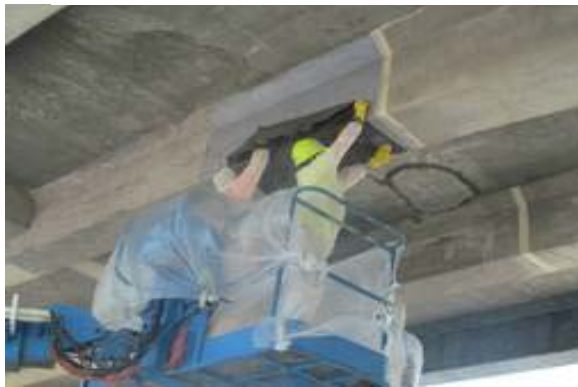
Figure 11 Applying CFRP Fabric
