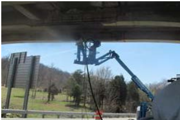
Figure 8 Blast Cleaning and Coating Exposed Steel
