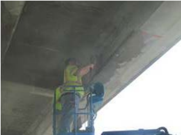
Figure 10 Preparing the CFRP Application Surface
