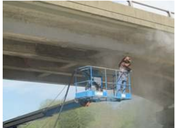
Figure 10 Preparing the CFRP Application Surface
