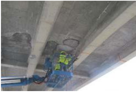
Figure 7 Removing Loose Concrete
