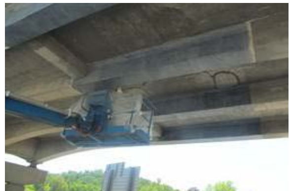
Figure 12 Applying Outer Layer of Epoxy
