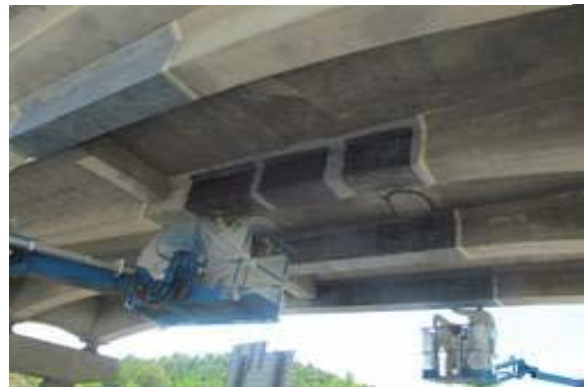
Figure 11 Applying CFRP Fabric
