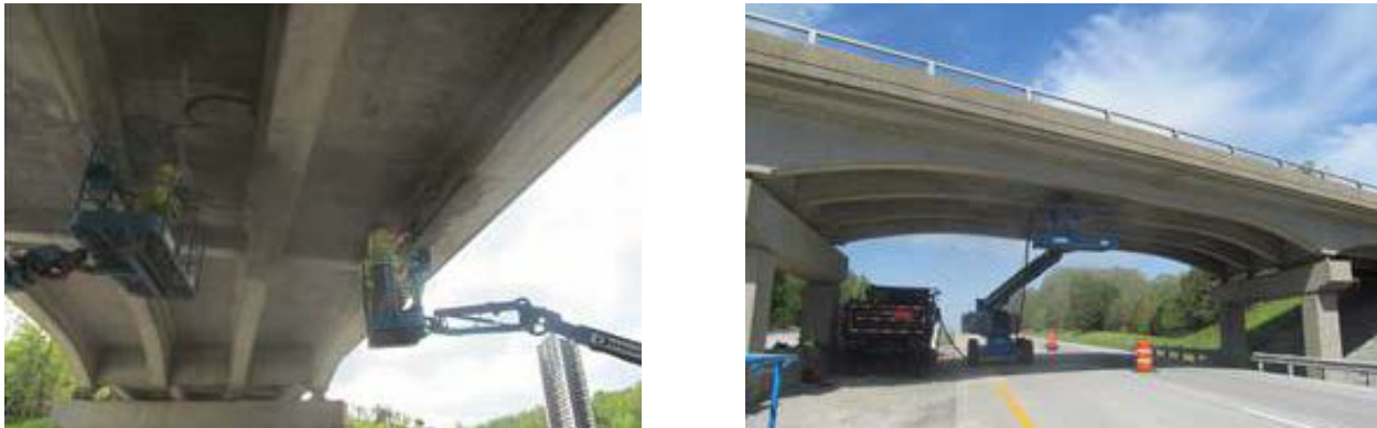
Figure 6 Multiple Man-Lifts Used in Retrofit with a Single Lane Closure
