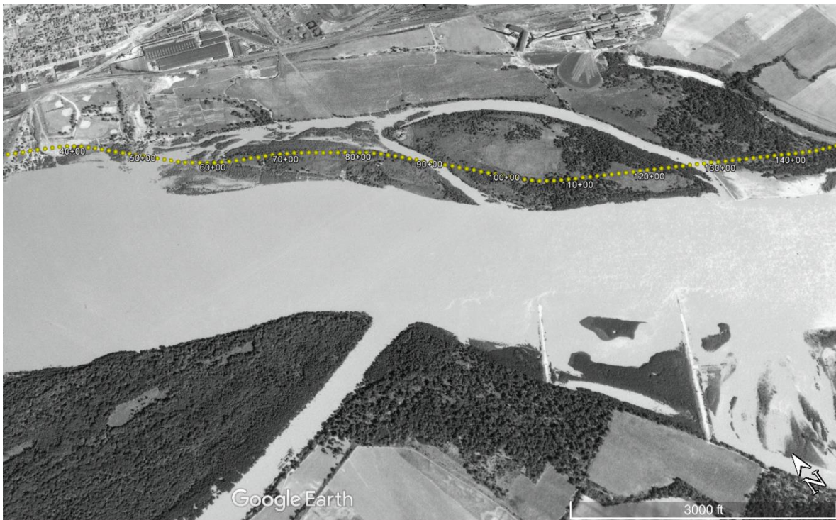
Figure 3-11-Aerial photo taken in 1941 of the future location of the Mel-Price reach of the Wood River levee with the levee stations overlaid.
