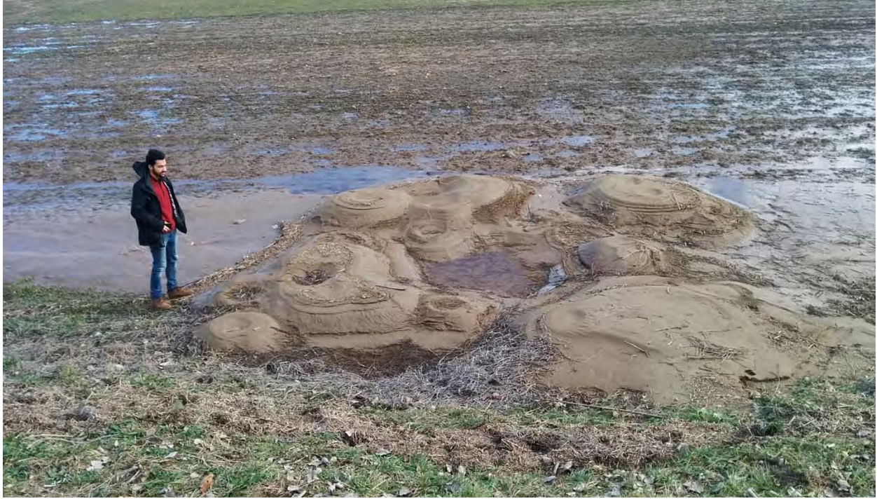
Figure 2-6 - Large sand boil network at levee toe near Olive Branch, IL (Rutherford et al., 2016)
