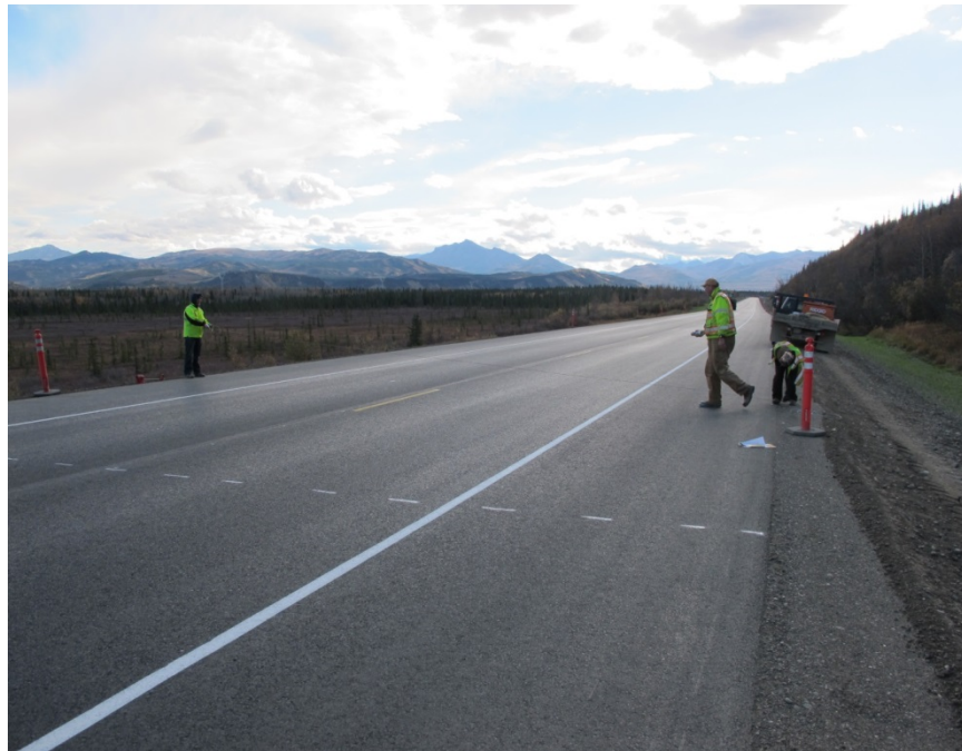
Figure 3.4 Surveyors laying out precuts with rabbit-tracks
