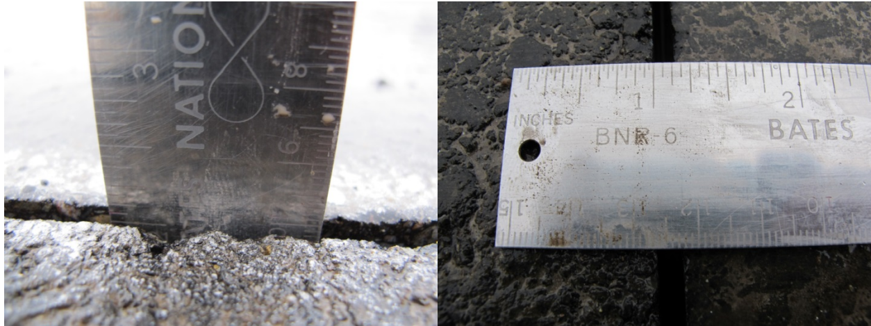
Figure 3.6 Inspection of sawn crack depth and width
