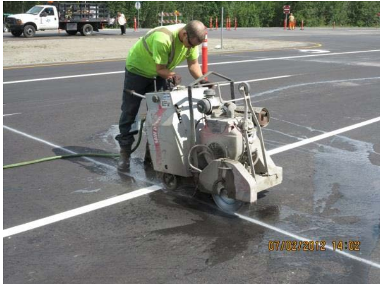
Figure 3.2 Saw Devil equipment and operator
