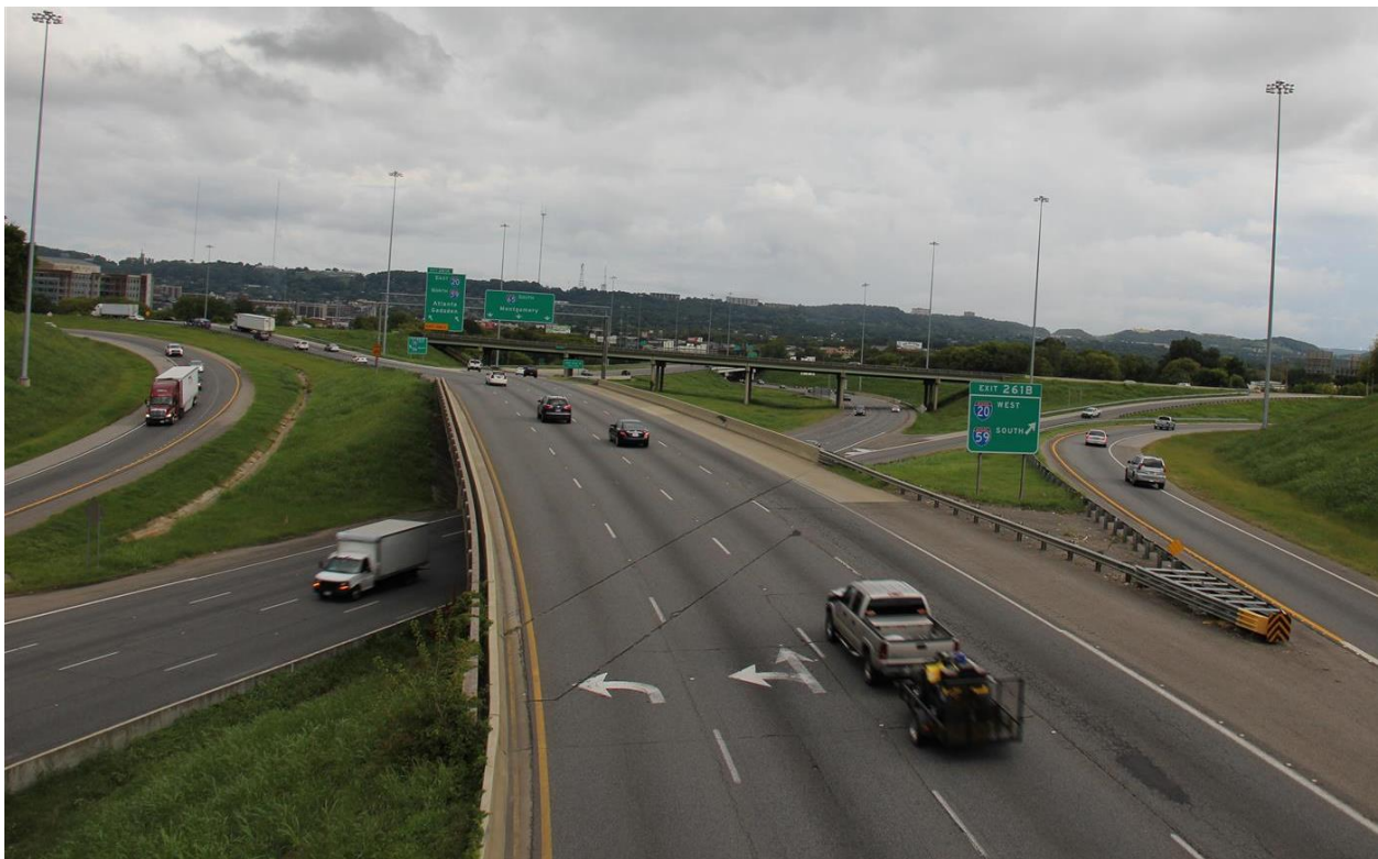
Figure 5-1. SB I-65 at milepost 261
