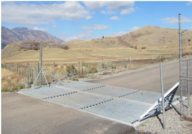
Figure 20. Double Cattle Guard (15 feet by 33 feet, 4.6 m × 7 m) Suspended over Excavation Pit (A), and Close View of Cattle Guard Rails (B), on an Access Road to U.S. Highway 91, MP 11, North of Mantua, Utah. Taken from Flower 2016.
