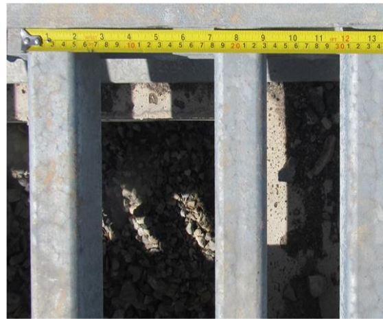
Figure 20. Double Cattle Guard (15 feet by 33 feet, 4.6 m × 7 m) Suspended over Excavation Pit (A), and Close View of Cattle Guard Rails (B), on an Access Road to U.S. Highway 91, MP 11, North of Mantua, Utah. Taken from Flower 2016.
