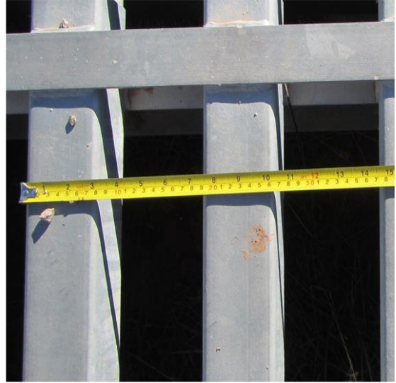
Figure 19. Standard Cattle Guard, 6.9 feet x 36 feet (2.1 m × 11 m), over Excavation Pit (A), and Close View of Cattle Guard Rails (B) on an Access Road to Interstate 15, MP 31, Near Pintura, UT. Taken from Flower 2016.
