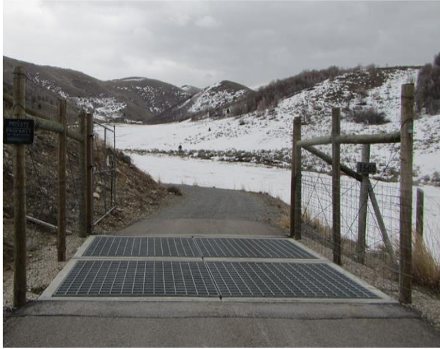
Figure 21. Wildlife Guard (16 by 16 feet, 4.9 m × 4.9 m) Suspended Over Excavation Pit (A), and Close View of Steel Grating (B) on an Access Road to U.S. Highway 91, MP 6, near Mantua, Utah. Taken from Flower 2016.
