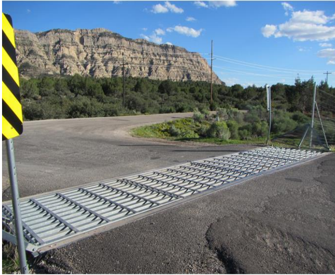
Figure 19. Standard Cattle Guard, 6.9 feet x 36 feet (2.1 m × 11 m), over Excavation Pit (A), and Close View of Cattle Guard Rails (B) on an Access Road to Interstate 15, MP 31, Near Pintura, UT. Taken from Flower 2016.
