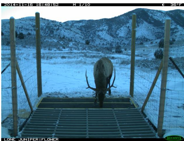
Figure 7. Bull Elk is Repelled from Electric Pavement at Hardware Ranch, UT.
