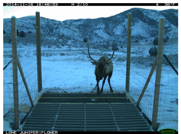
Figure 7. Bull Elk is Repelled from Electric Pavement at Hardware Ranch, UT.
