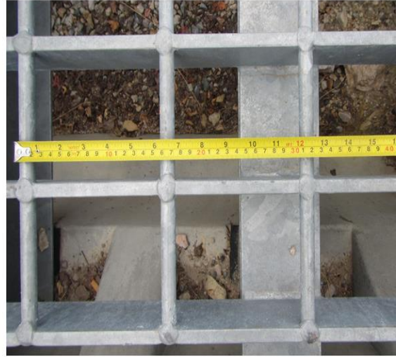
Figure 21. Wildlife Guard (16 by 16 feet, 4.9 m × 4.9 m) Suspended Over Excavation Pit (A), and Close View of Steel Grating (B) on an Access Road to U.S. Highway 91, MP 6, near Mantua, Utah. Taken from Flower 2016.
