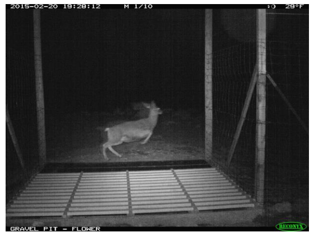
Figure 6. Mule Deer Doe is Repelled from Electric Pavement at Hardware Ranch, UT.
