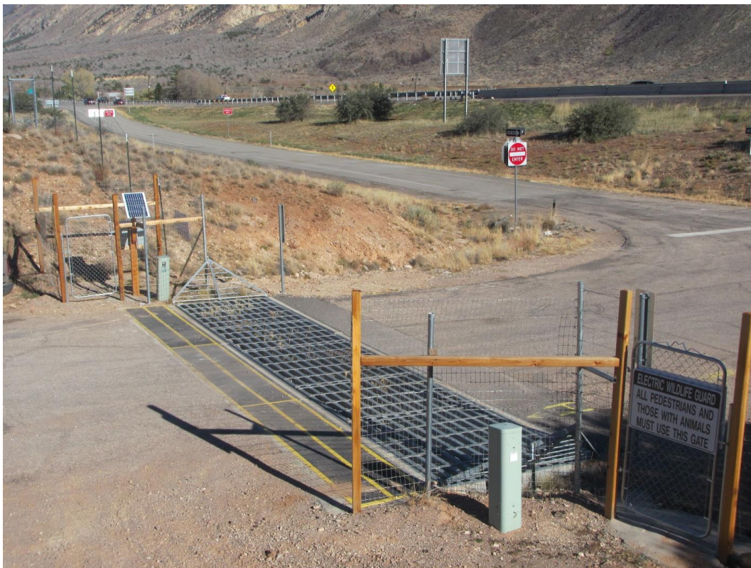
Figure 4. Cattle Guard Augmented with Electric Pavement 3 x 36 feet at West Access Road to I-15 at Exit 31, Near Pintura, Utah.
