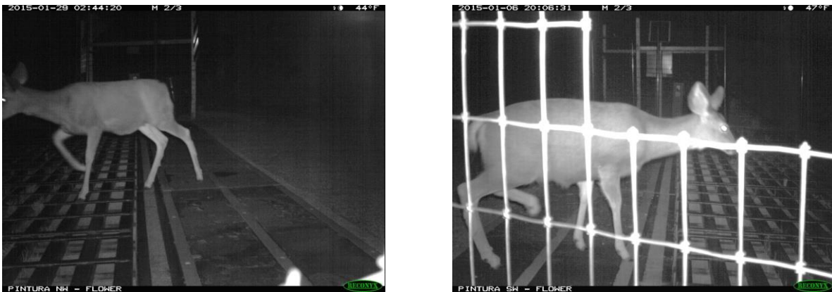
Figure 13. Two Examples of Mule Deer Does Walking Across I-15 Pintura Electric Pavement.
