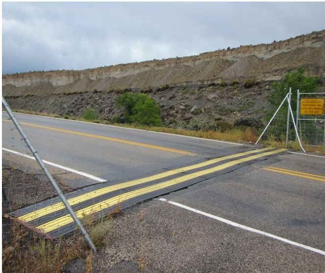
Figure 22. Electrified Mat (4 feet by 36 feet, 1.2 m × 11 m, A) and Close View of Composite Planks with Embedded Metal Electrodes (B), on an Access Road to U.S. Highway 6, MP 236, Near Helper, Utah.
