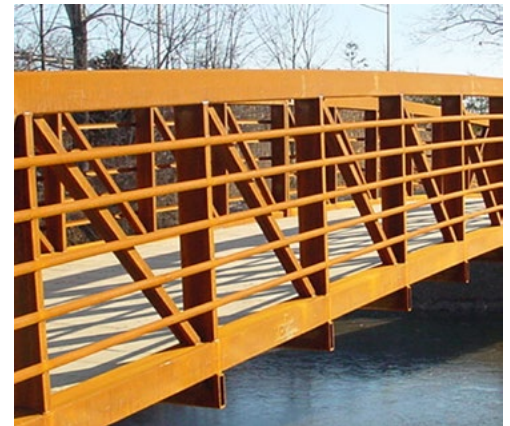
Weathering steel develops an even coat of oxide that resists corrosion and does not need painting.
