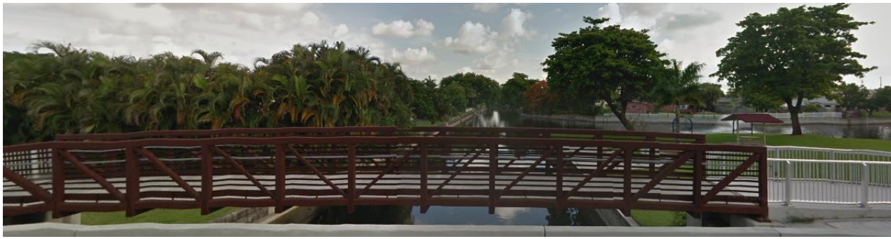
Figure 17: Weathering steel bridge in Margate, FL.
