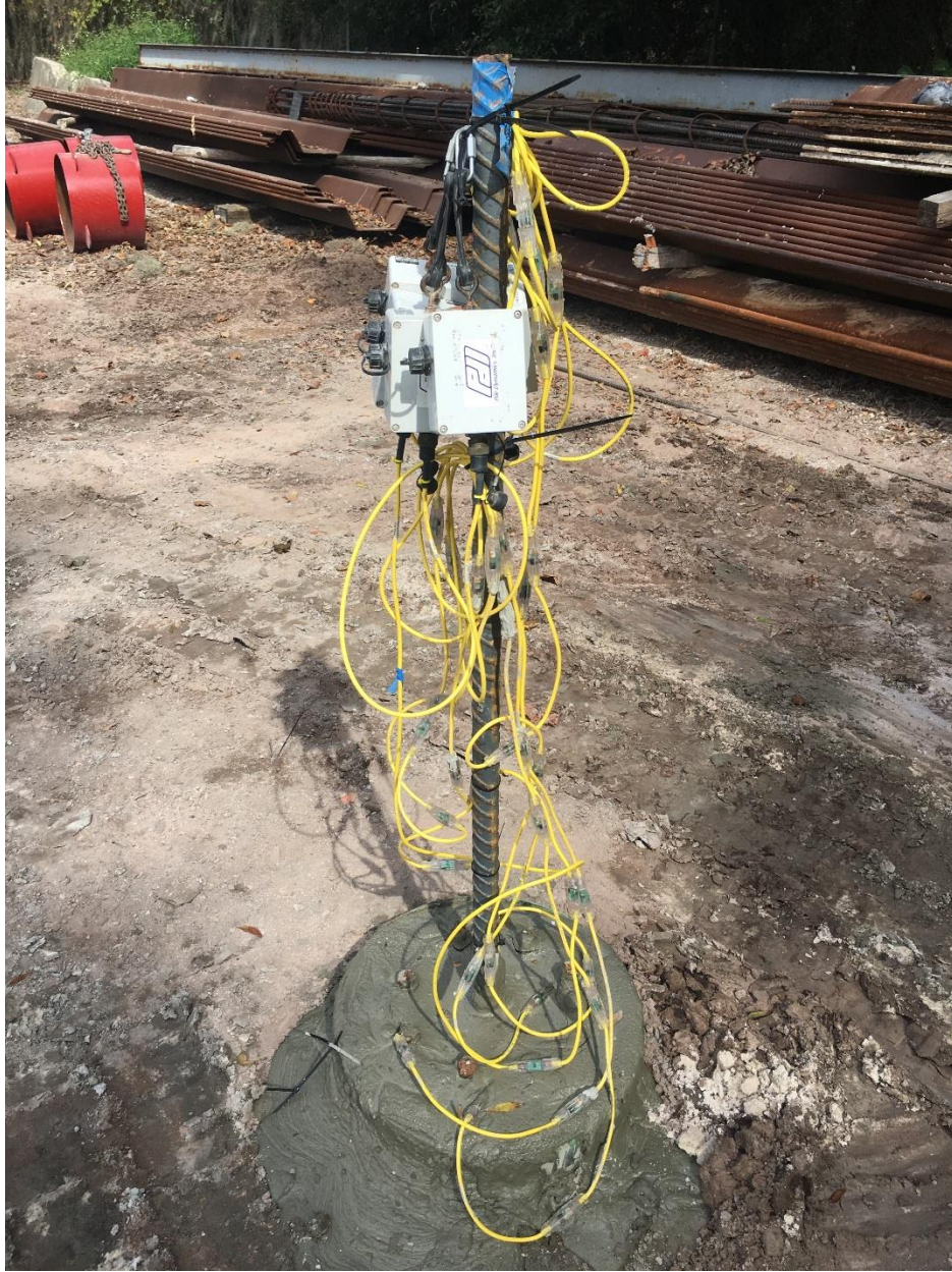
Figure 2.16 Pile L1 with thermal wires and attached TAP units.
