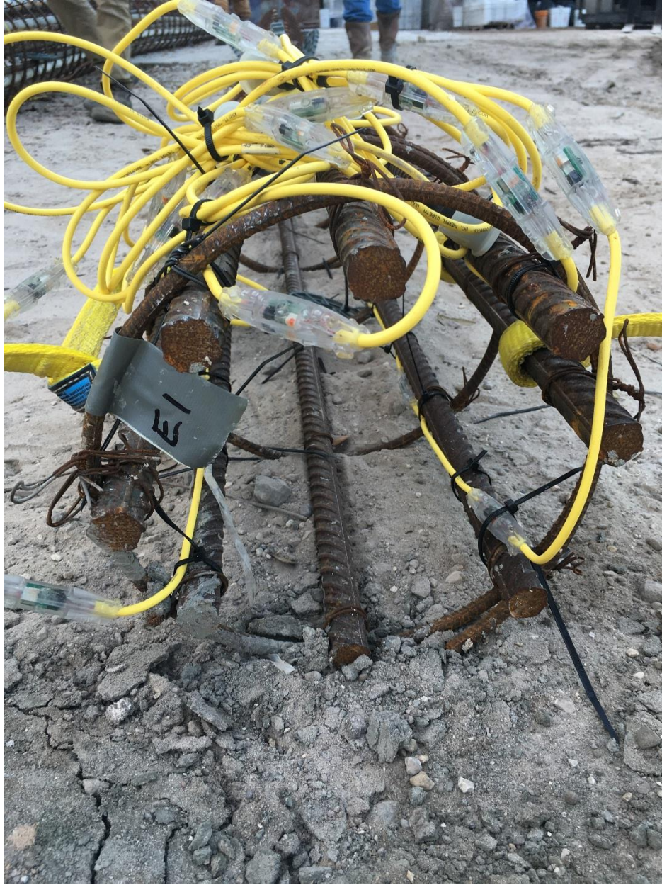
Figure 2.7 Pile E1 reinforcing cage with thermal wires attached.
