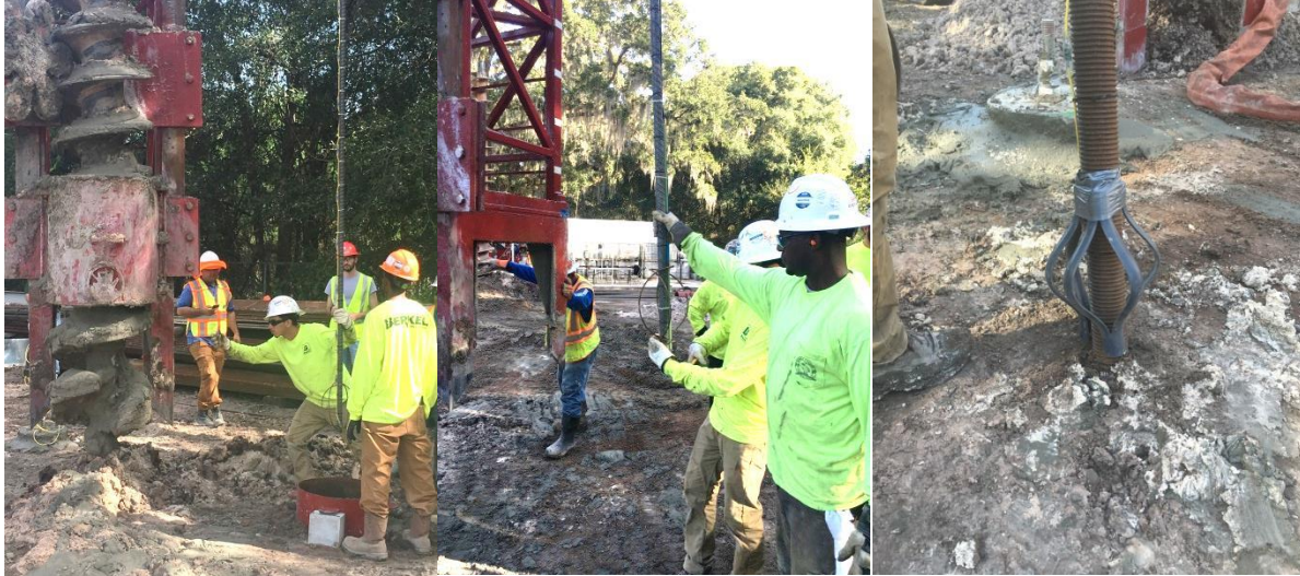
Figure 4.4 Number 8 bar with small and widely spaced centralizers \approx 10 ft (left).
