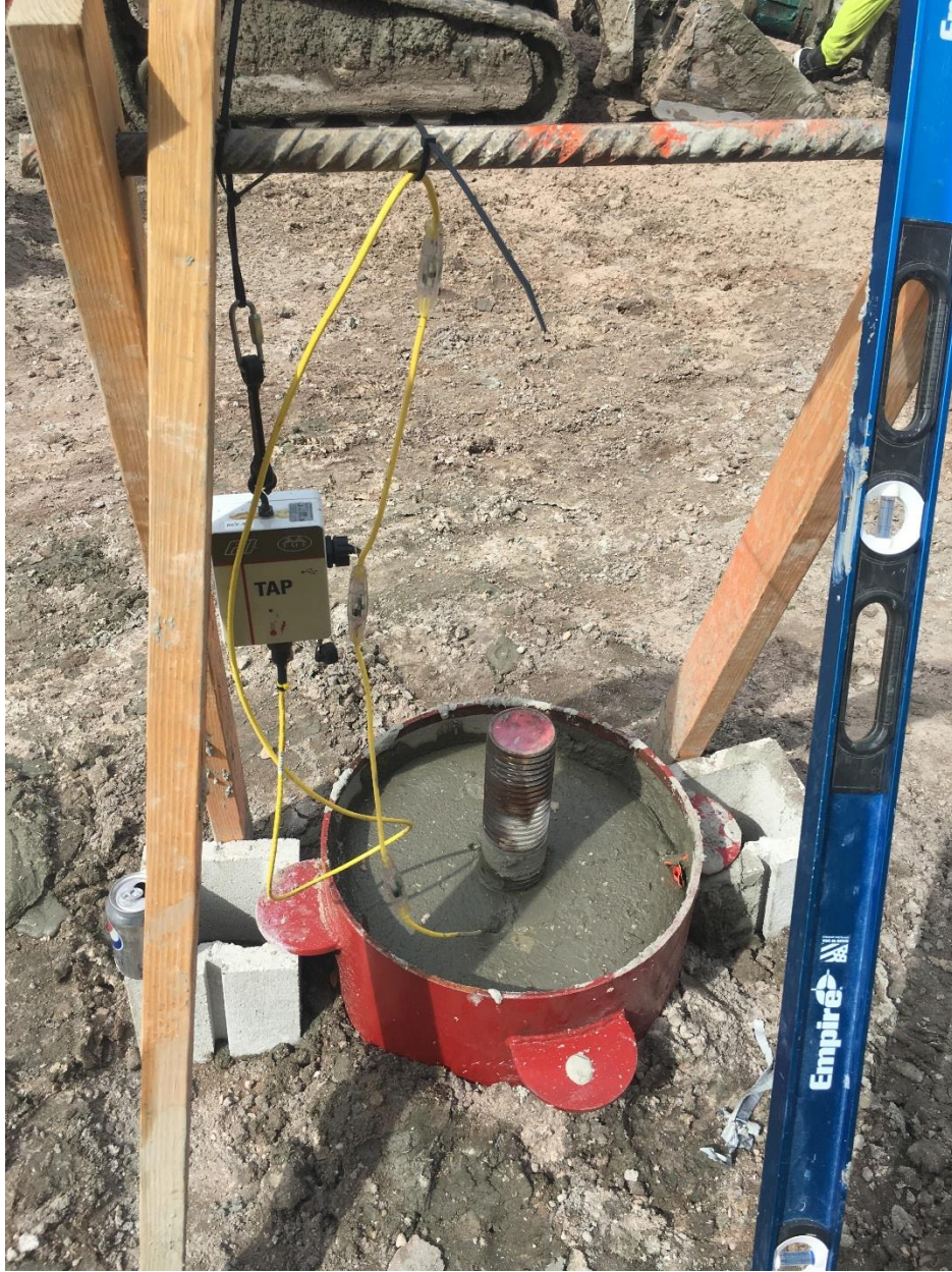
Figure 2.18 Pile T1 with thermal wires and attached TAP unit.
