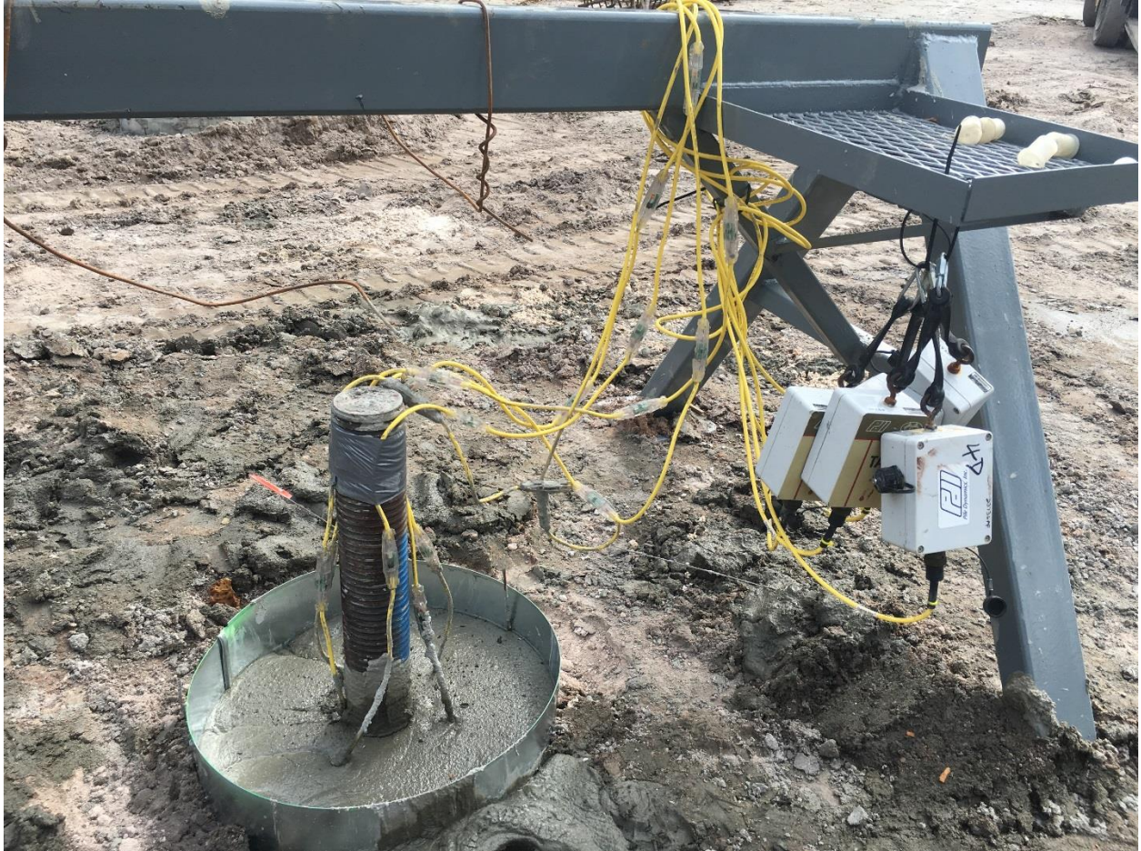
Figure 2.15 Pile E1 with thermal wires and attached TAP units.
