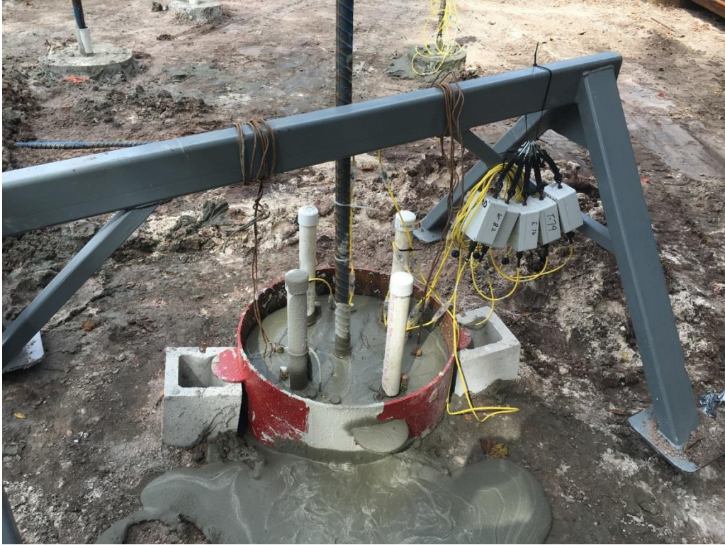
Figure 2.19 Pile L2 with thermal wires and attached TAP units.
