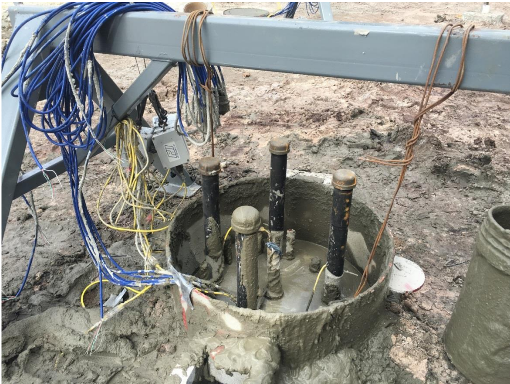
Figure 2.20 Pile C2 with thermal wires and attached TAP units.
