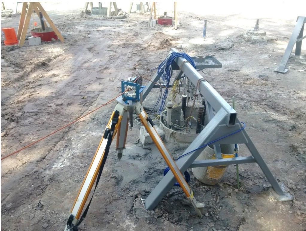
Figure 2.11 Probe testing pile C2 at approximately 24 hours after pile installation.
