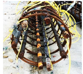
Steel reinforcing cage wired with temperature sensors before placement in concrete pile.
