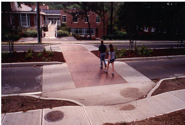
Figure A- 6. Raised crossing (PEDSAFE, 2017).
