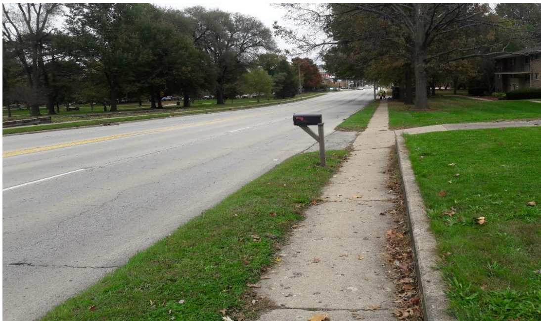
Figure E-38. Kirby Ave. Typical Roadway View.
