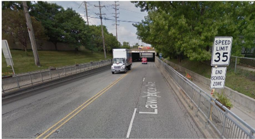
Figure 42. Example of pedestrian channelization, Cook County, Illinois.
