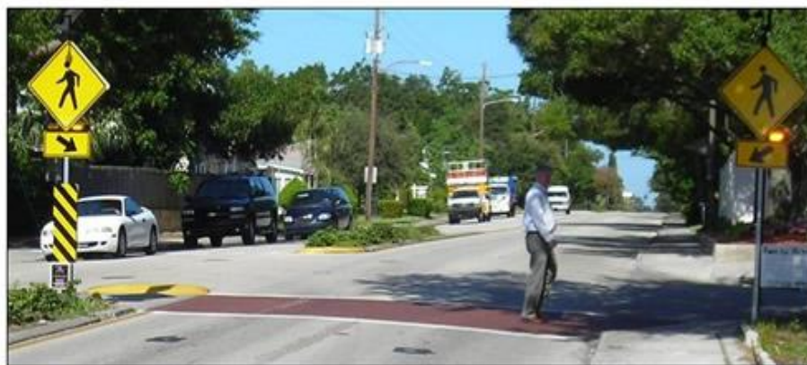
Figure A- 8. RRFB system (Pecheux et al. 2009).
