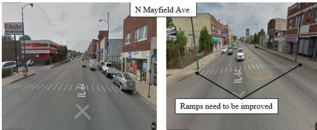
Figure E-74. Example of marked crosswalks at the intersection of W. North Ave. and N. Mayfield Ave.
