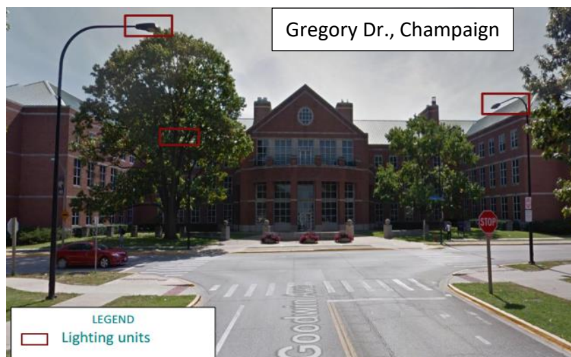
Figure 32. Example of inadequate street-lighting location.
