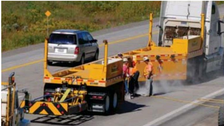
Figure 4-5 Using MBT-1 mobile work zone barrier in the field (Graham et al., 2011)
