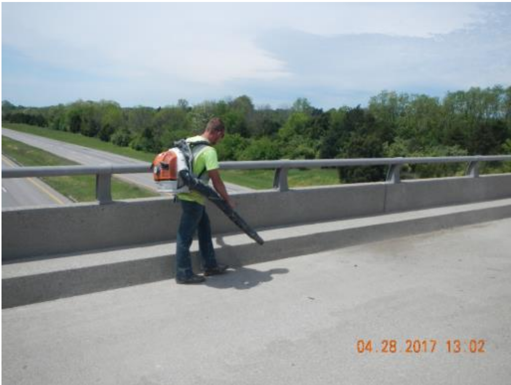
Figure 3 Removing debris with leaf blower
