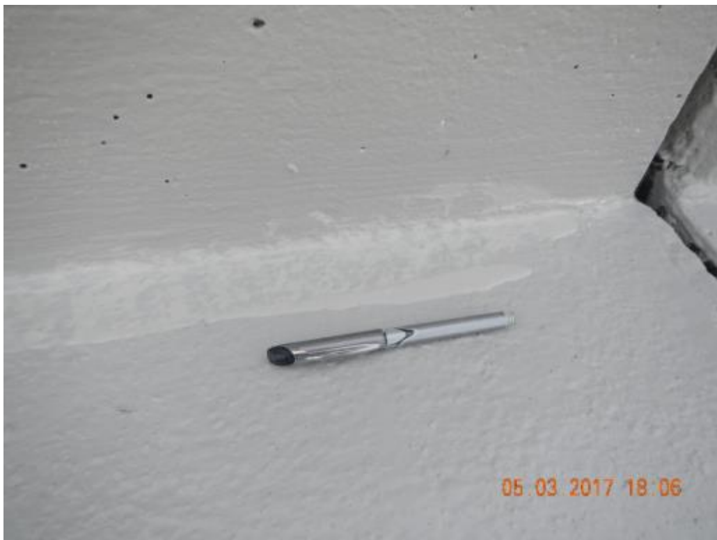
Figure 8 Excessive runs
