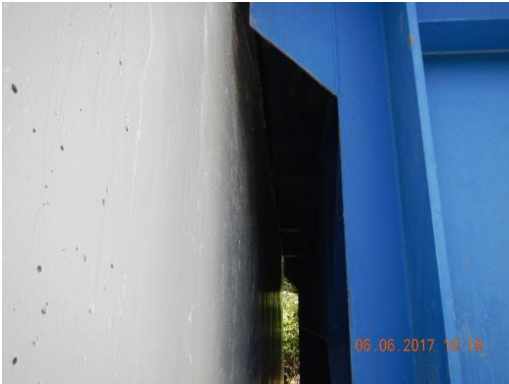
Figure 11 Back wall of abutment with floor beam in close proximity
