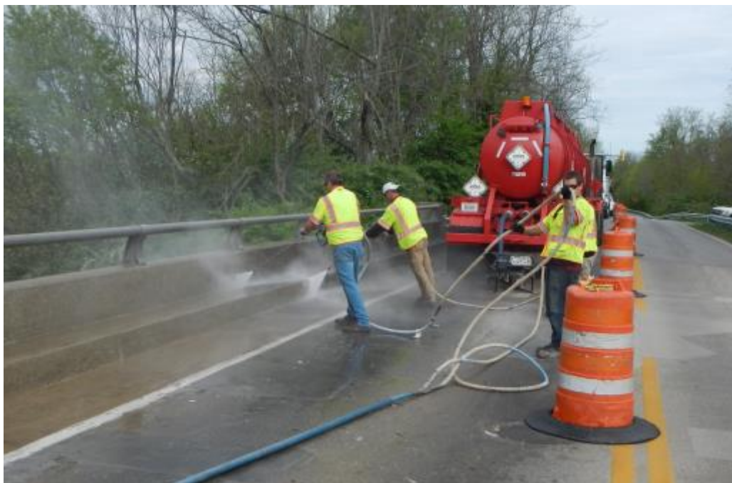
Figure 2 Washing with appropriate stand-off
