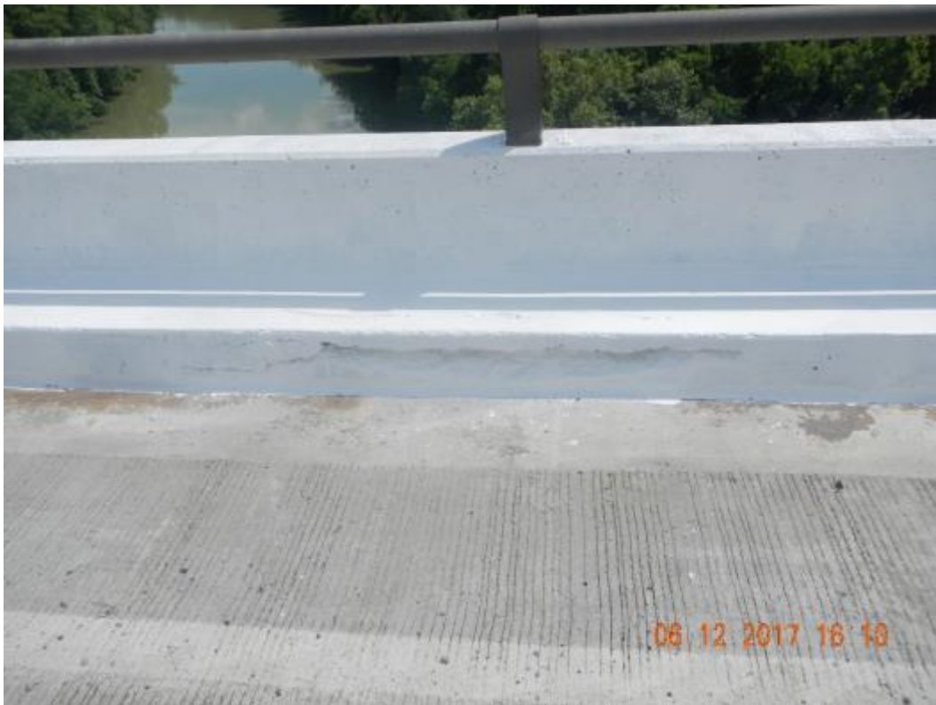
Figure 12 Spalled concrete
