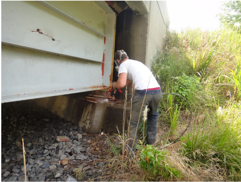
Figure 31. Worker Pressure Washing Concrete Abutment Pedestal
