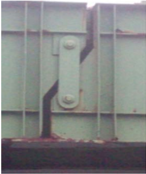
Figure 11. Pin and Hanger Bearing (13 op. cit.)
