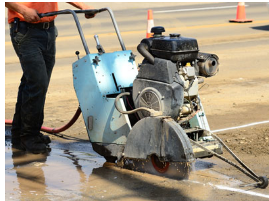
Figure 28. Concrete Sawing
