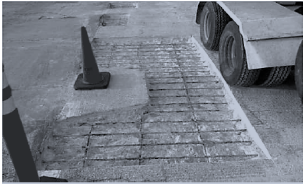
Figure 25. Partial depth repair (op. cit. 6)
