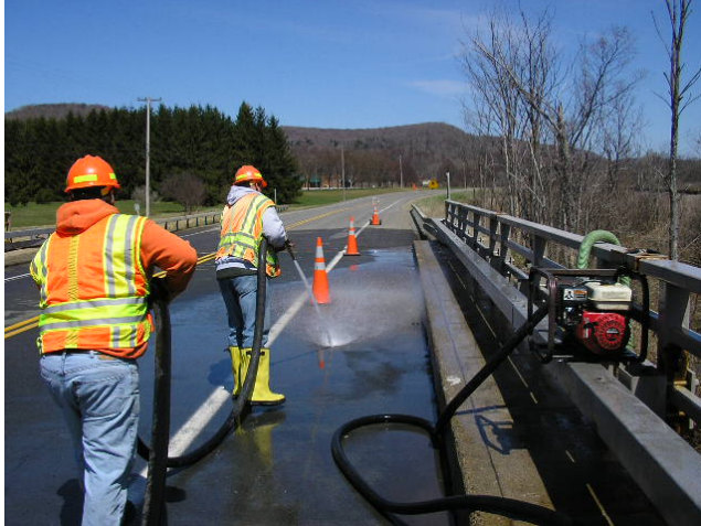
Figure 15. Workers Washing Gutter Line of Bridge Deck (Picture Courtesy of NYSDOT)
