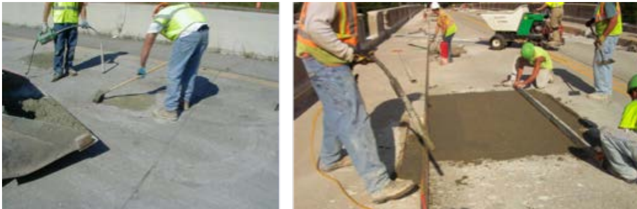
Figure 29. Placing and Finishing Repair Material
