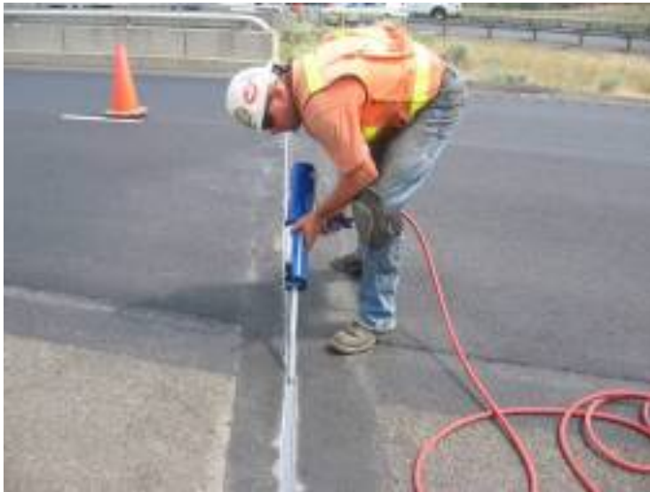
Figure 3. Worker Installing a Poured Joint Seal
