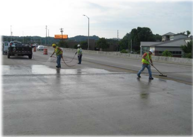
Figure 17. Sealing a Bridge Deck with a Silane
