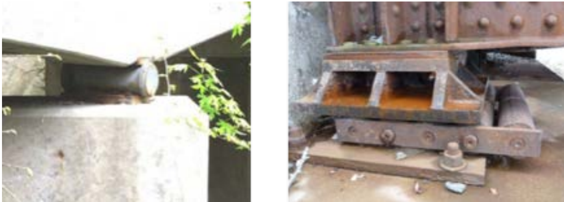
Figure 10. Roller Bearings (13). (10a) Single on left, (10b) Nested on right
