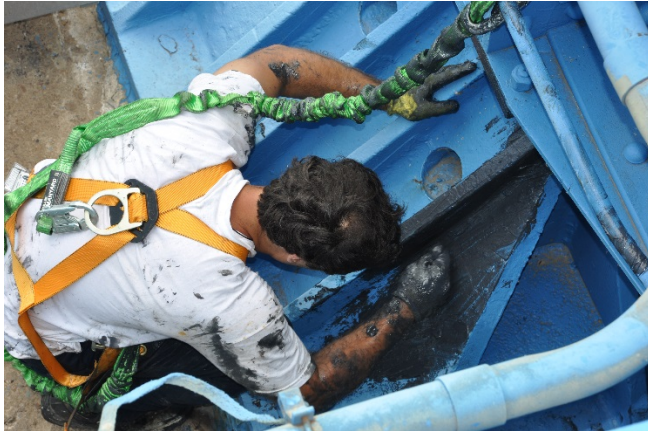
Figure 13. Lubricating a Clean Bearing
