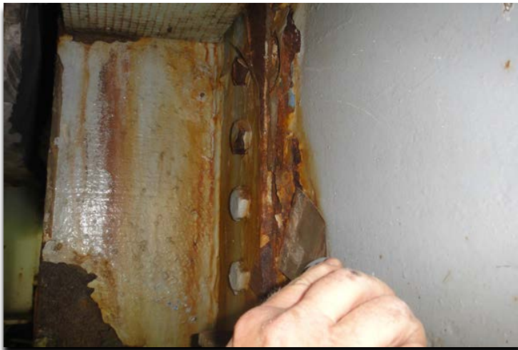
Figure 20. Removing Loose Paint with a Scraper per SSPC SP2
