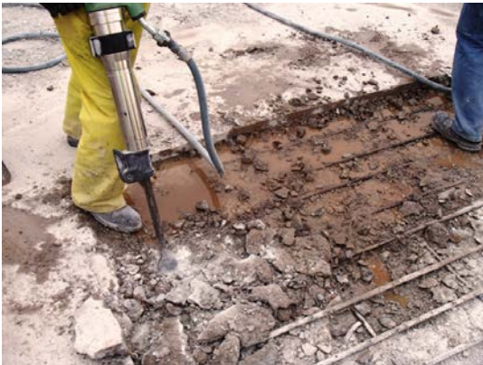
Figure 27. Concrete Removal (op. cit. 6)
