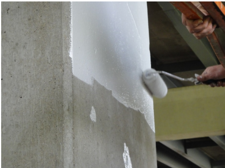
Figure 32. Painting Concrete Pier Using Roller Application
