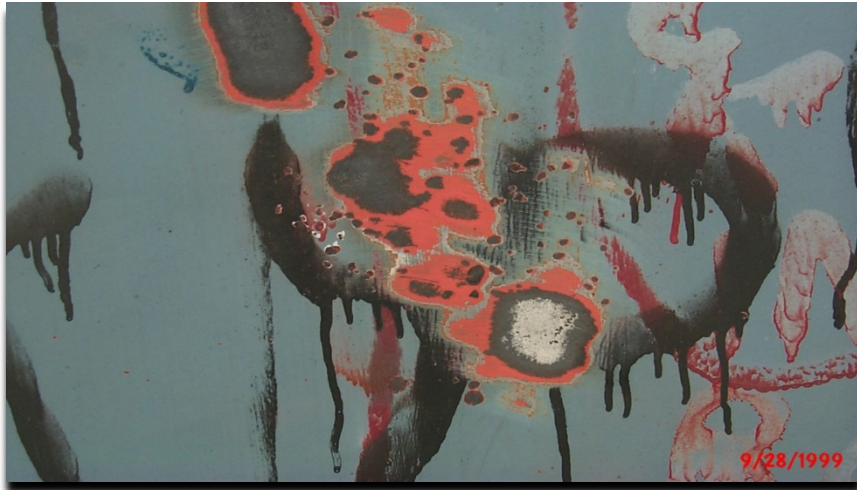
Figure 22. Feathered Edges of Existing Coating Prior to Spot Repair
