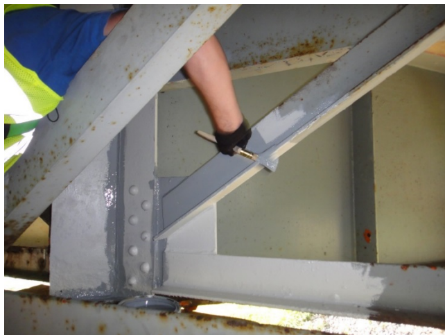
Figure 23. Spot Painting Applied with a Brush.
