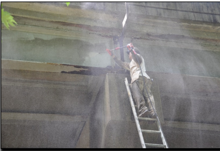
Figure 16. Worker Washing a Steel Beam End Under a Joint
