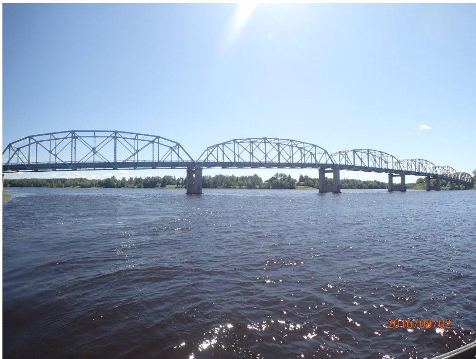
Figure 4.5 Baudette Bridge Overall Photo.
