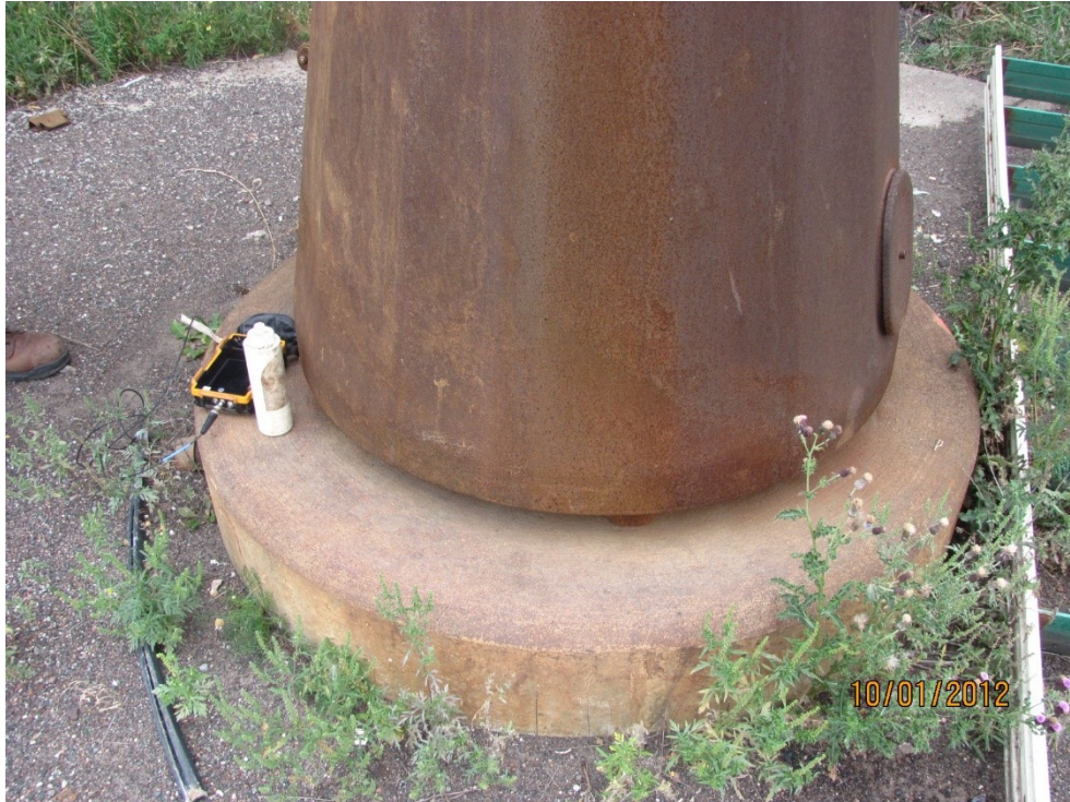
Figure 4.8 Duluth High Mast Light Base Photo.
