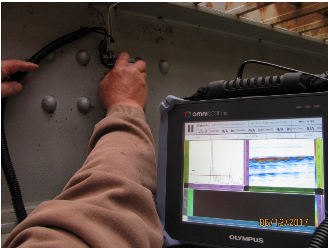
Figure 2.1 Phased array ultrasonic being utilized on steel bridge element.
