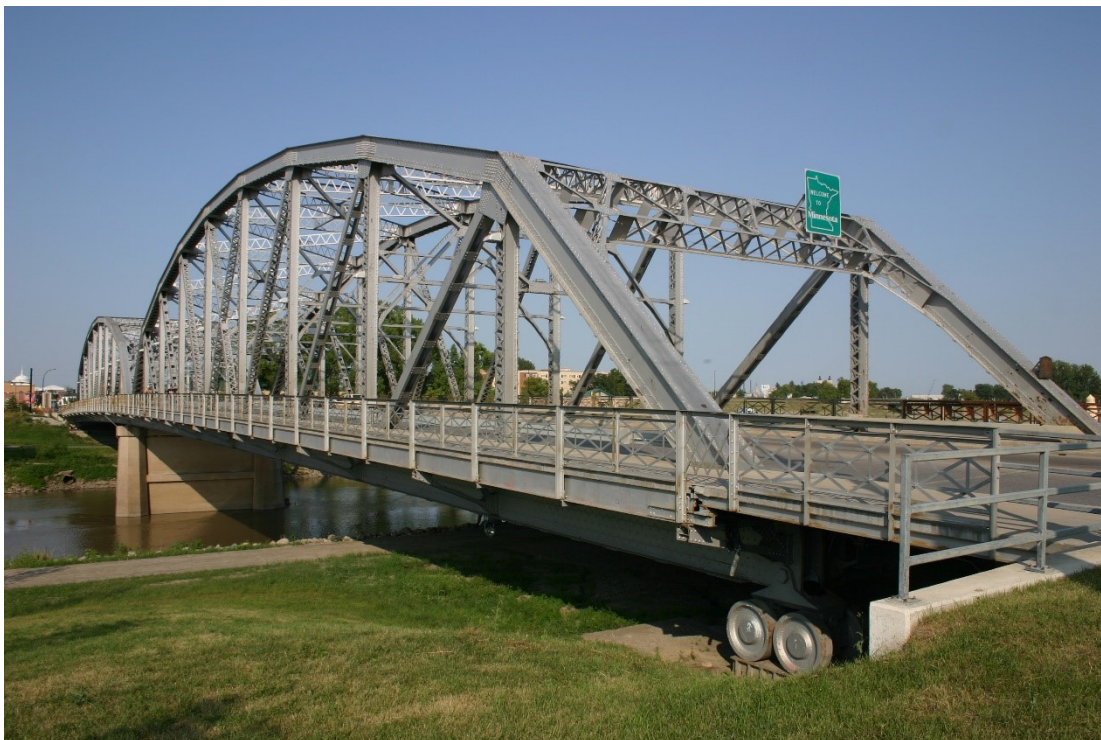
Figure 4.1 Sorlie Bridge Overall Photo.
