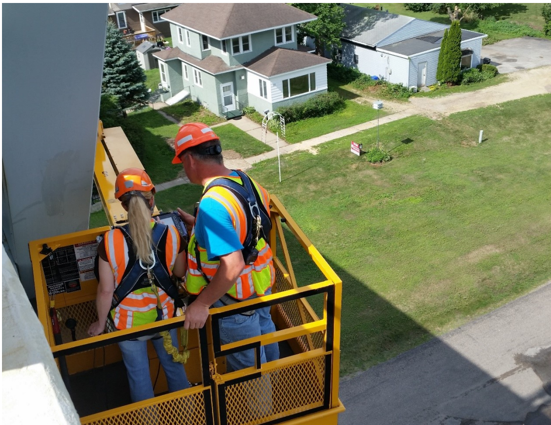
Figure 5.1 Phased Array Corrosion Mapping Field Work.
