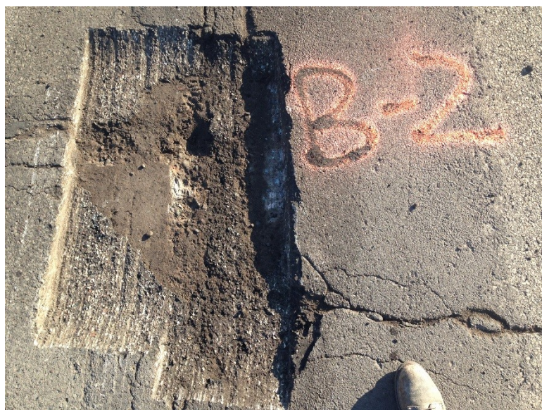
Figure 3.26 Pothole B-2 after Milling.
