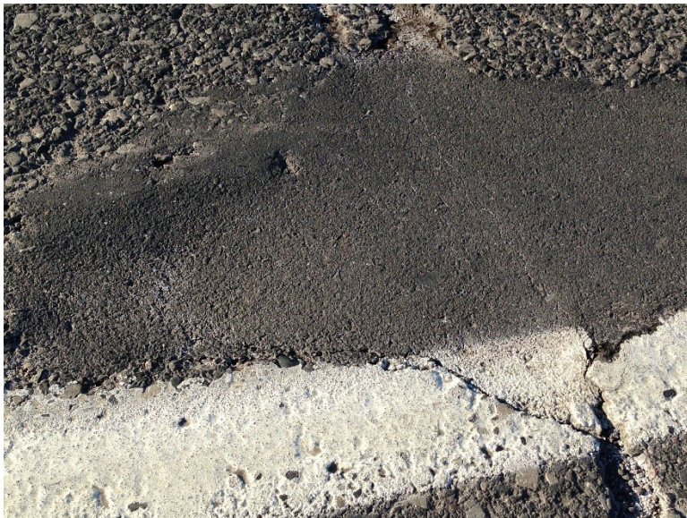
Figure 3.20 Pothole A-5 (240 Days after Installation).
