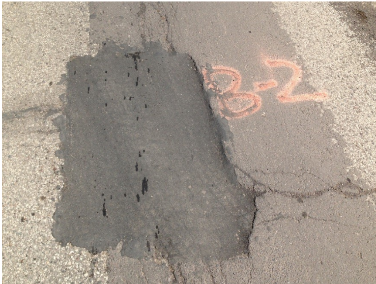
Figure 3.39 Pothole B-2 (3 Days after Patching).
