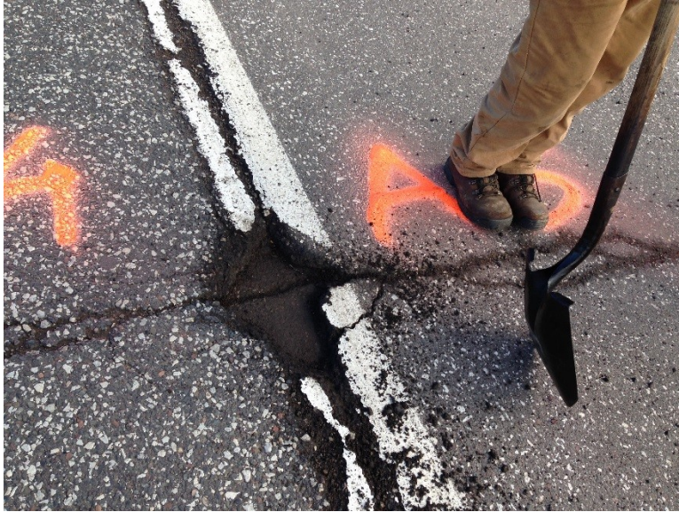
Figure 3.5 Pothole A-5 prior to Patching (After Cleaning).
