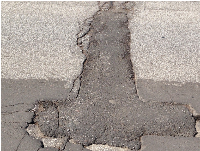
Figure 3.44 Pothole B-5 (146 Days after Patching).
