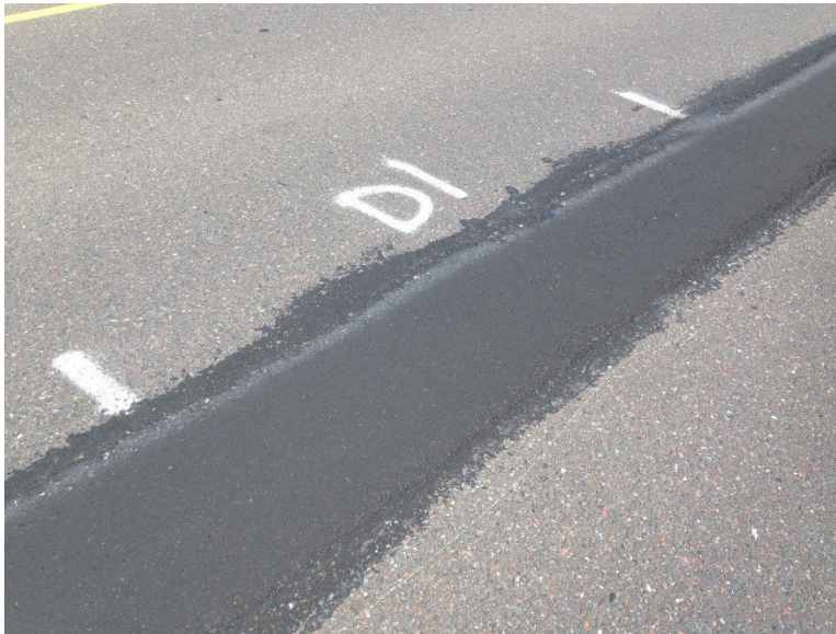
Figure 3.63 Pothole D-1 (35 Days after Patching).
