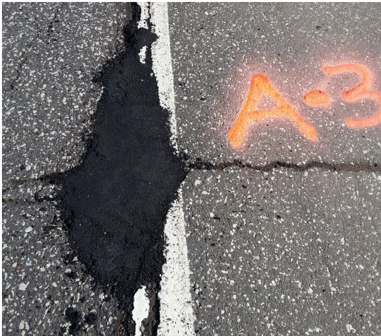
Figure 3.8 Pothole A-3 after Patching.
