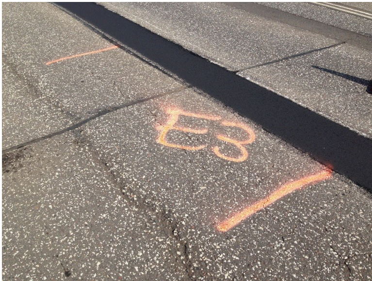
Figure 3.74 Pothole E-3 after Compaction.
