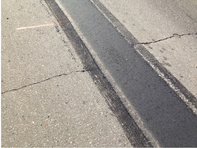
Figure 3.61 Pothole D-3 with Clean Compaction.
