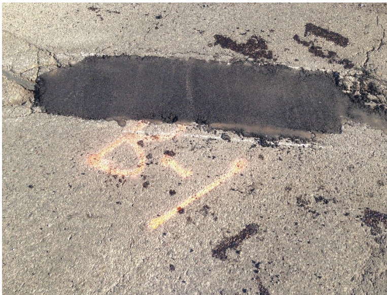
Figure 3.36 Pothole B-1 after Patching.
