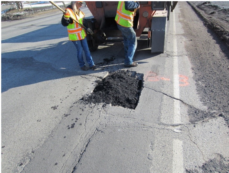
Figure B3: Cold Mix Step 3.
