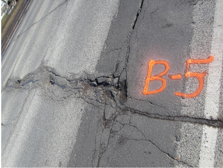
Figure 3.29 Pothole B-5 before Milling.
