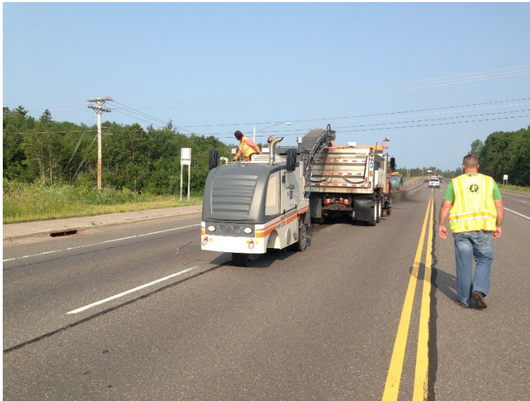
Figure B9: Mill and Fill Step 1.
