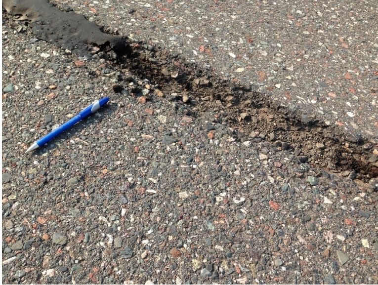
Figure 3.56 Section of Longitudinal Crack with Sealer Missing.
