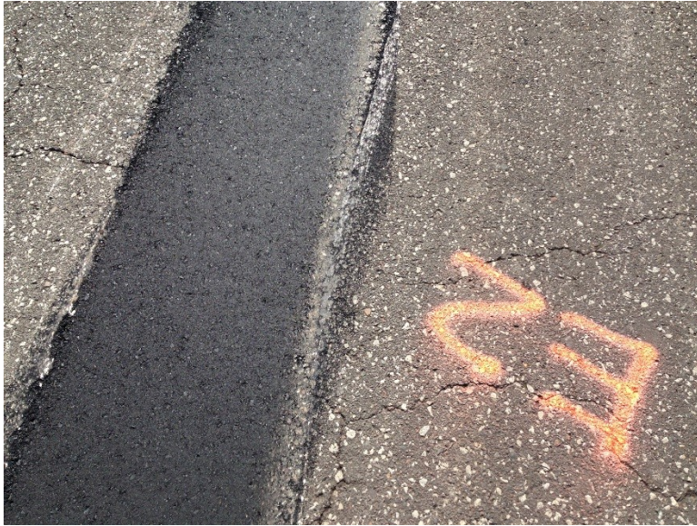
Figure 3.73 Pothole E-2 after Compaction.
