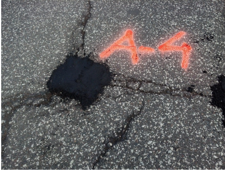
Figure 3.9 Pothole A-4 after Patching.
