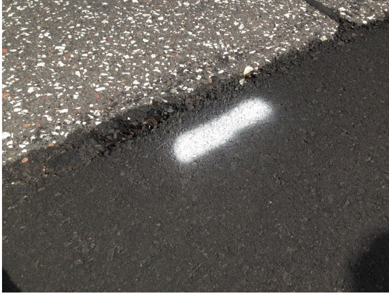
Figure 3.80 Poorly Compacted Interface (28 Days after Patching).
