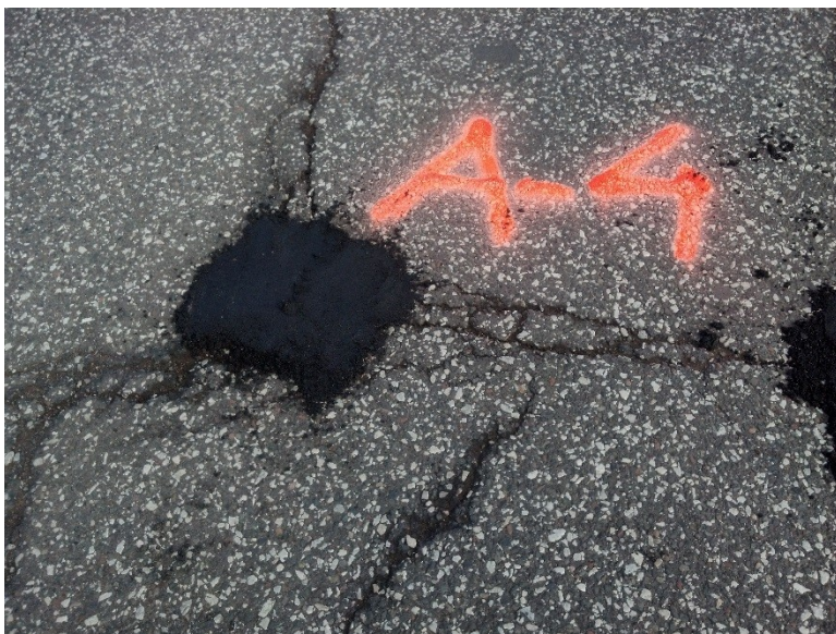
Figure 3.14 Pothole A-4 after Patching.
