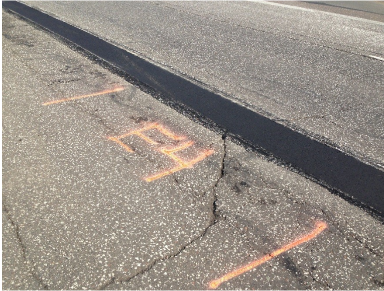
Figure 3.75 Pothole E-4 with Transverse Crack.
