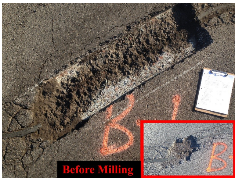
Figure 3.25 Pothole B-1 before and after Milling.
