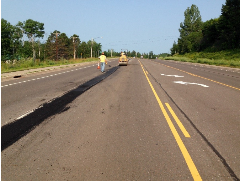
Figure B13: Mill and Fill Step 4.
