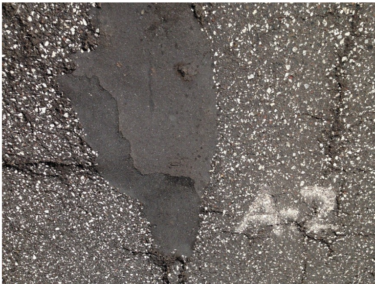
Figure 3.12 Pothole A-2 (149 Days after Patching).
