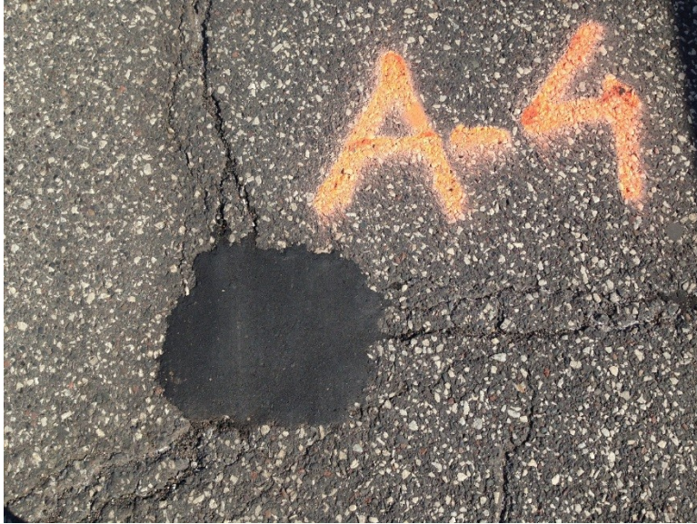
Figure 3.15 Pothole A-4 (3 Days after Patching).
