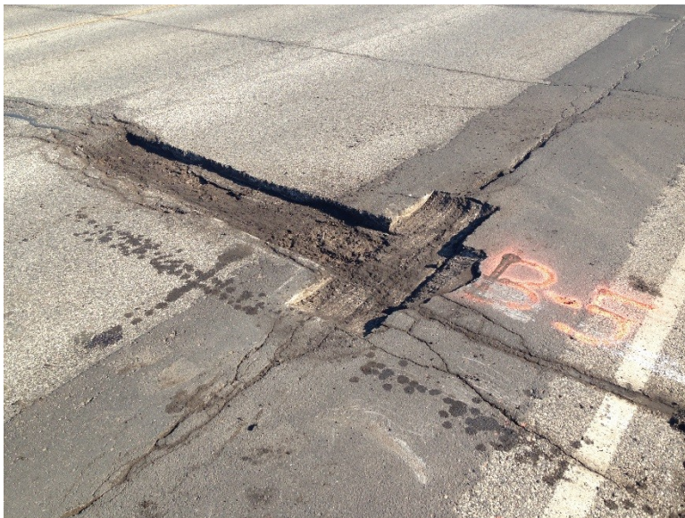
Figure 3.30 Pothole B-5 after Milling.
