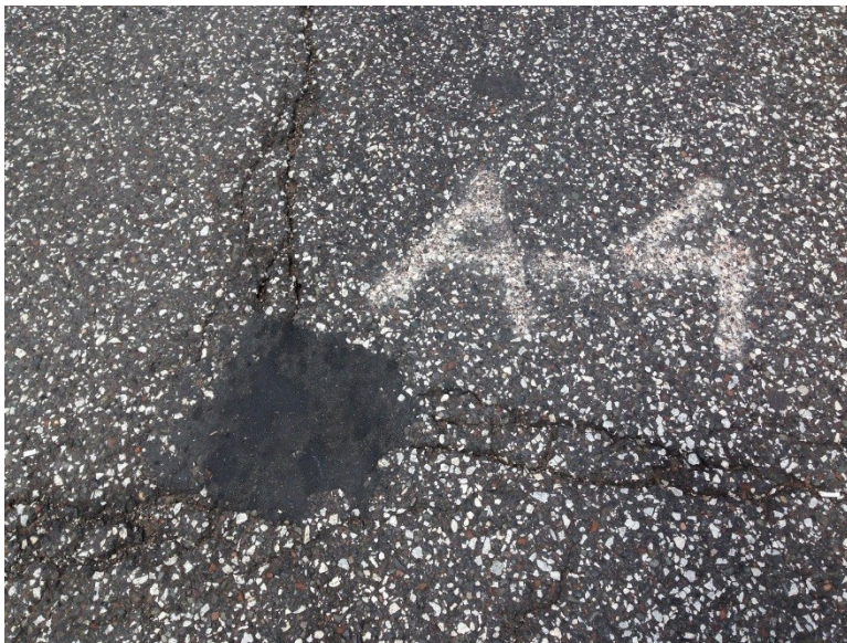
Figure 3.16 Pothole A-4 (149 Days after Patching).
