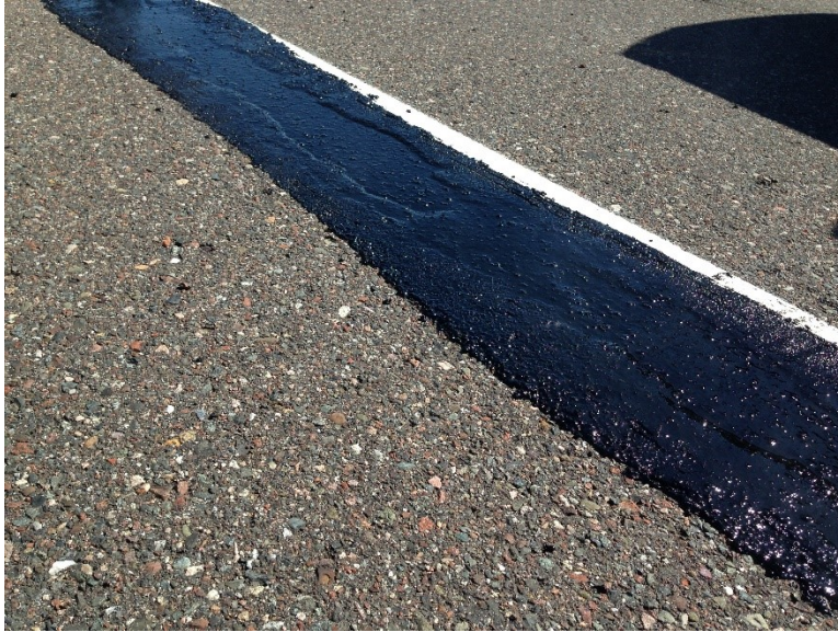
Figure 3.54 Finished Mastic Patch.
