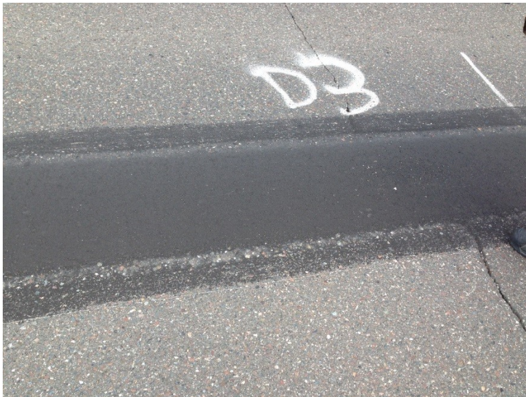
Figure 3.65 Pothole D-3 (35 Days after Patching).
