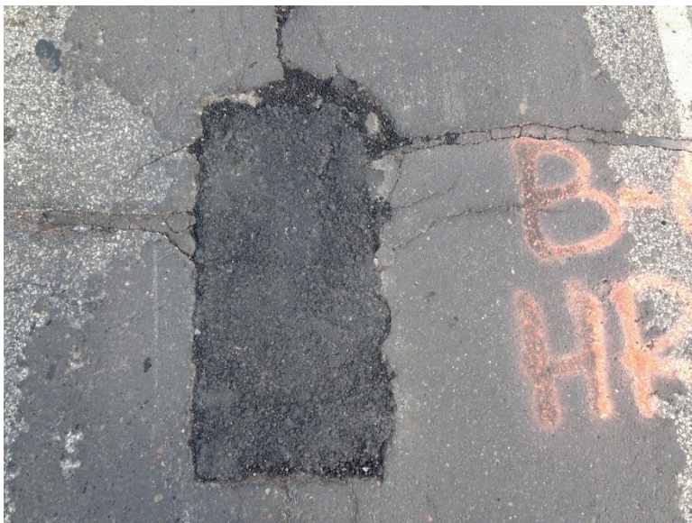
Figure 3.46 Pothole B-6 (3 Days after Patching).
