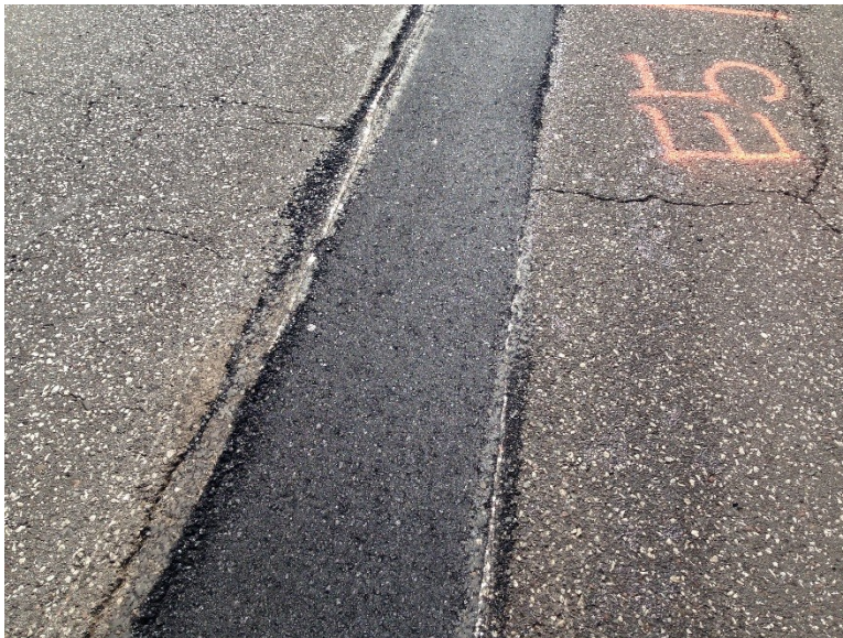
Figure 3.76 Pothole E-5 after Compaction.
