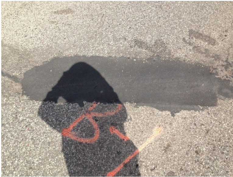
Figure 3.37 Pothole B-1 (3 Days after Patching).
