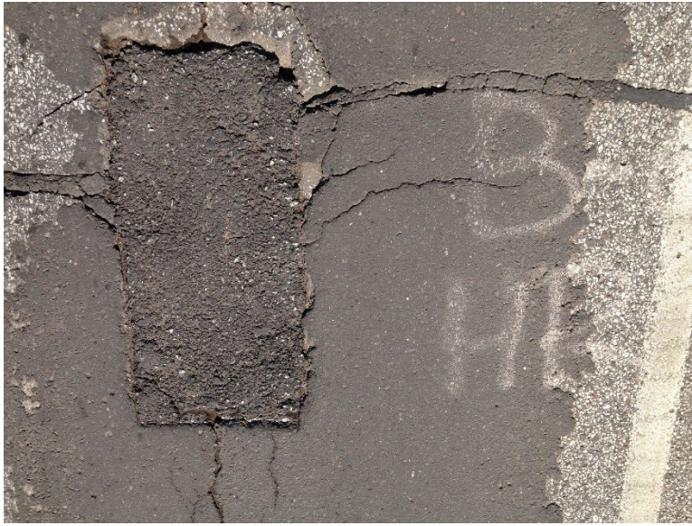
Figure 3.47 Pothole B-6 (146 Days after Patching).
