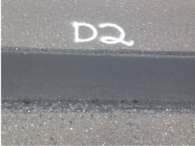
Figure 3.64 Pothole D-2 (35 Days after Patching).
