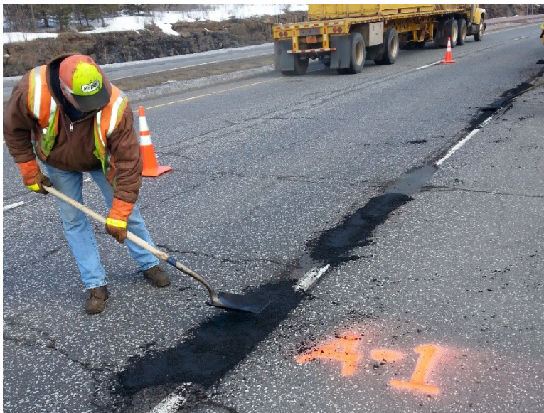
Figure 3.6 Pothole A-1 after Patching.
