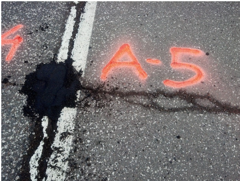
Figure 3.10 Pothole A-5 after Patching.
