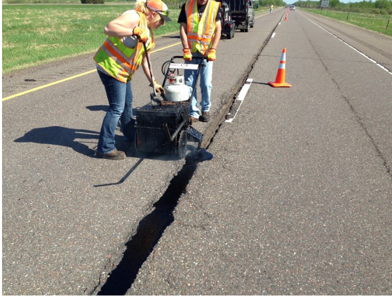
Figure 3.52 Filling Longitudinal Crack with Mastic.
