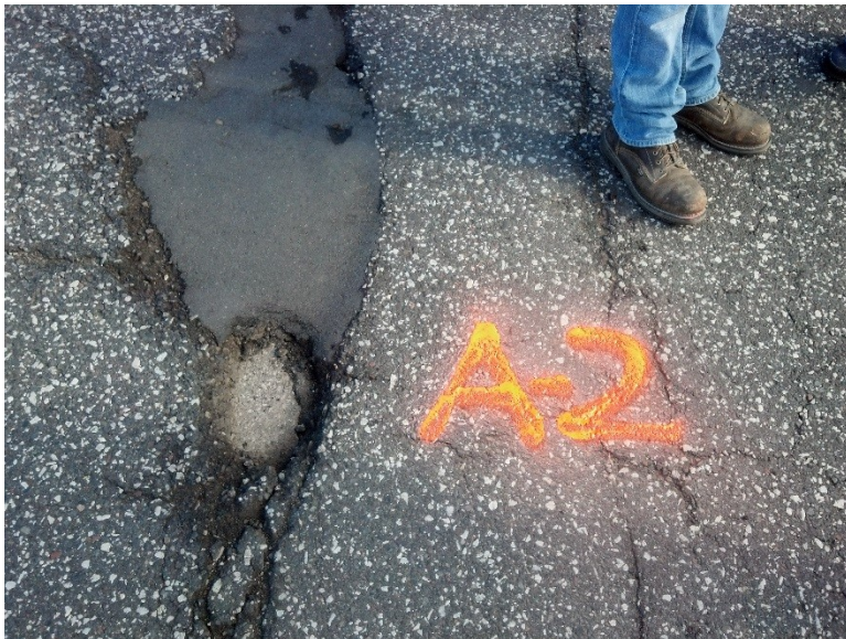
Figure 3.2 Pothole A-2 prior to Patching (After Cleaning).
