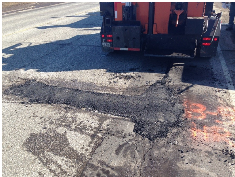
Figure 3.42 Pothole B-5 after Patching.
