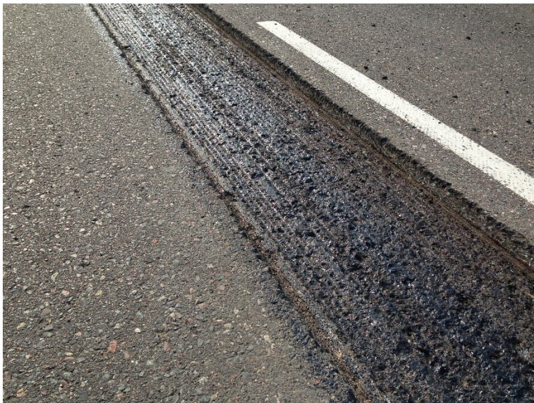
Figure 3.57 Milled Trench.
