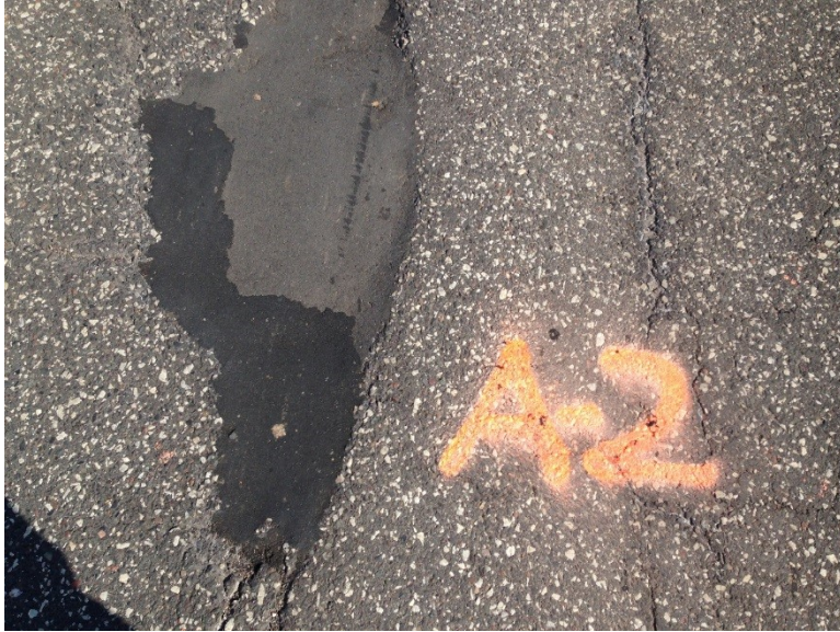
Figure 3.11 Pothole A-2 (3 Days after Patching).
