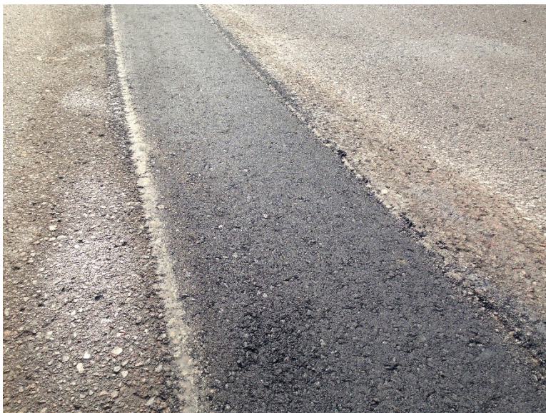
Figure 3.60 Pothole D-2 with Clean Compaction.
