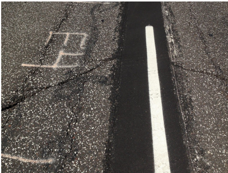
Figure 3.79 Pothole E-4 (28 Days after Patching).
