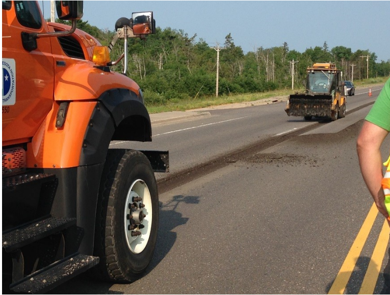
Figure B11: Mill and Fill Step 2.
