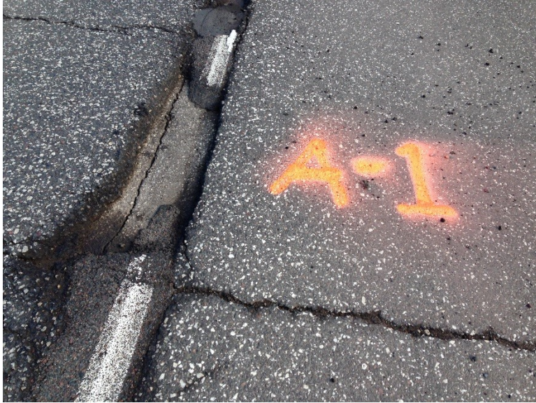
Figure 3.1 Pothole A-1 prior to Patching (After Cleaning).
