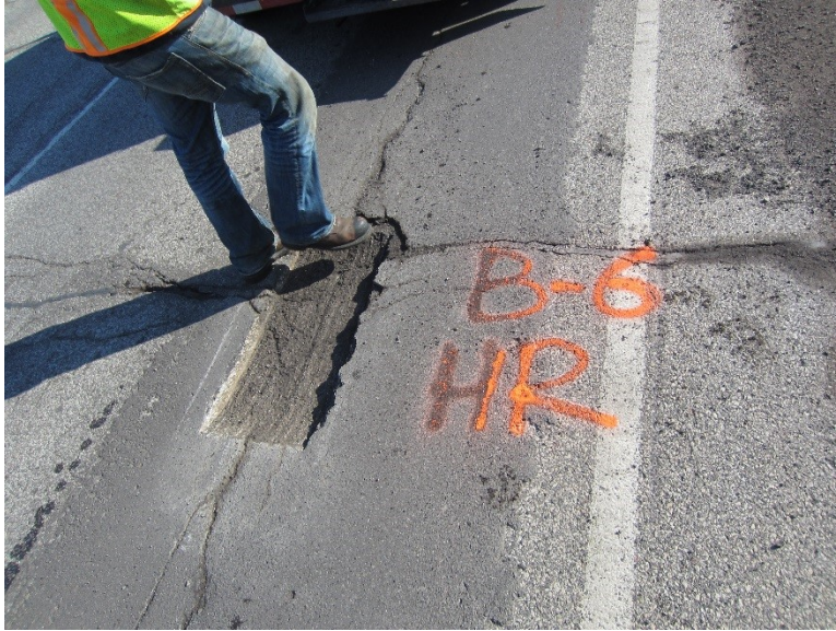
Figure 3.31 Pothole B-6 after Milling.
