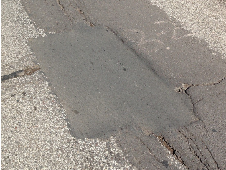
Figure 3.40 Pothole B-5 (146 Days after Patching).
