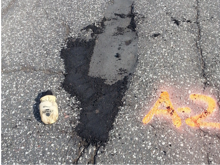
Figure 3.7 Pothole A-2 after Patching.
