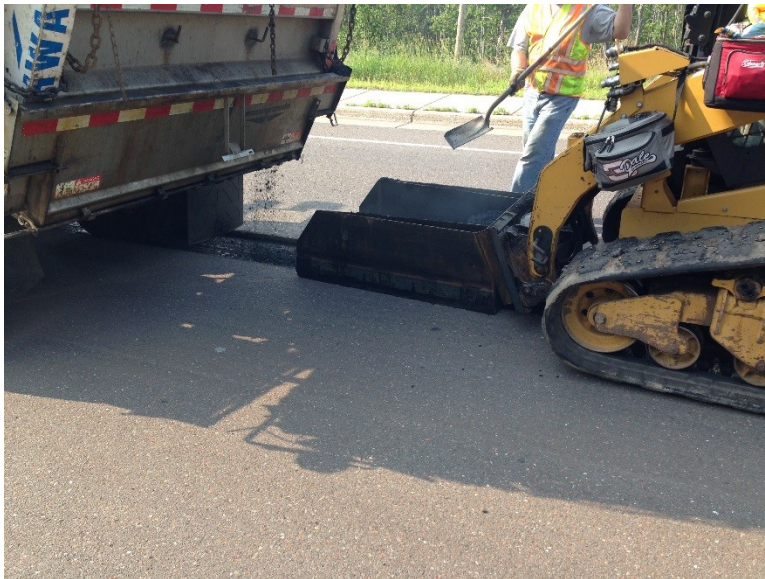
Figure B12: Mill and Fill Step 3.
