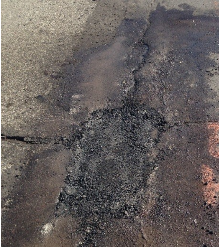
Figure 3.45 Pothole B-6 immediately after Patching.
