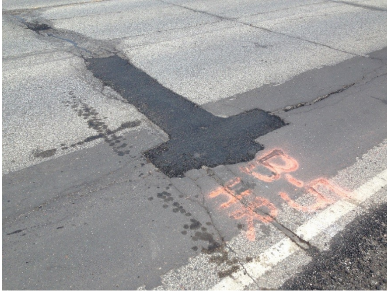
Figure 3.43 Pothole B-5 (3 Days after Patching).
