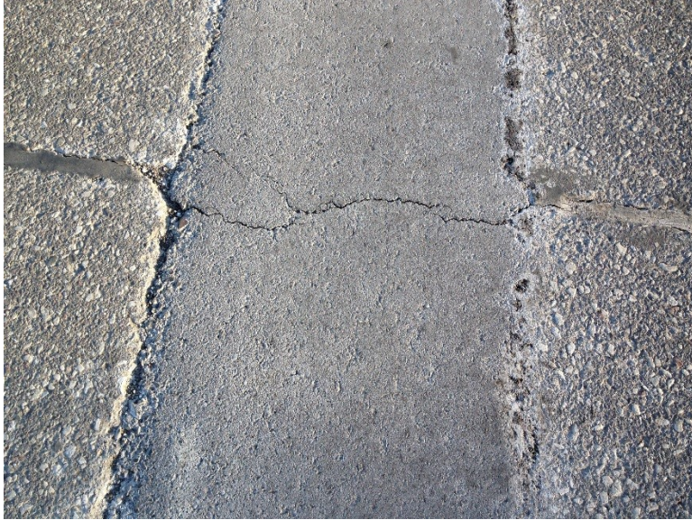
Figure 3.82 Cracking of Pothole E-3 (119 Days after Installation).
