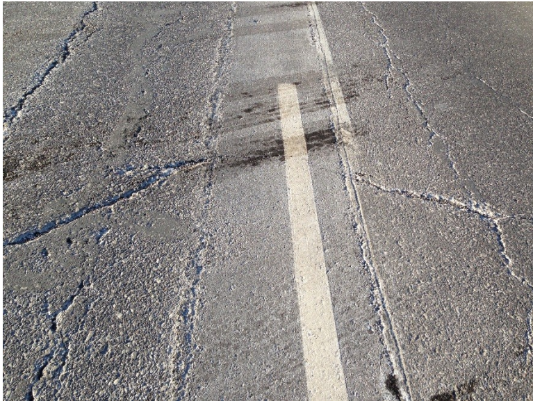
Figure 3.83 Pothole E-4 (119 Days after Installation).
