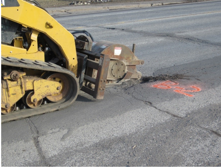
Figure B1: Cold Mix Step 1.
