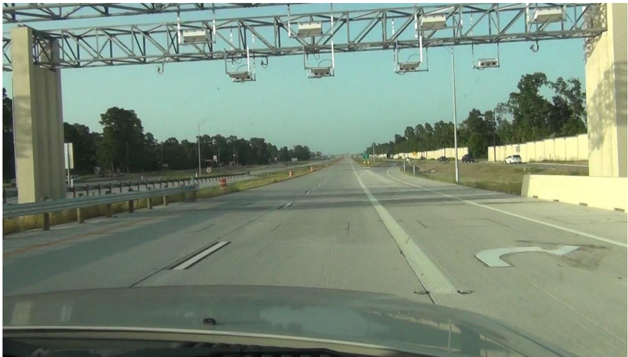
Figure 160. TTI Field Photo of Eastbound Main Lanes West of Spring Trails Ridge at TTI Location 3A, SH 99 Segment G.
