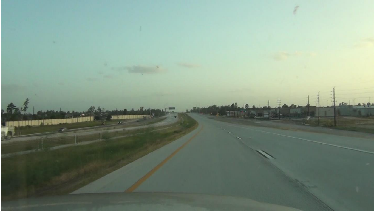
Figure 167. TTI Field Photo of Westbound Main Lanes East of Rayford Rd Underpass at TTI Location 5, SH 99 Segment G.
