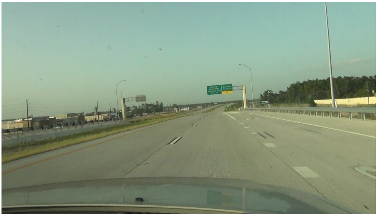
Figure 166. TTI Field Photo of Eastbound Main Lanes East of Rayford Rd Underpass at TTI Location 5, SH 99 Segment G.
