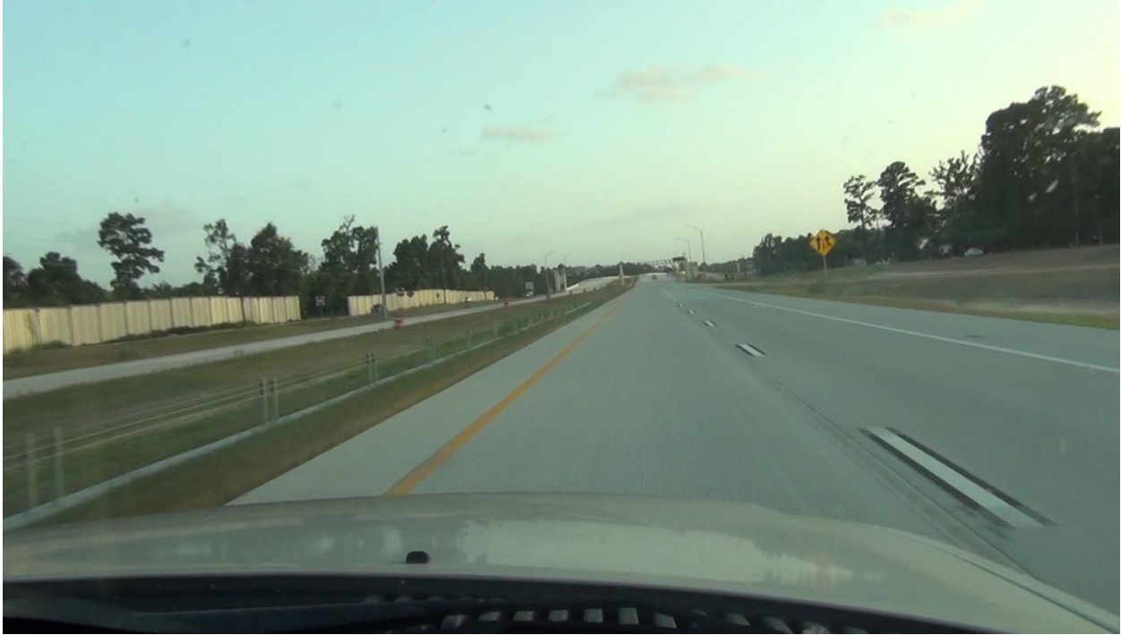
Figure 161. TTI Field Photo of Westbound Main Lanes West of Spring Trails Ridge at TTI Location 3A, SH 99 Segment G.
