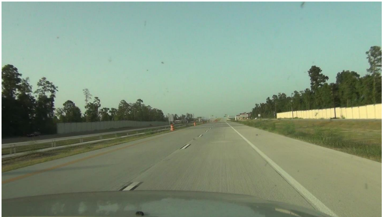
Figure 163. TTI Field Photo of Eastbound Main Lanes at Discovery Creek Underpass at TTI Location 4, SH 99 Segment G.
