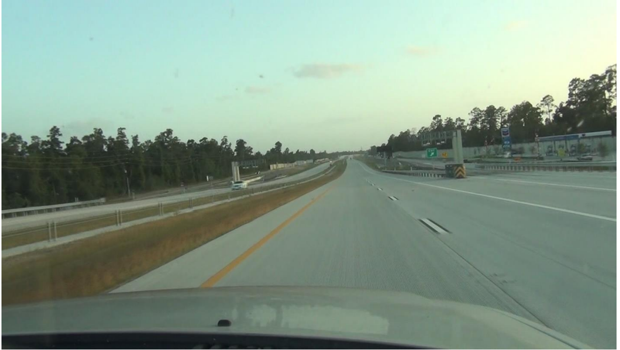
Figure 164. TTI Field Photo of Westbound Main Lanes at Discovery Creek Underpass at TTI Location 4, SH 99 Segment G.
