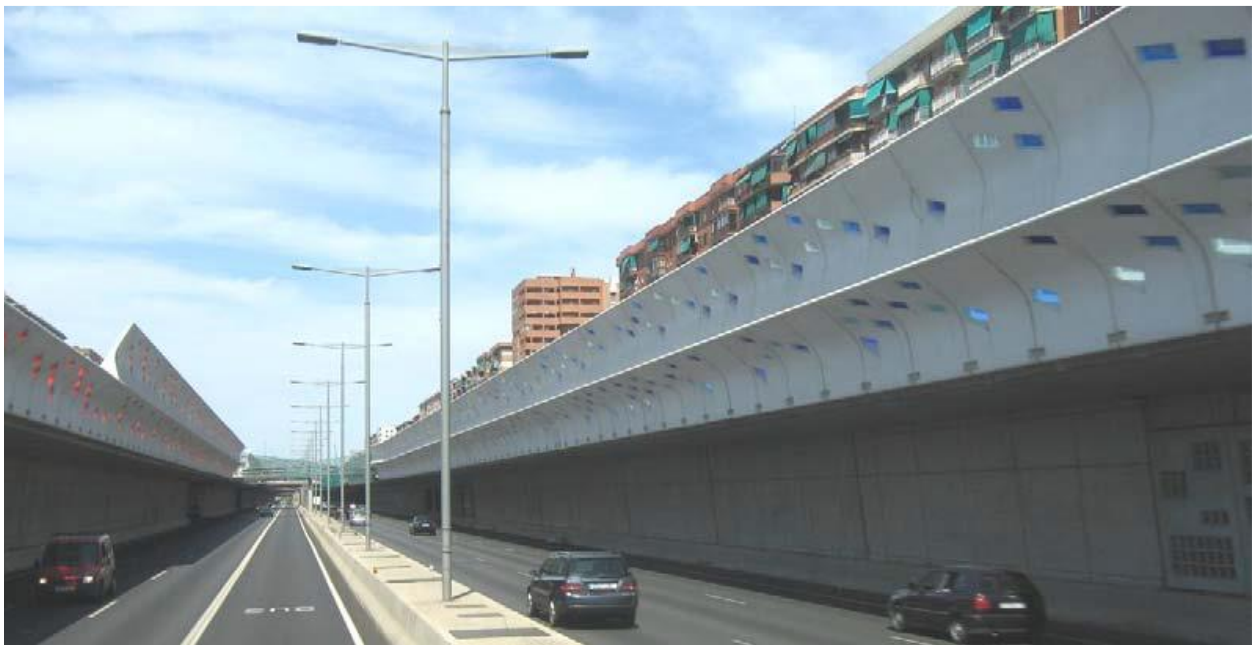
Figure 28. Steel Noise Barrier in Vienna, Austria, Bending over the Highway to Increase the Noise Reduction.
