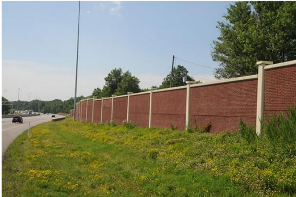
Figure 20. Brick Sound Wall.
