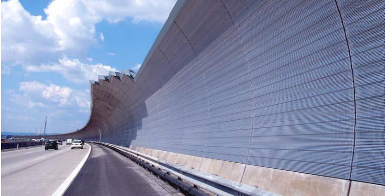
Figure 28. Steel Noise Barrier in Vienna, Austria, Bending over the Highway to Increase the Noise Reduction.
