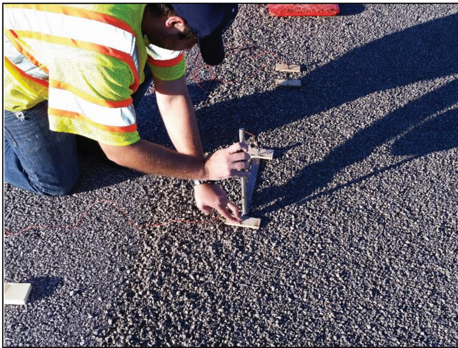
Figure 4.25 Tapping steel rod probes.
