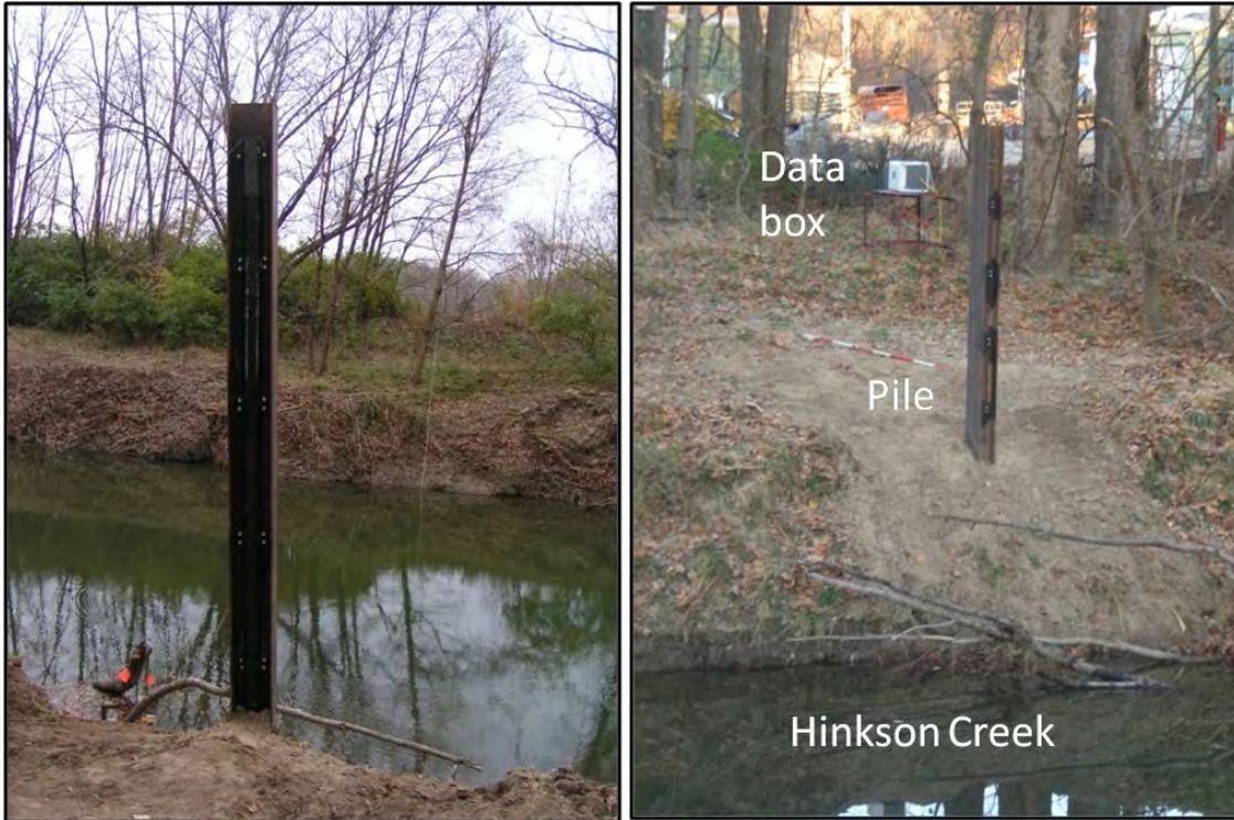
Figure 5.13. Photograph of the test pile installation at Hinkson Creek.
