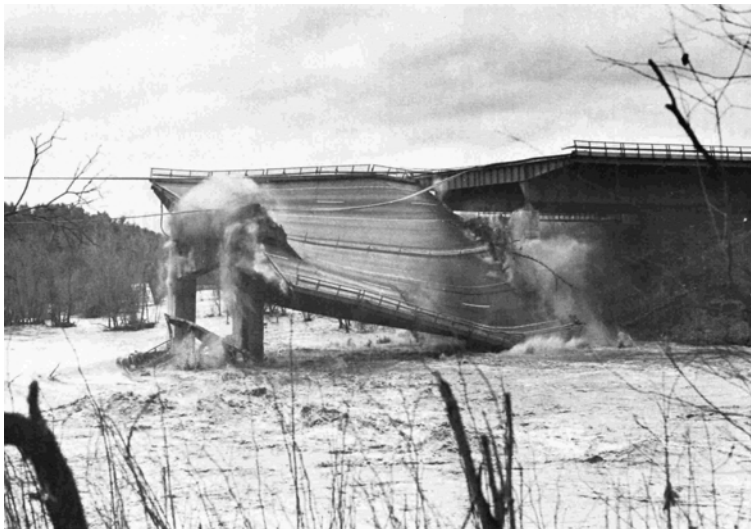
Figure 2.1. Photograph of the Skoharie Creek Bridge collapse, 1987.
