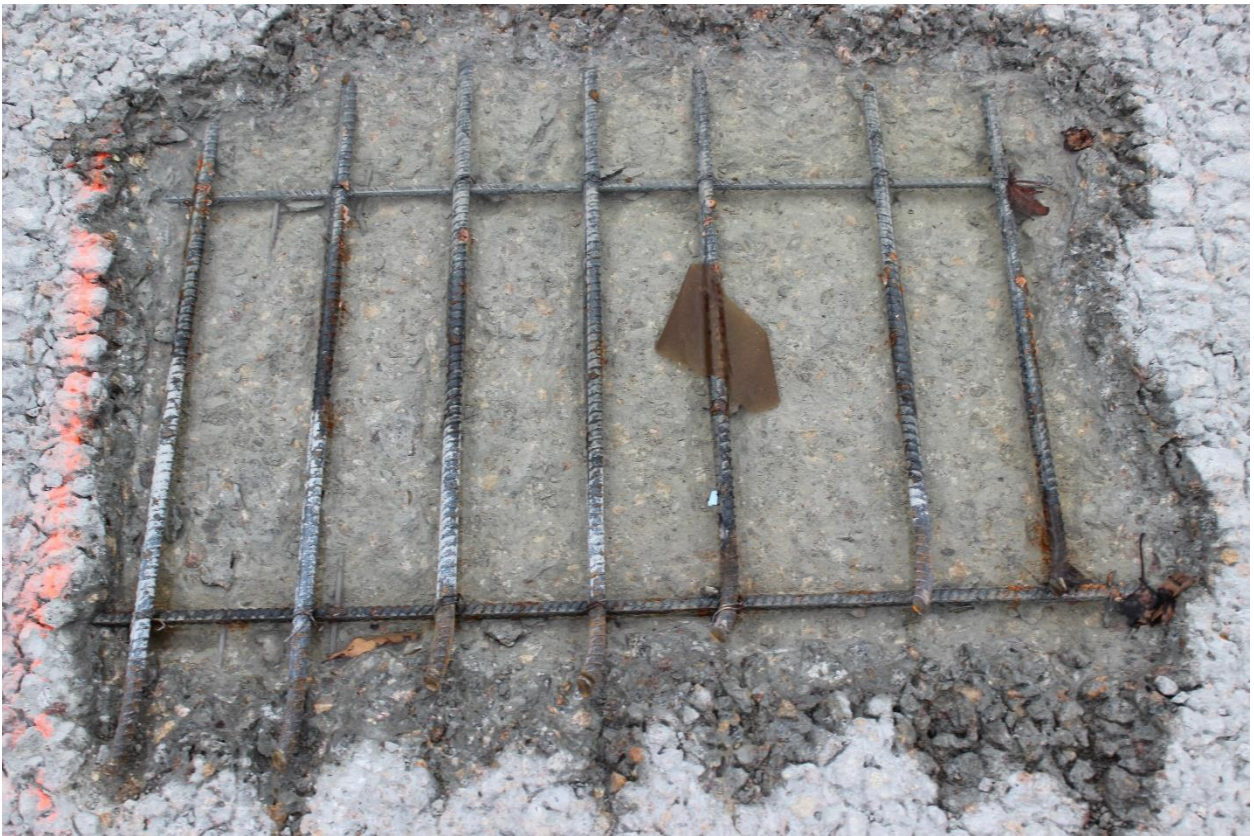
Figure 44: representative area with residual water and debris.
