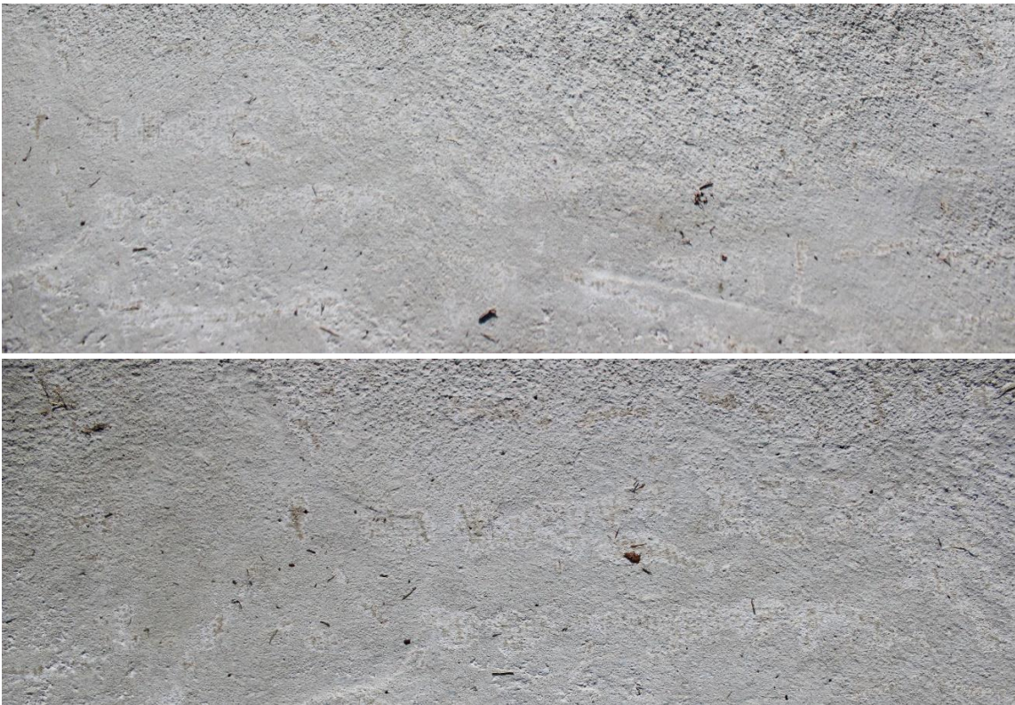
Figure 37: Photograph of fiber reinforced LMC overlays after 21 days.
