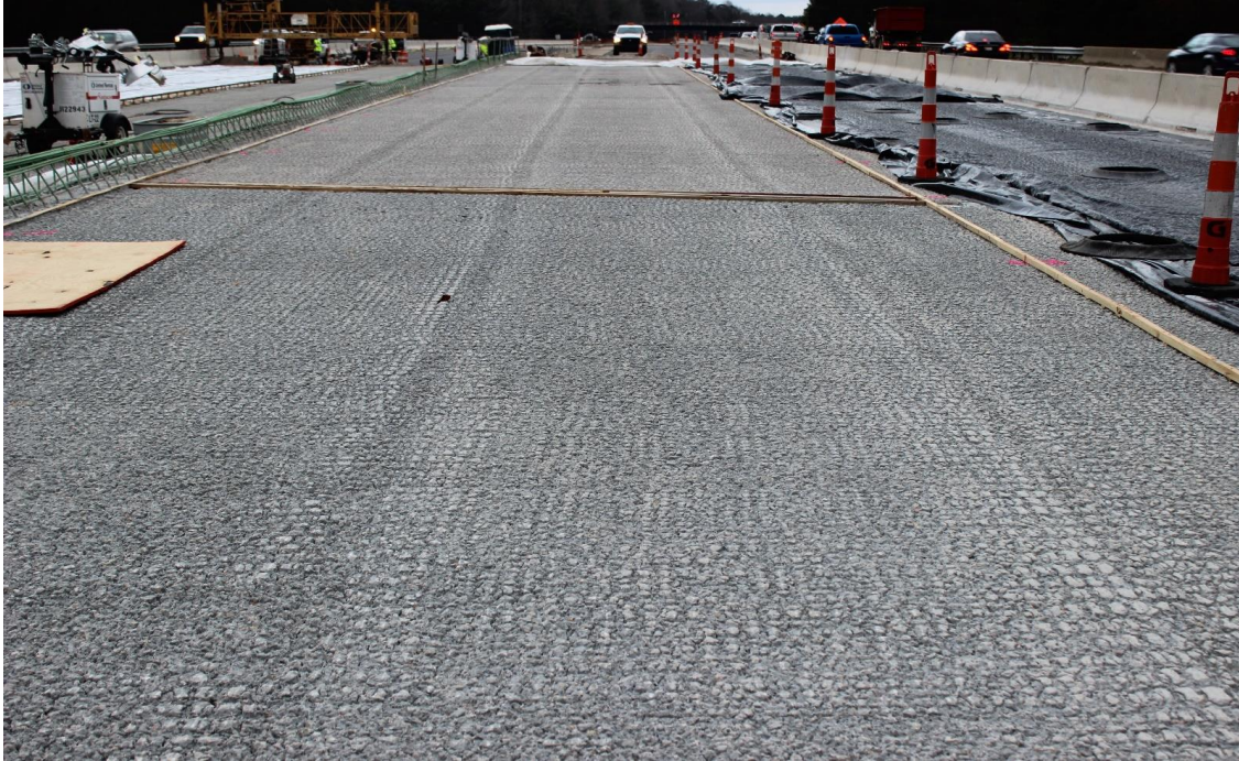
Figure 40: Photograph of the north end of the scarified bridge.
