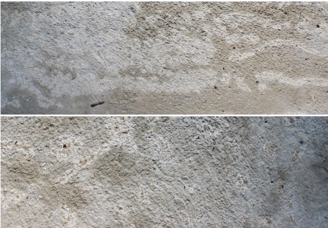
Figure 35: Photograph of fiber reinforced LMC overlays after 14 days.
