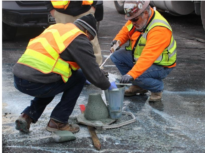
Figure 46: Photograph of slump test performed on-site.
