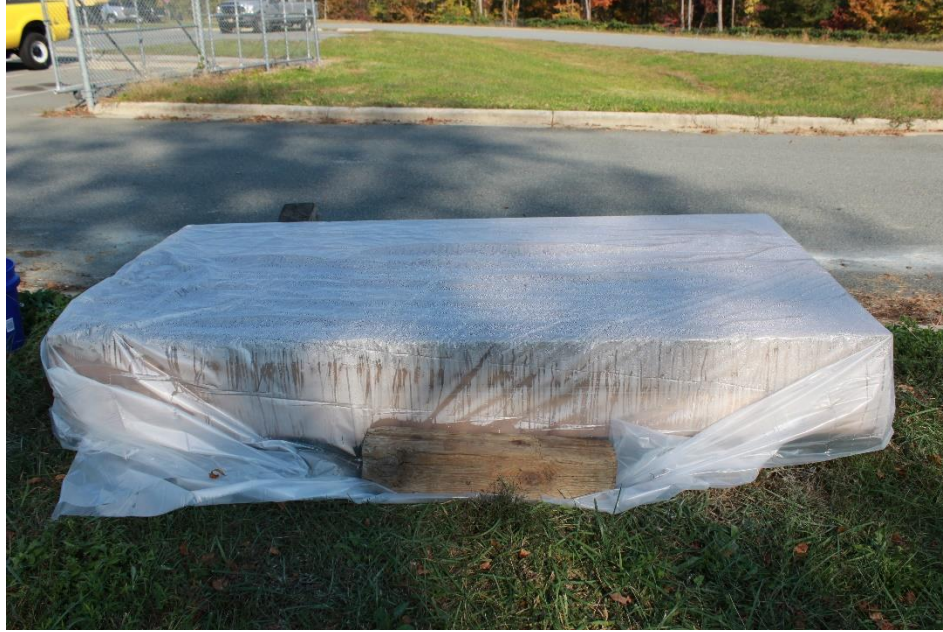
Figure 11: Photograph of curing condition: saturated burlap under 4-mil plastic sheet.
