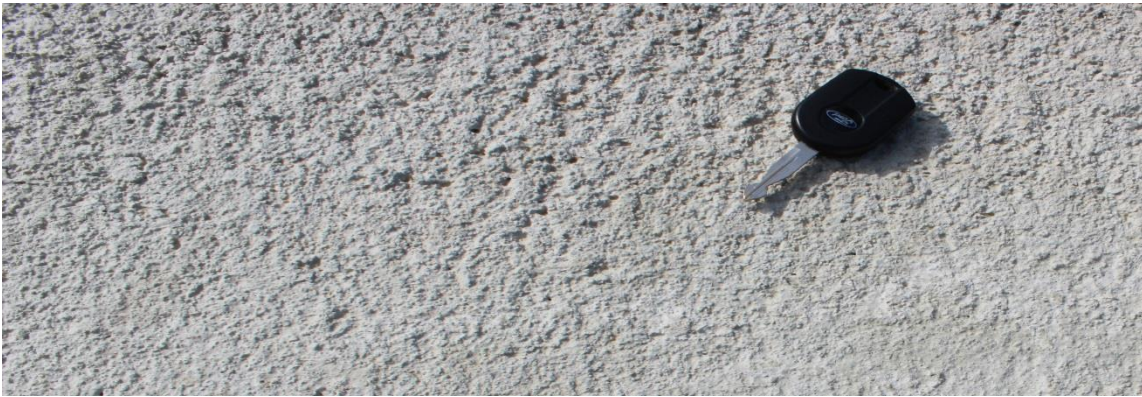
Figure 38: Photograph of LMC overlays after 165 days.
