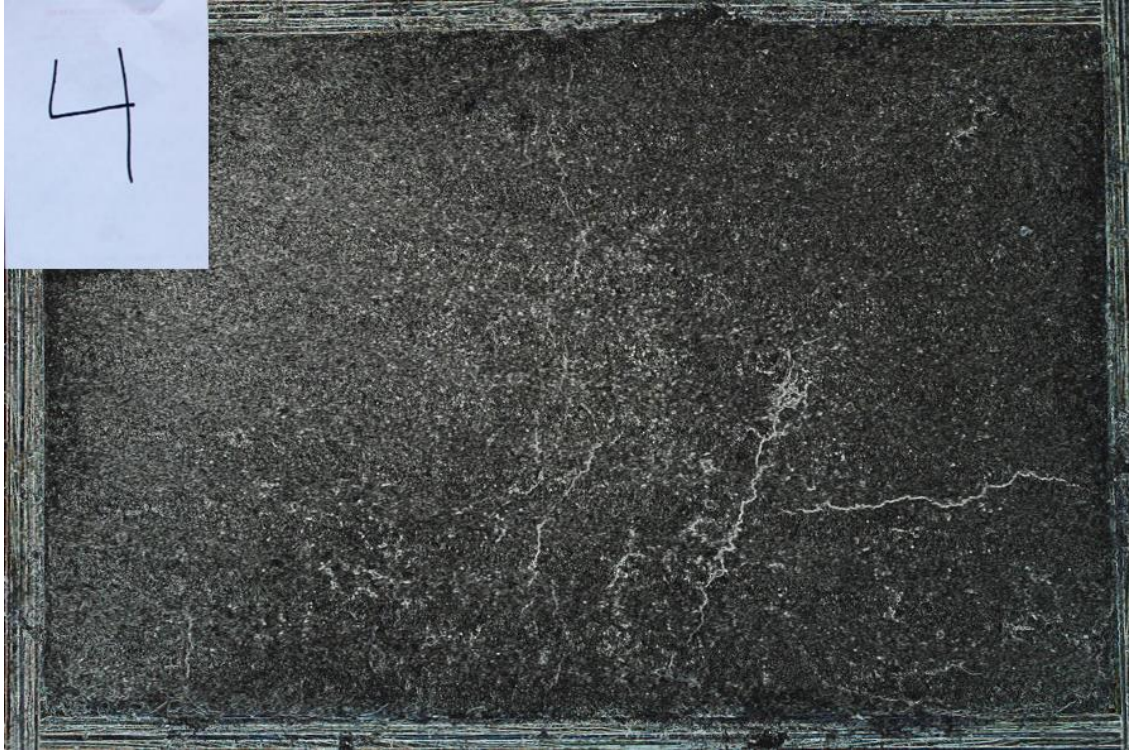
Figure 19: Photograph of the specimen with shallow surface cracking due over-finishing (same specimen as Figure 18d).
