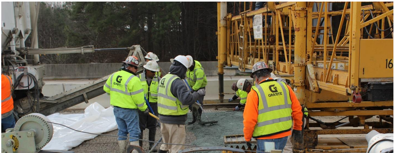
Figure 48: Auger-roller mechanical system used in the Gorman Street LMC bridge overlay.
