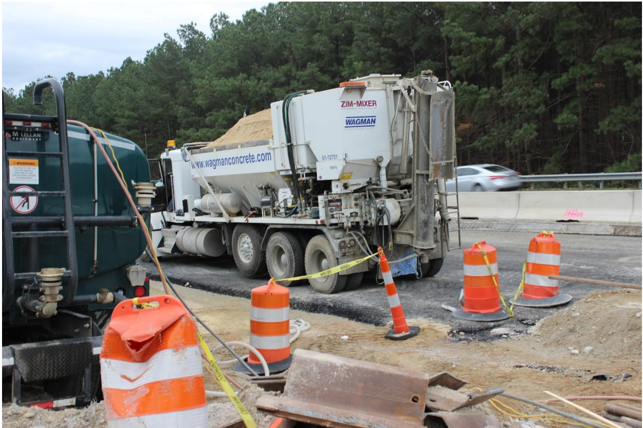
Figure 45: Volumetric mixer used for field batching of LMC mixes
