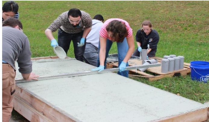
Figure 10: Photograph of the LMC overlay during the casting.
