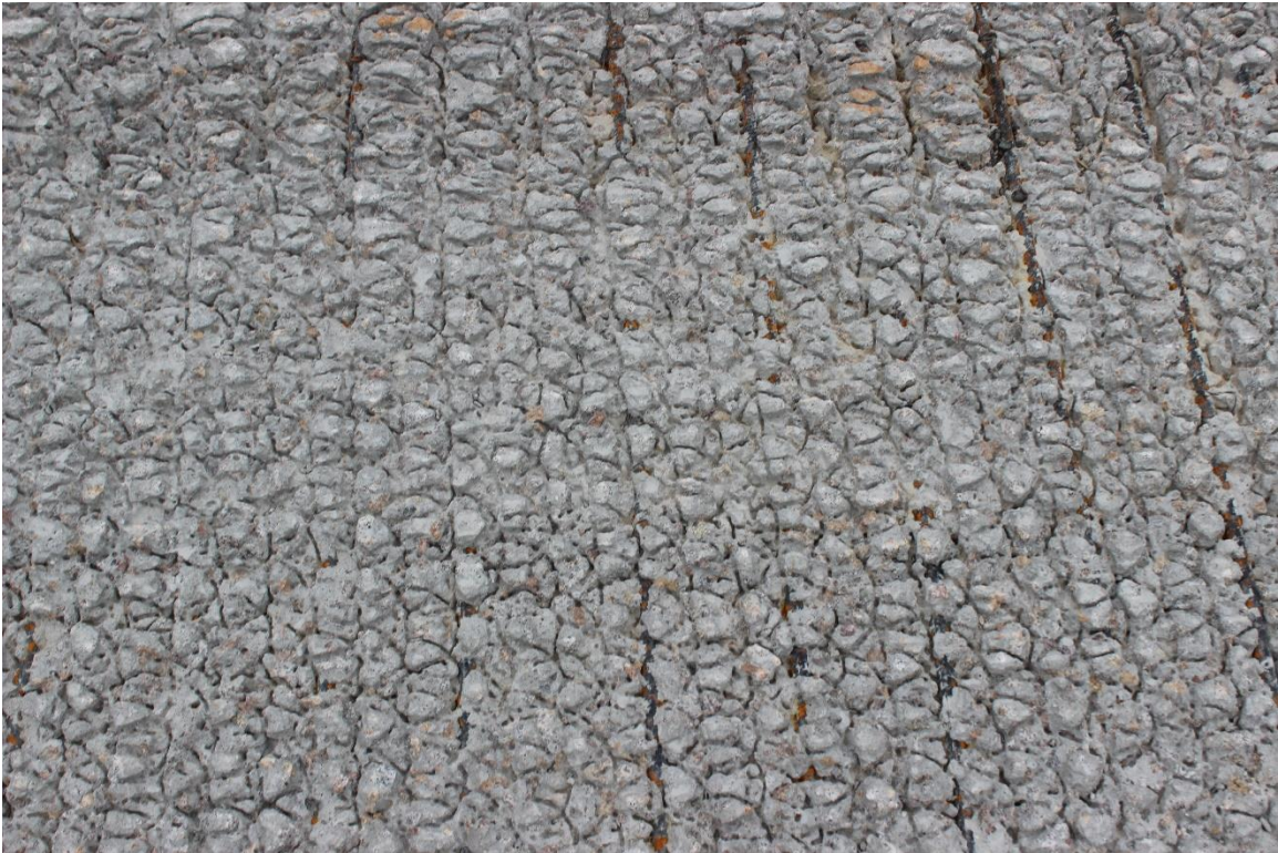
Figure 41: Photograph of scarification directly above the bridge mid span.
