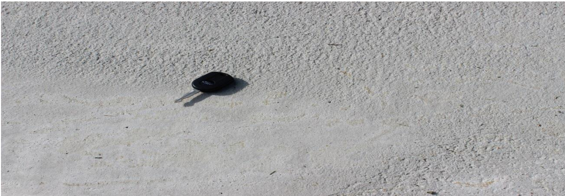
Figure 38: Photograph of LMC overlays after 165 days.
