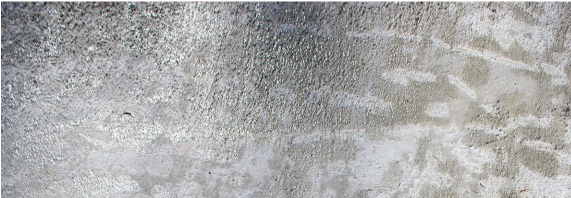
Figure 31: Photograph of fiber reinforced LMC overlays after 3 days.
