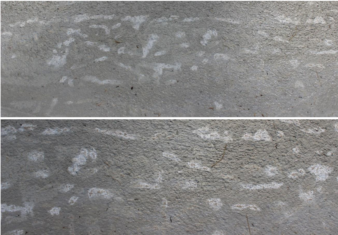
Figure 33: Photograph of fiber reinforced LMC overlays after 7 days.
