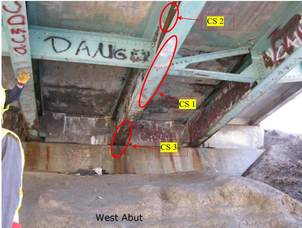
Figure 5.8 Bridge with multiple condition states
