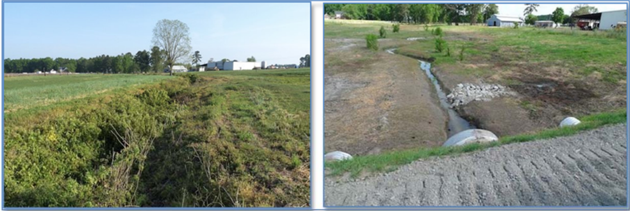
Figure 12 Rose branch before and after construction of wetlands.
