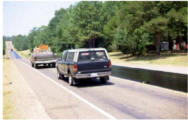
Pilot vehicle guides traffic through construction site.
