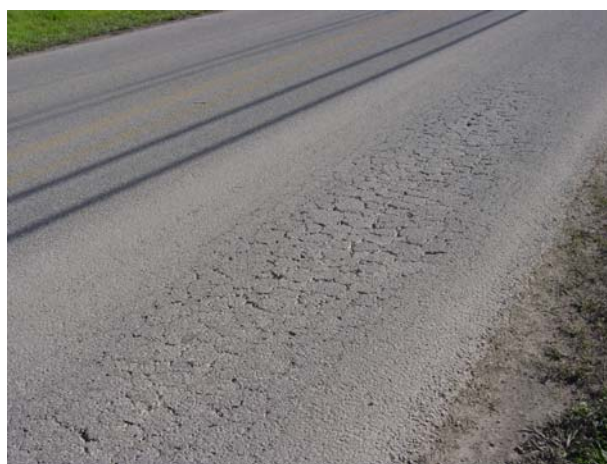
Fatigue Cracking
