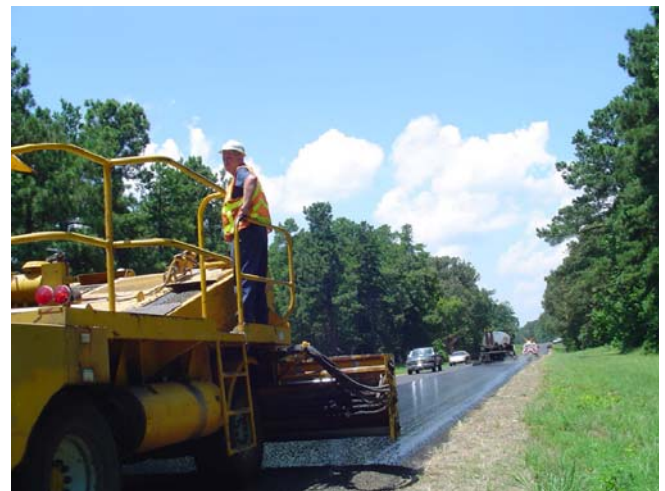
Seal Coat Application
