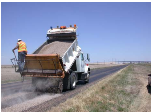
Applying Small-Size Aggregate to Treat a Bleeding Chip Seal (TRB 09-0659 pg. 9)
