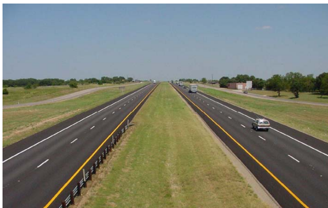
Microsurfaced pavement
