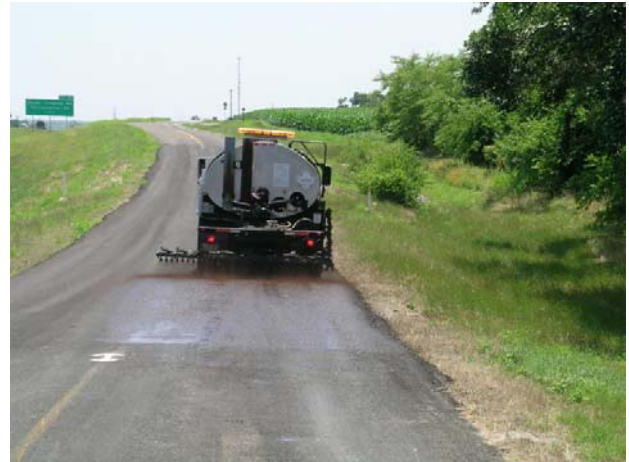
Fresh patches should be fog sealed prior to seal coat application.
