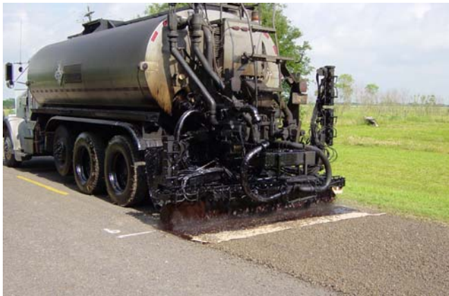
Seal Coat Application
