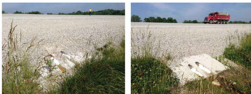
Figure 8.1 Drainage pipes observed on the new US-231 near Purdue Airport.
