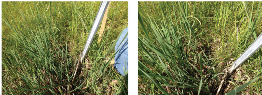
Figure 7.5 Buried K-drains on the side slope of I-65N.
