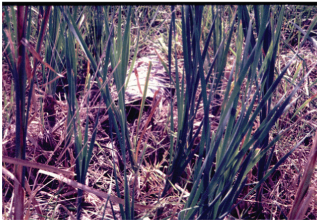
Figure 3.4 Typical hidden outlet pipe (14).
