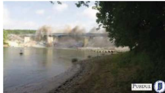
(f) Bridge after implosion
