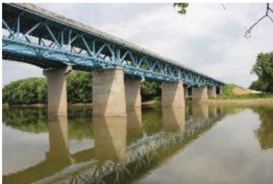
(b) Bridge before demolition
