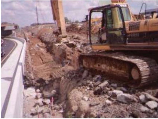
(a) Earthwork for placement of pad
