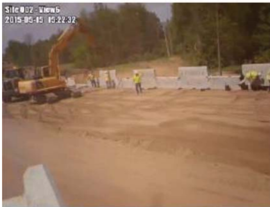
(e) Placing next row of panels
