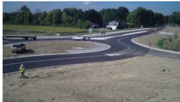
(c) Roundabout construction complete
