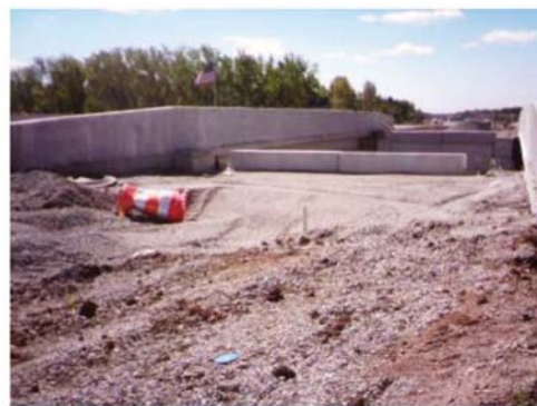
(h) Bridge is complete 8/31/15
