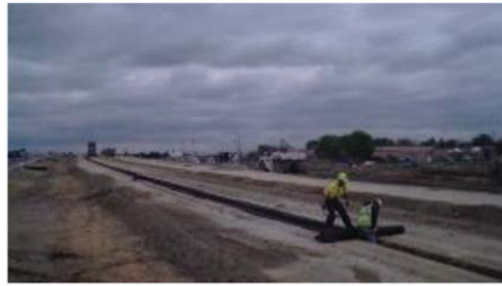
(b) Placing geotextile fabric
