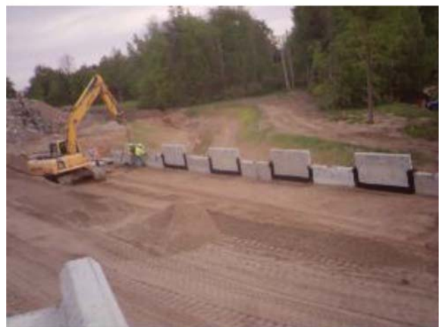
(c) Fabric is then placed horizontally along the seam
