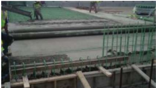
(e) 6/9/15 4:22 PM – Concrete is placed
