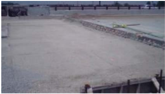
(a) 6/2/15 – Bridge abutment formwork
