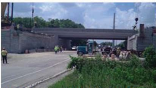
(g) 12:56 PM – Beam is detached from crane
