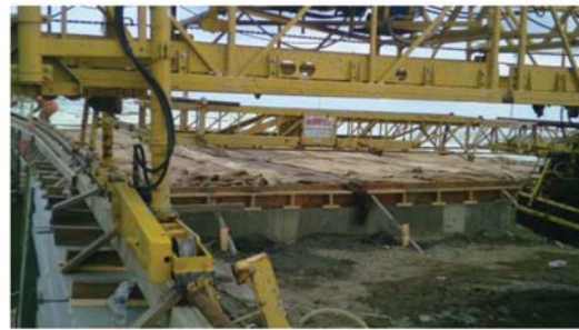
(f) 7/2/15 – Concrete curing under burlap
