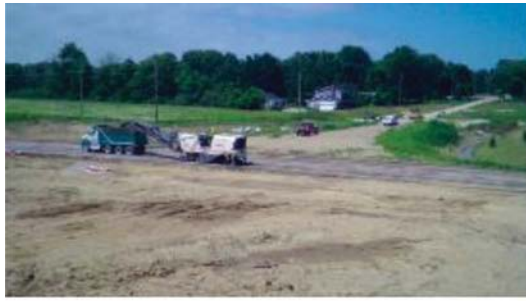
(a) 6/23/15 – Demolition of old roadway
