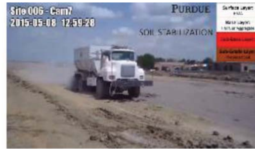
(b) 5/8/15 – Lime soil stabilization
