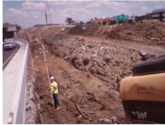
(b) Check level for pad
