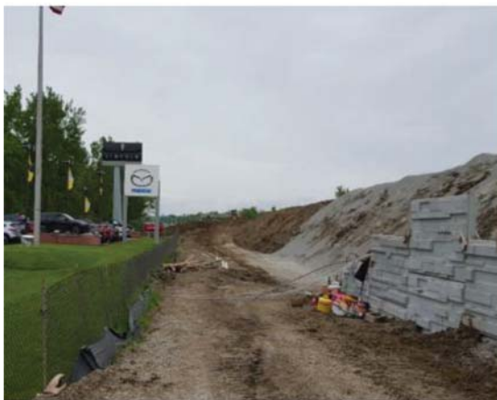
(b) Bridge during construction
