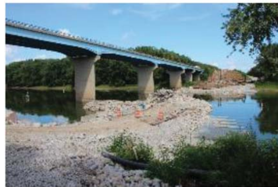
(c) Bridge fully removed
