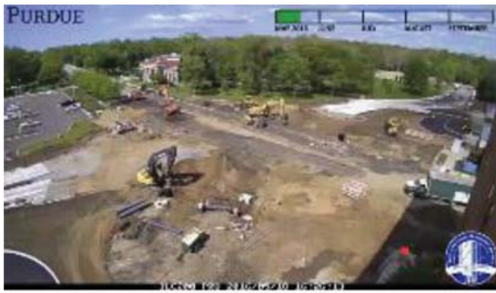
(a) Demolish original intersection 5/18/16
