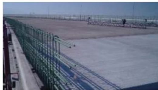
(h) 10/12/15 – Steel layout for concrete guardrail
