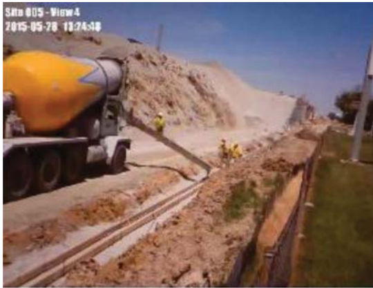
(a) Placing concrete for leveling pad
