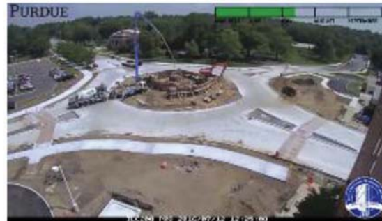
(f) Place concrete at roundabout center 7/12/16
