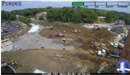
(c) Place aggregate base for concrete pavement 6/1/16
