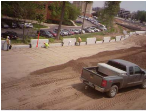
(a) Connecting straps to panels
