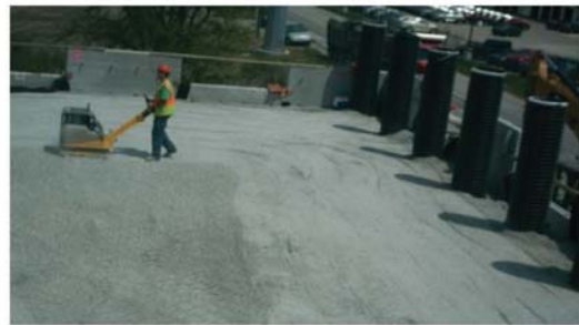
(f) 2:42 PM – Soil compaction
