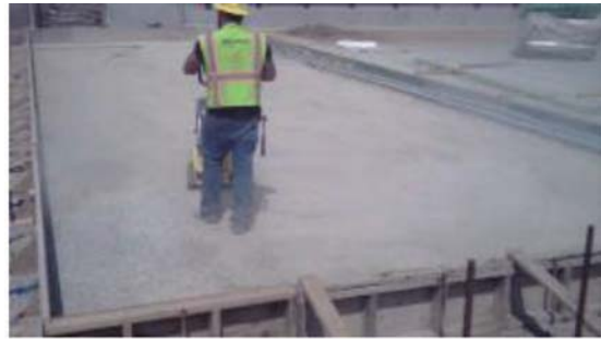
(b) 6/4/15 11:22 AM – Compaction of soil
