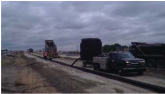
(c) Underdrain pipe placement
