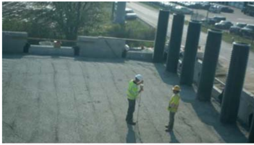
(a) 9:28 AM – Compaction test
