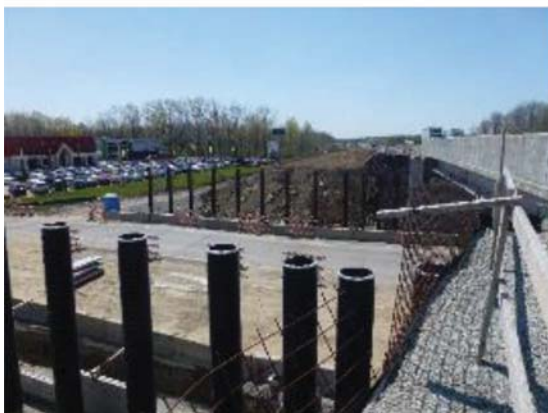
(b) Bridge during construction
