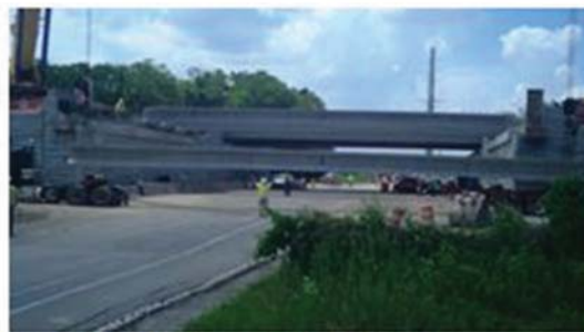
(d) 12:50 PM – Beam is lifted off truck
