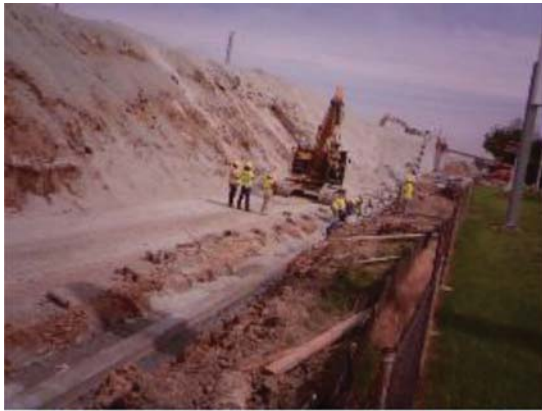
(a) Bare leveling pad – start panel placing
