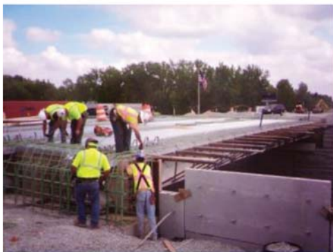
(e) Bridge decking operations 6/16/15
