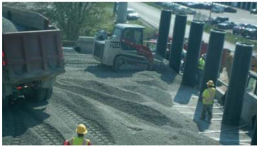
(c) 10:51 AM – Structural backfill placement
