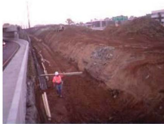
(f) Remove forms and place panels
