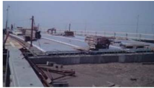
(b) 6/9/15 – Safety railing installed
