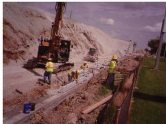
(f) Level half-size panels with wooden shims
