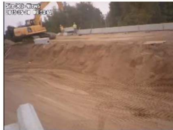
(f) Placing finishing coping
