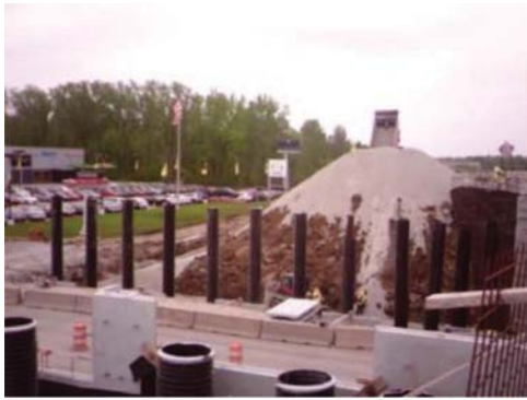
(a) Stockpiling structural backfill 5/14/15
