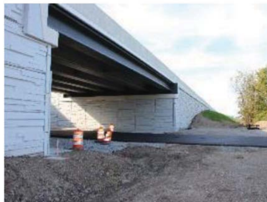
(c) Bridge construction complete
