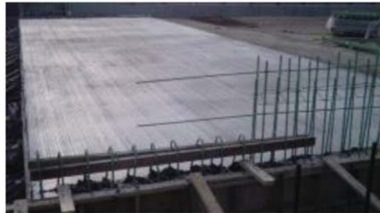
(f) 6/9/15 6:06 PM – Concrete begins to cure
