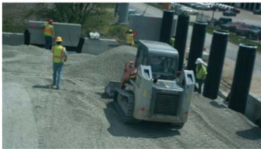
(e) 12:51 PM – Panel placement, soil placement
