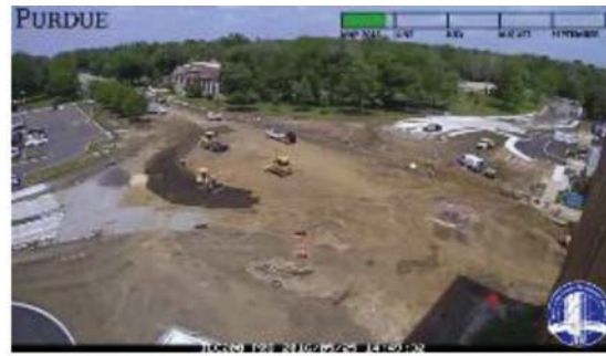
(b) Place subgrade soil for concrete pavement 5/25/16
