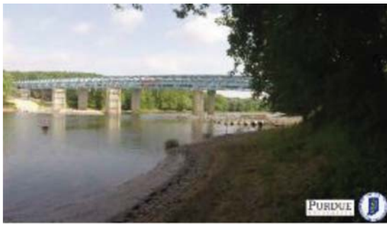
(a) Bridge before charges are set
