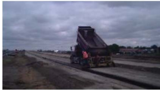
(d) Aggregate placed to facilitate drainage
