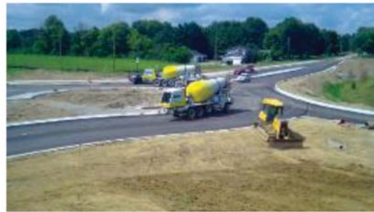
(f) 8/26/15 – Place concrete curbs and truck apron
