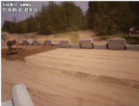
(c) Soil placement – beginning of a lift
