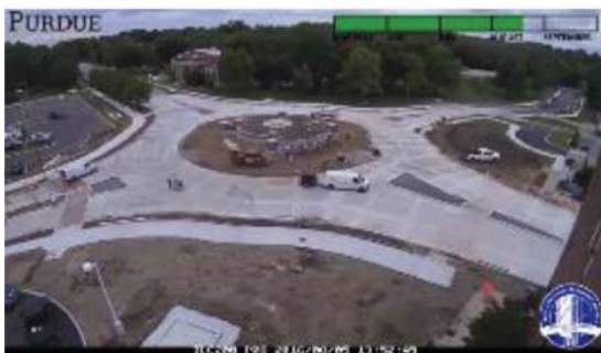
(g) Saw-cut pavement panel joints 8/5/16
