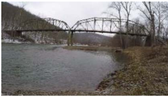
(a) Bridge before charges are set
