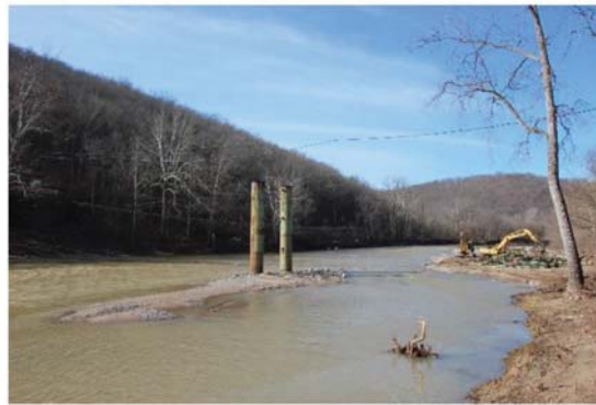
(c) Bridge during removal
