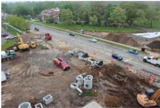
(b) Roundabout during construction
