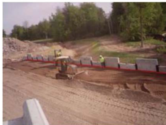
(f) Soil level after lift
