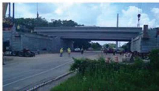
(f) 12:53 PM – Beam is lowered into place
