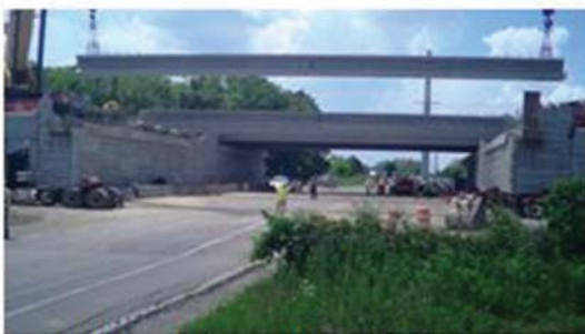
(e) 12:51 PM – Beam is lifted above bridge
