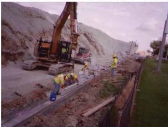
(e) First row of panels contains two distinct panel types
