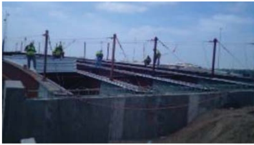
(a) 6/4/15 – Bridge deck pan installation
