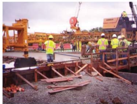
(f) Place concrete deck on bridge 7/9/15
