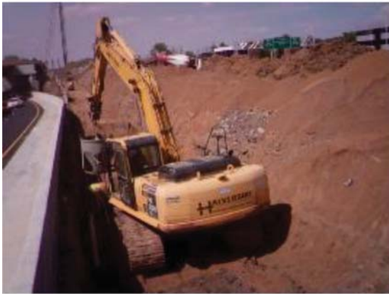
(e) Place leveling pad concrete
