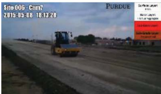
(e) 5/8/15 6:13 PM – Soil is compacted
