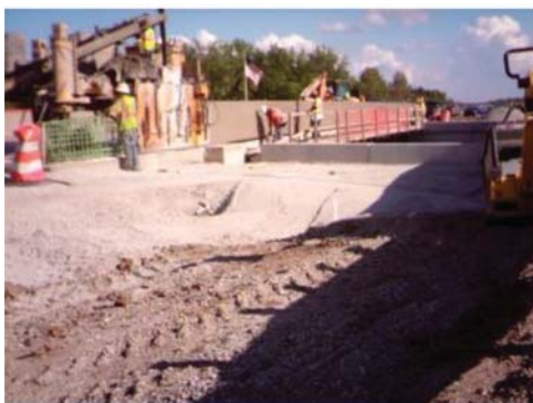
(g) Slip-form concrete guardrails 8/11/15
