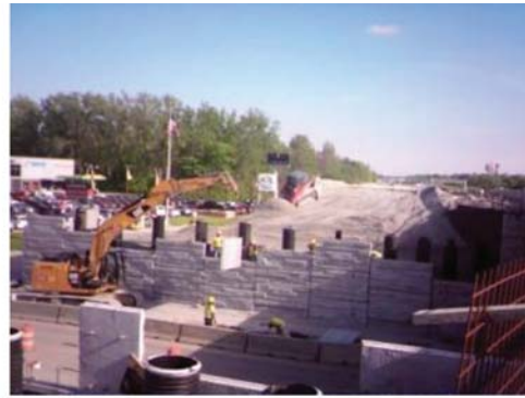
(b) Placing panels of MSE wall 5/19/15
