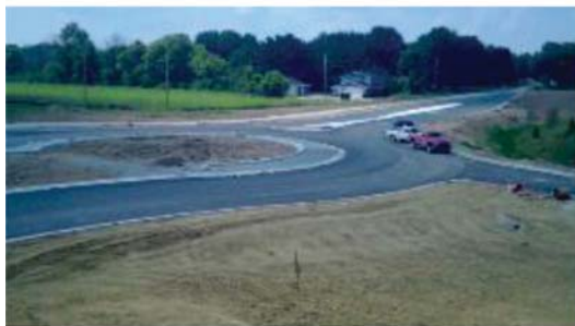
(g) 8/31/15 – Allow concrete to cure
