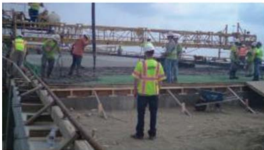
(e) 7/2/15 – Concrete is placed on bridge deck
