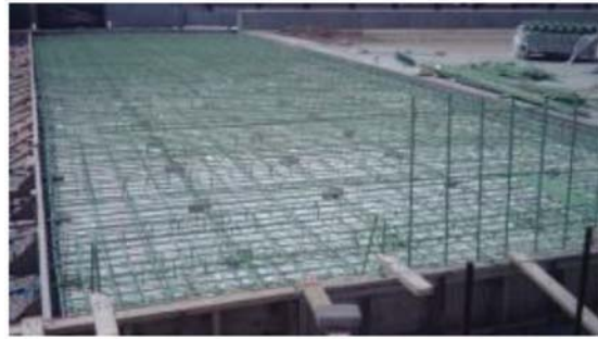
(d) 6/5/15 – Steel is placed for abutment
