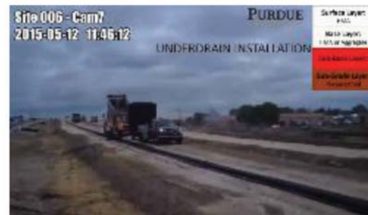
(f) 5/12/15 – Underdrain installation
