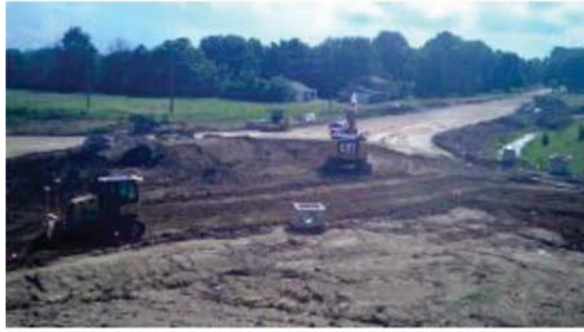
(c) 7/14/15 – Roundabout earthwork
