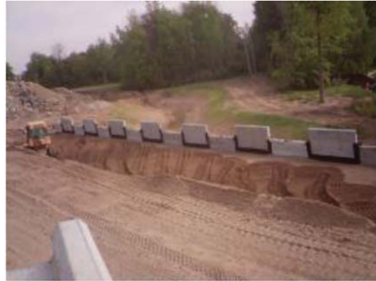
(b) Soil is pushed toward the panels
