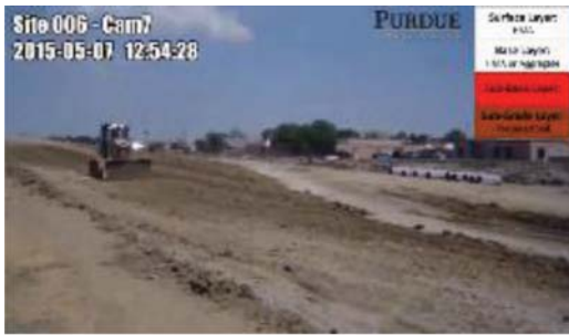
(a) 5/7/15 – Roadway Earthwork
