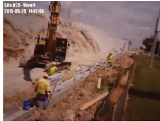
(b) Placing first row of panels
