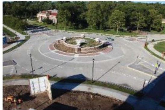
(c) Roundabout construction complete
