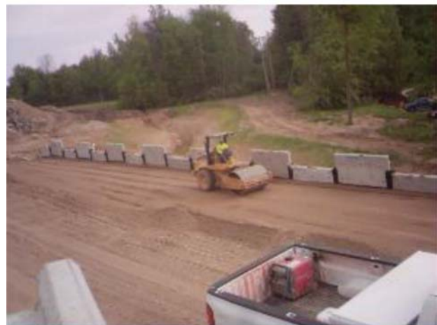
(b) Vibratory roller must make 5 passes over soil
