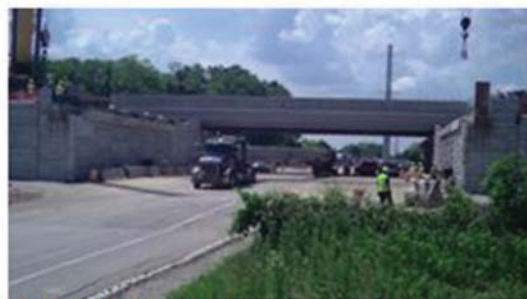
(h) 12:59 PM – Beam No. 9 arrives on site
