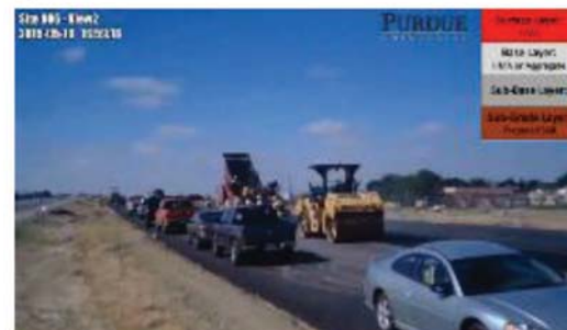
(h) 5/19/15 1:56 PM – Asphalt surface layer is applied
