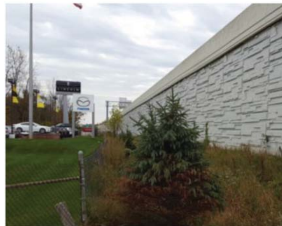
(c) Bridge construction complete
