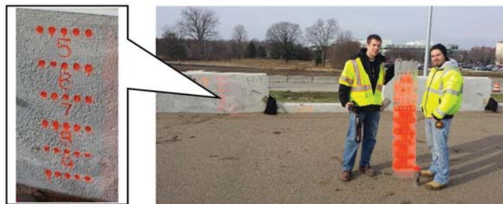
(g) MSE wall backfill lift thickness reference
