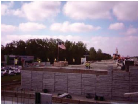
(c) Bridge beam support 6/2/15
