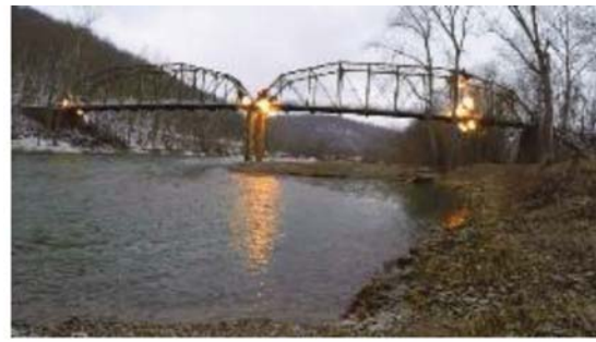
(b) Bridge during implosion
