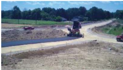
(e) 7/30/15 – Place asphalt base layer
