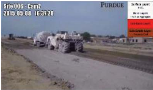
(c) 5/8/15 – Lime mixed into soil
