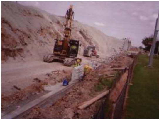
(c) Place on leveling pad and level vertically and horizontally
