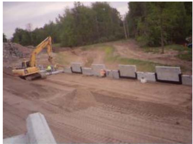
(a) Panel before joint covering fabric is placed
