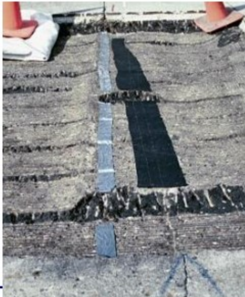
Figure E-2. Prevention of reflective cracking by localized debonding.
