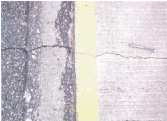
Figure E-1. Reflective cracking observed at MnROAD.
