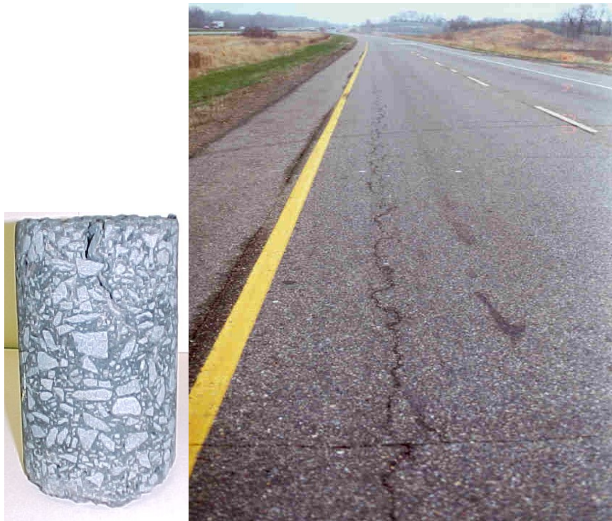
Figure E-3. Top-down longitudinal fatigue cracking at MnROAD.
