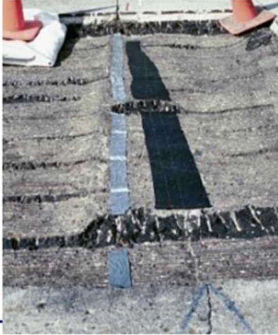
Figure 12. Prevention of reflective cracking by localized debonding.
