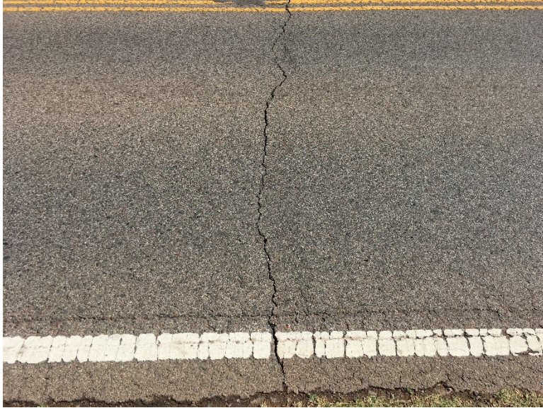
Figure 10. Transverse (thermal) cracking in an existing HMA pavement.
