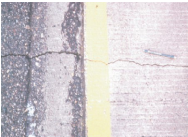
Figure 10. Transverse (thermal) cracking in an existing HMA pavement.
