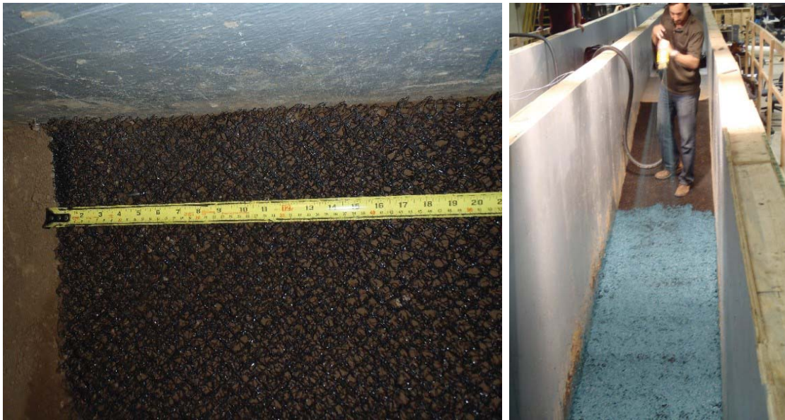
Figure 3.13. Photo on the left shows the turf reinforcement mat installed on the soil. Photo on the right shows the Fiber Reinforced Matrix being applied.
