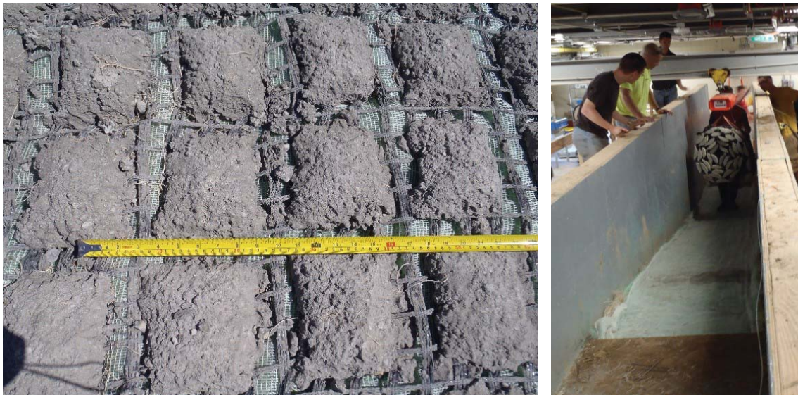
Figure 3.14. Photo on the left shows the concrete blocks and flexible geogrid underlain by the turf reinforcement mat. In the photo on the right, the turf reinforcement mat is overlaying the soil and the concrete blocks and flexible geogrid is being hoisted into place.
