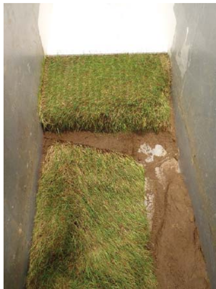
Figure 4.66. Looking upstream at shoulder to slope transition after the geogrid has been removed. Most of the transition is still intact while the areas where there was a seam between the rolled out pieces of sod allowed water to penetrate and erode the slope surface under the sod which was being partly held in place by the geogrid and landscaping staples.
