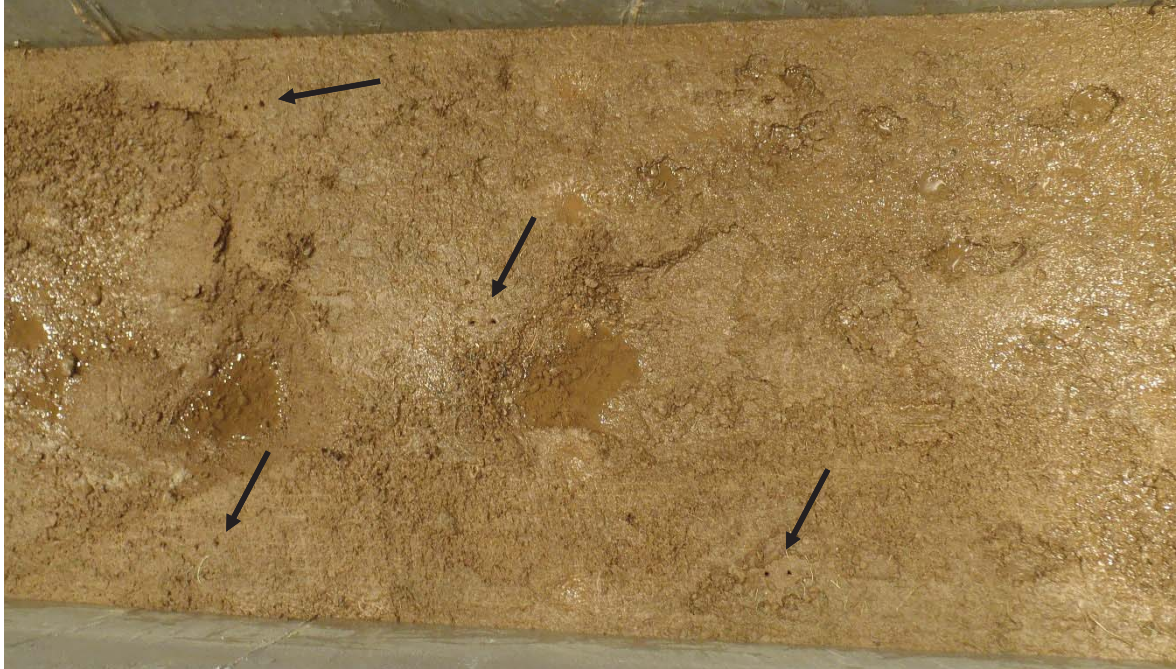
Figure 6.1. View from above of the bare soil after the ECB was removed post-testing, 6H:1V slope. Note the indicated holes where the staples were holding down the stabilization material. Flow was from right to left.
