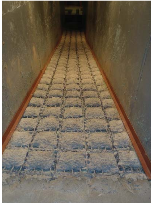
Figure 4.98. View from shoulder after Flexamat ® Plus installation and before testing.
