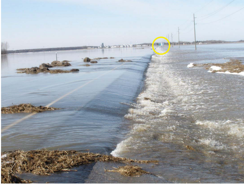
Figure 1.4. Overtopping event on MN TH1 near Oslo, Minnesota, March 21, 2010. “TH 1 at Jct 220 near Oslo 20100321”. Note road signs in yellow circle. Photo by JT Anderson, MnDOT
