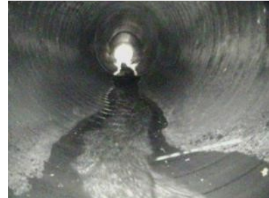
Figure 8 – Inspection video for culvert ID 36918
