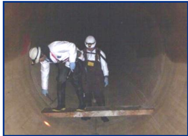
Figure 5.3 – Hammer Sound Testing
