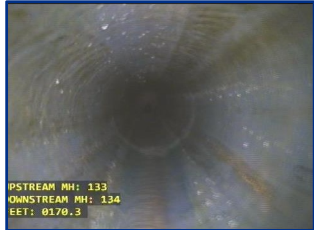
Figure 5.7 – Video Inspection of a Cured-in-Place Pipe Liner
