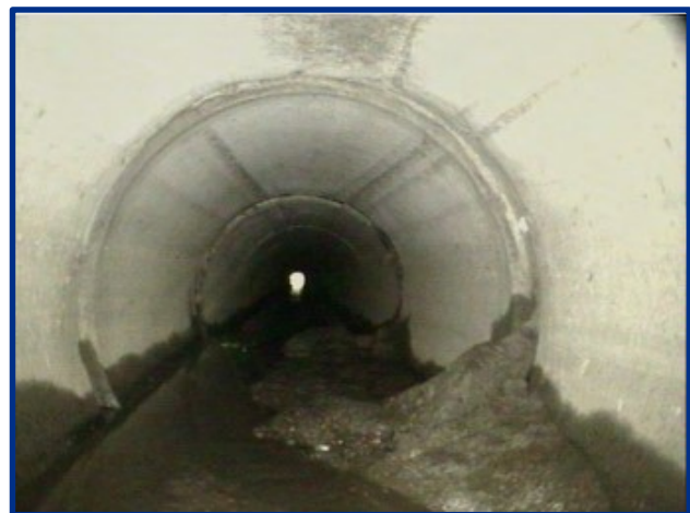
Figure 3.6 – Image Capture from CCTV Camera Inspection
