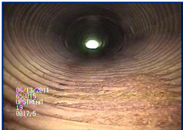
Figure 1.2 – Video Inspection Video Snapshot
