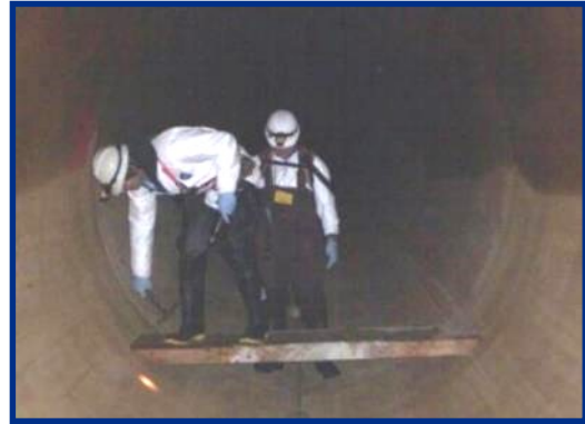
Figure 3.5 – Hammer Sound Testing
