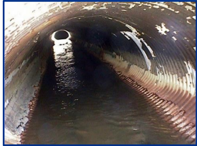
Figure 5.6 – CCTV Image Distortion
