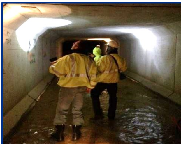
Figure 3.2 – Person Entry Inspection of a Rectangular Culvert
