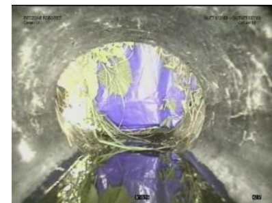
Figure 6 – A tarp was hung at the culvert’s outlet to control camera lighting.
