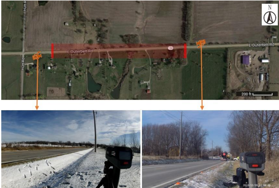
Figure 2.2.2 Field Settings on MO 150 Highway Work Zone (Google Maps 2017)
