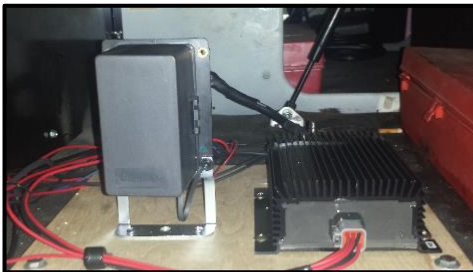
Figure 48. Power Supply and Converter Installation.
