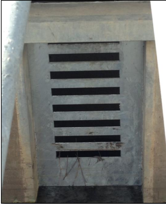
Figure 16. Actual installation of (left) water quality orifice plate, and (right) elliptical slot weir for the Northfield Detention Basin.
