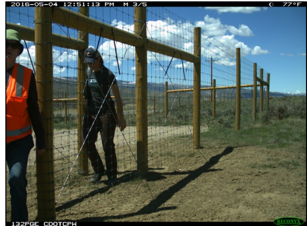
Figure 11. CDOT pedestrian walk-through gate design.
