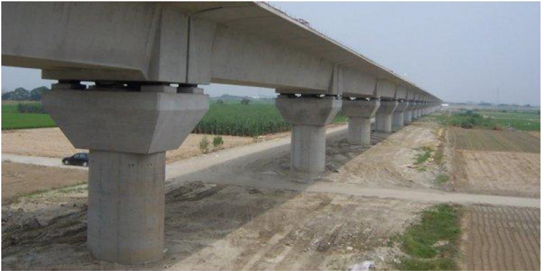
Figure 3-8: Taiwan High-Speed Rail Viaduct
