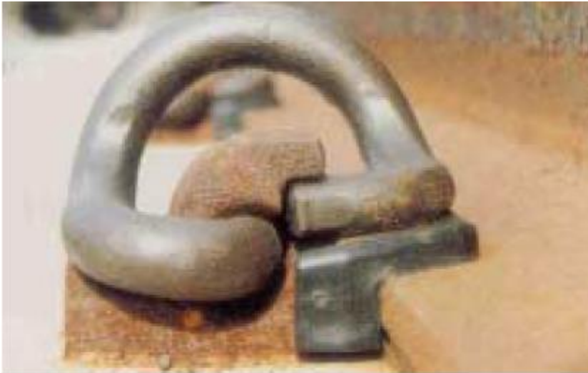
Figure 8.23: Pandrol fastening system
