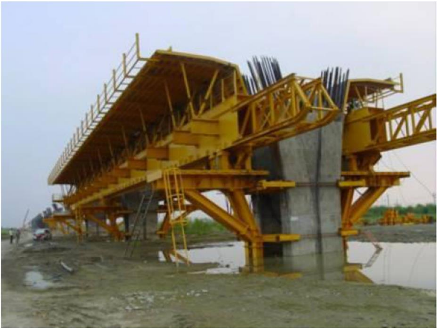
Figure 3-12: Example of Travelling Shoring System
