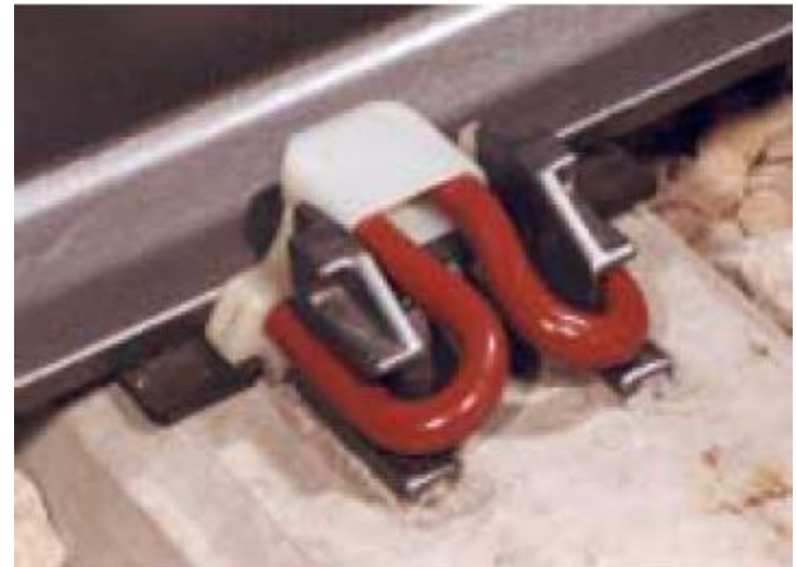
Figure 8.24: Pandrol Fastclip
