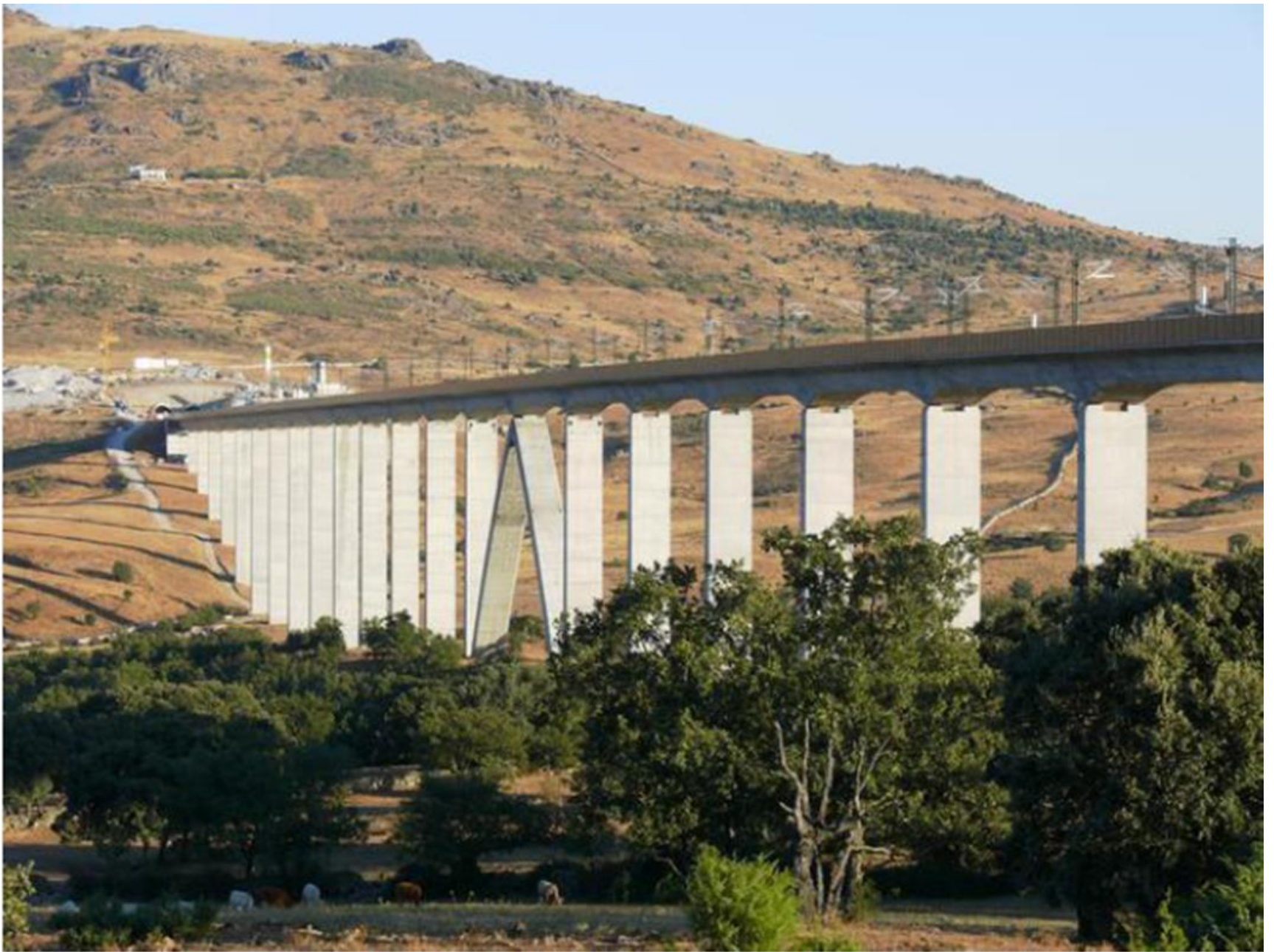
Figure 3-6: AVE High Speed Rail Viaduct
