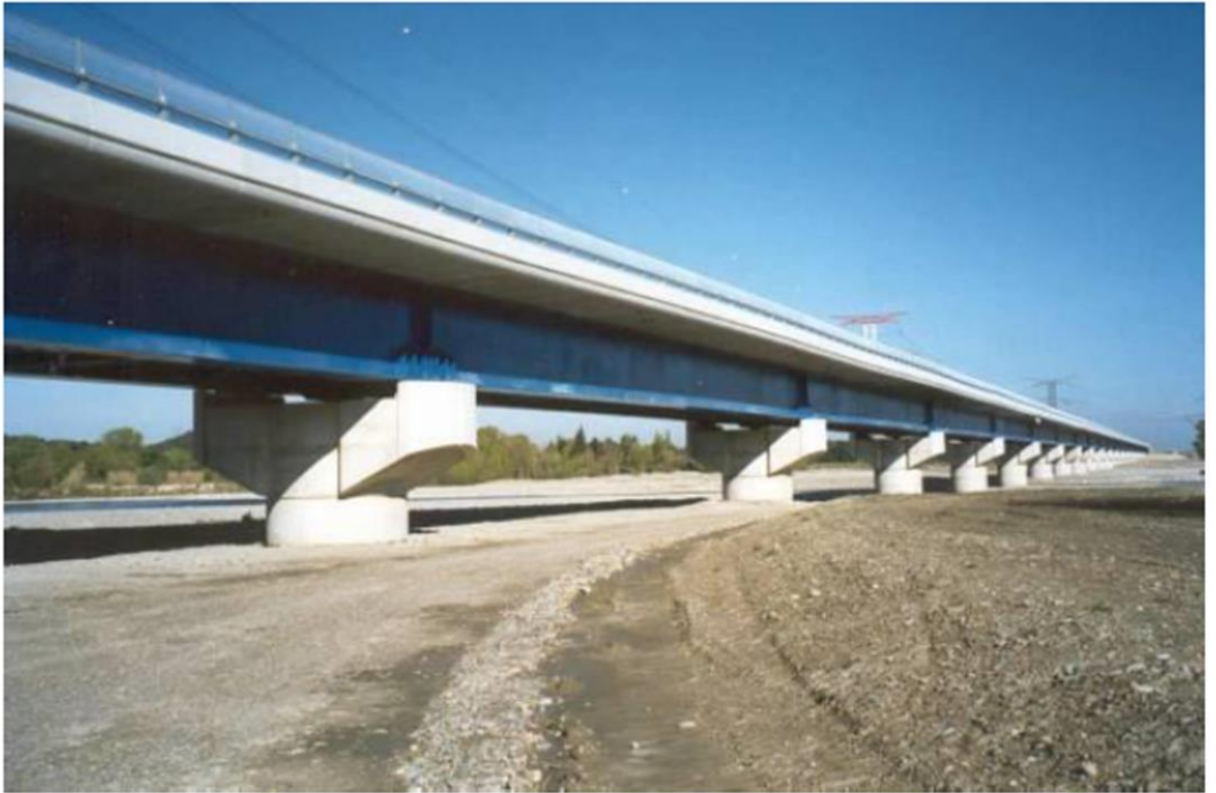
Figure 3-3: Cheval Blanc Viaduct, France
