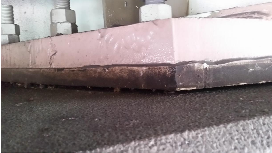
Figure 6-18: Bearing 7 of Abutment 2 partial uplift from substructure
