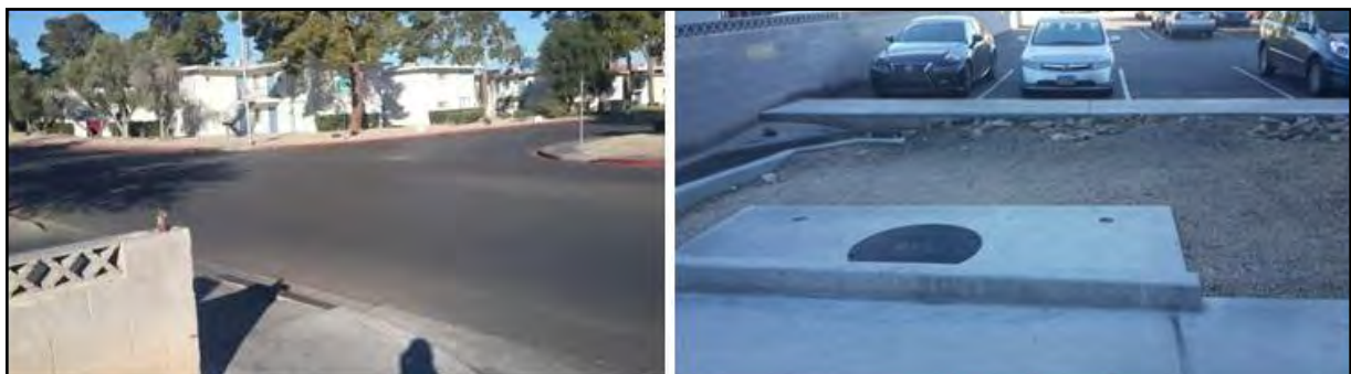
Claymont Street and Cottage Grove Avenue
