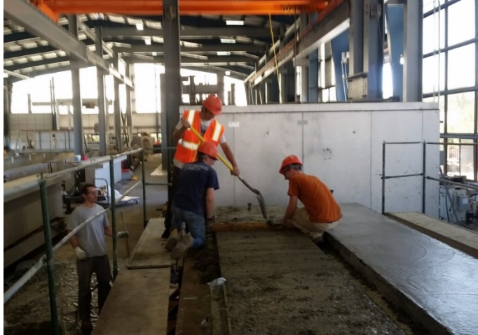
Figure 3.14: Concrete placement process
