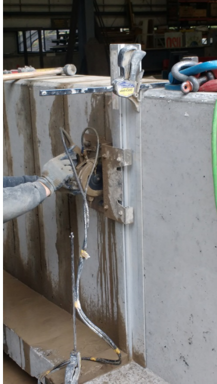
Figure 3.15: Groove cutting process with aluminum saw guide
