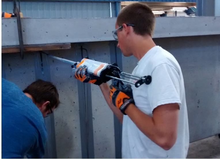
Figure 3.16: Titanium installation process
