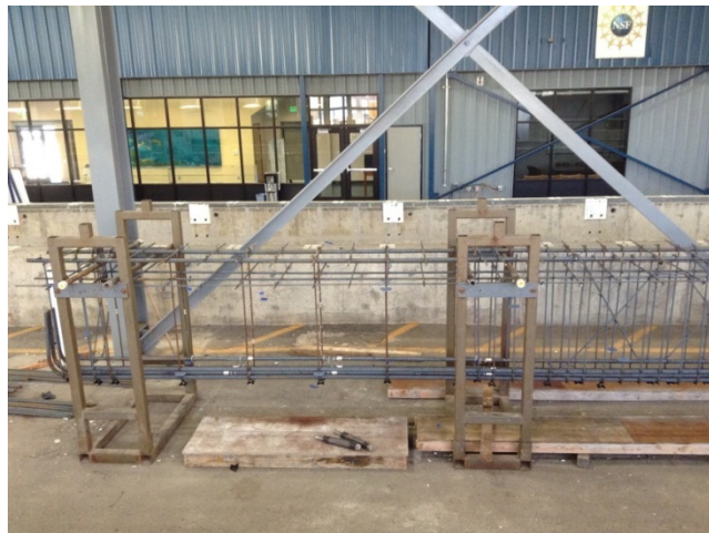
Figure 3.13: Cage construction process (test section on left)
