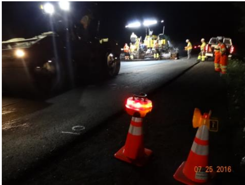
Figure 7.14: Intellicone® triggered 100 feet away from Paver
