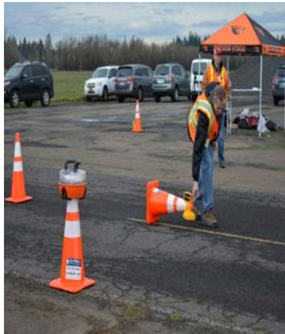
Figure 6.5: Intellicone® Activated Manually
