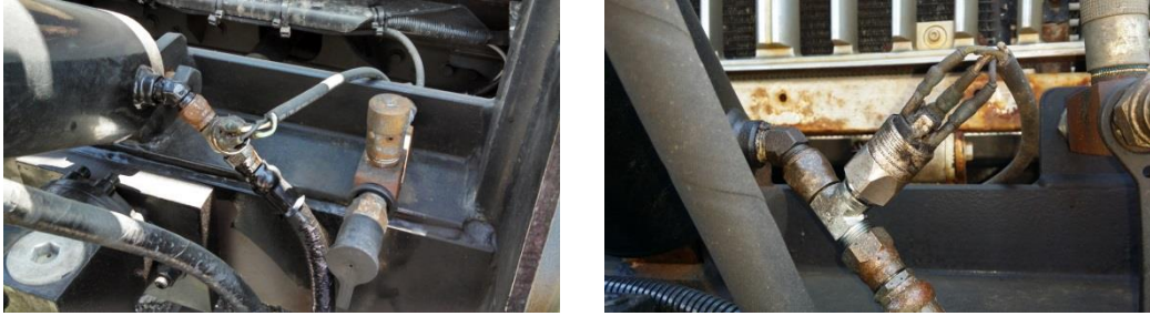
Figure A.15: Completed Installation of Hydraulic Pressure Sensor.
