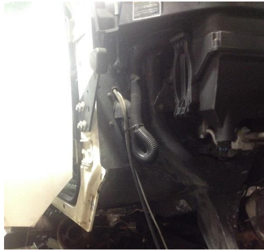
Figure A.11: Drilled hole through fire wall into cab.
