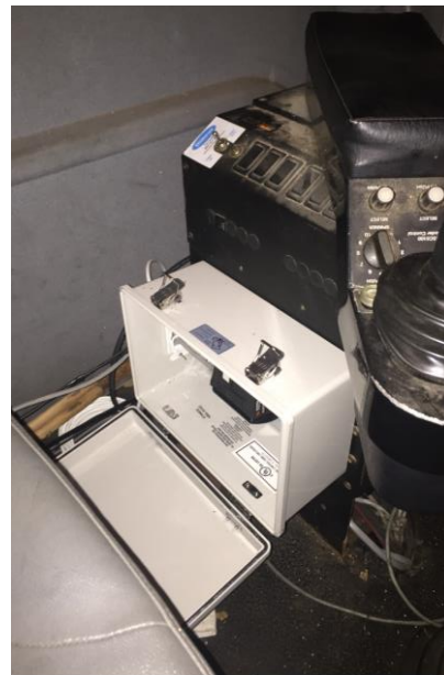
(b) Enclosure to Protect Modem
