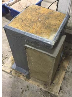
Fig. 35. The first casting of concrete in a water tank.
